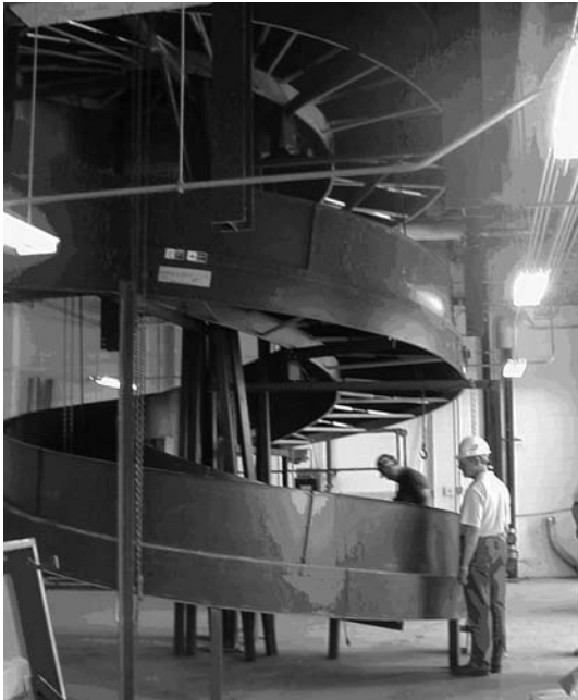
Baggage transfer system at the rail station at Newark Airport, which allows bags to be carried by truck to the terminal, is one of many solutions presented in ACRP Report 4, on ground access from public transportation to airports.
