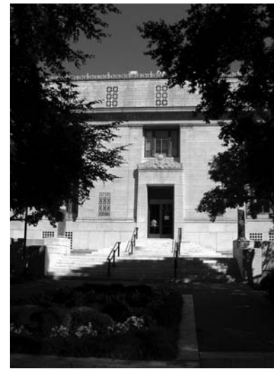
The National Academy of Sciences building on Constitution Avenue is scheduled to undergo a two-year renovation starting in spring 2009. The building is known for its architectural ornaments and bas-reliefs.
