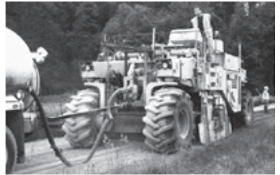
Water is injected during a mixing operation as part of the construction process for full-depth reclamation of failed pavements, described in Transportation Research Circular E-C135, Maintenance Management 2009 .
