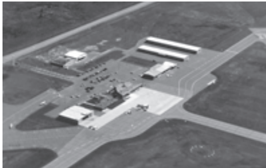
ACRP Report 16, Guidebook for Managing Small Airports , provides direction to managers of small airports. (Photo: Chisholm-Hibbing Airport Authority)
