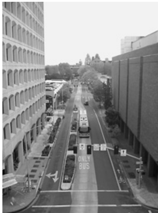
A bidirectional bus-only lane on a bus rapid transit line in Eugene-Springfield, Oregon, from TCRP Synthesis 83, Bus and Rail Transit Preferential Treatments in Mixed Traffic .
