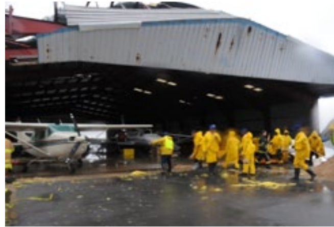
Firefighters and city employees work to contain oil and fuel spilled at the North Little Rock Airport in Arkansas after a 2008 tornado damaged aircraft and buildings. Upcoming HMCRP reports present practical approaches to emergency response preparedness, release containment, and more. (Photo: Charles S. Powell, FEMA)
