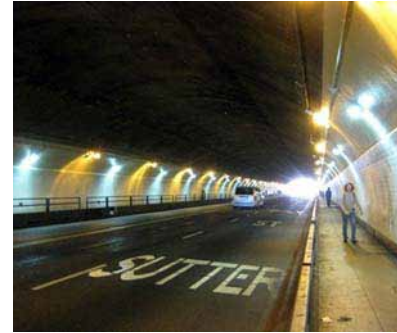
Design guidance for fire management in tunnels—including combined-use tunnels such as this one in San Francisco, California—is explored in NCHRP Synthesis 415.
