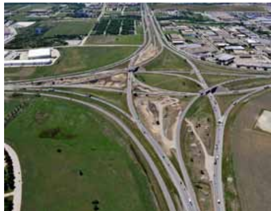
Completion of the North Tarrant Express Lanes in Texas is scheduled for 2015. This and other transportation projects fostered under public-private partnerships were examined in a special issue of TR News developed through the Project Delivery Methods Committee. (Photo: North Tarrant Express)
