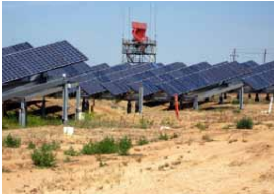
The solar photovoltaic panels at Meadows Field Airport in Bakersfield, California, are located approximately 250 ft from the runway. ACRP Synthesis 28 examines the safety impacts of energy technologies on aviation. (Photo: Harris Miller Miller & Hanson Inc.)
