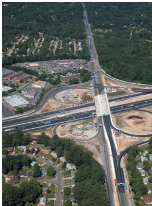
The SHRP 2–developed Selection Assistant for Utility Locating Technologies tool provided a cost-saving preliminary estimate and comparison of alternatives for a proposed alignment of Route 620 in Fairfax County, Virginia. (Photo: Trevor Wrayton, Virginia DOT)
