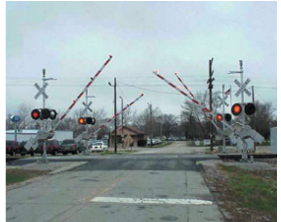
A four-quadrant gate grade crossing treatment in Gardner, Illinois. NCFRP Report 16 provides guidance for protecting and preserving freight infrastructure and routes. (Photo: U.S. DOT)
