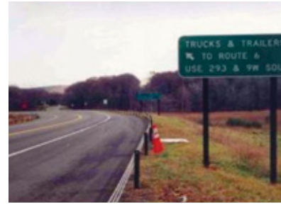
An example of improper roadway signs and geometrics. The second edition of NCHRP Report 600, Human Factors Guidelines for Road Systems , presents information on human factors for highway designers and traffic engineers.
