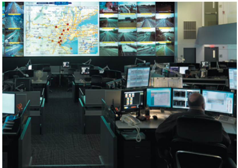
The New Jersey Turnpike Authority's high-tech Traffic Management Center. NCHRP Report 693 offers practical guidance on training skilled staff for traffic operations and management. (Photo: New Jersey Turnpike Authority)
