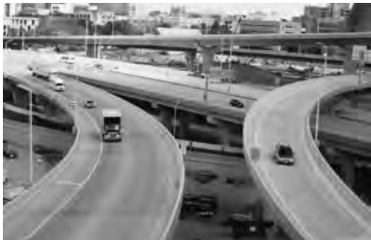
High-performance concrete, used for the deck and substructure of Lake Champlain Bridge in New York State, is the focus of NCHRP Synthesis 441. (Photo: New York State Department of Transportation)
