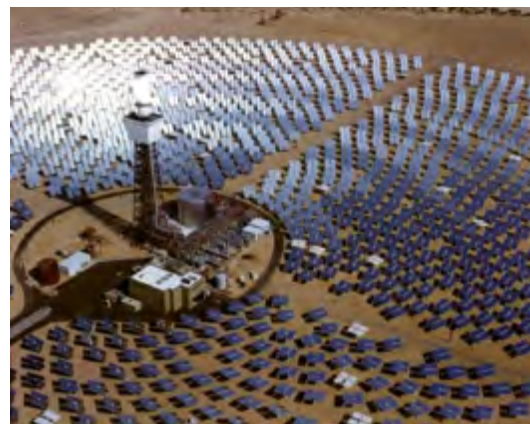
A solar-powered central receiver system in Daguerre, California. Renewable energy for highway maintenance facilities is explored in NCHRP Report 751. (Photo: Sandia National Laboratories)
