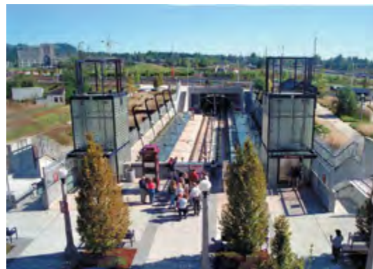
The Sunset Transit Center in Portland, Oregon. The Transit Cooperative Research Program published the third edition of the highly valued Transit Capacity and Quality of Service Manual in 2013.
