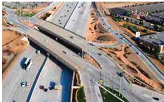
The diverging diamond interchange project at Pioneer Crossing in Utah is presented in NCHRP Synthesis 455, Alternative Technical Concepts for Contract Delivery Methods , as an innovative solution generated by alternative concepts in a design-build project. (Photo: S. Haines)
