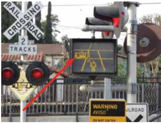
A pictogram in a blank-out sign in Los Angeles shows a side view of approaching trains, from TCRP Report 175, Guidebook on Pedestrian Crossings of Public Transit Rail Services . (Photo: Fitzpatrick)
