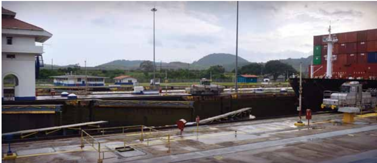
Miraflores Locks on the Panama Canal. (Photo: Amanda Richards)
