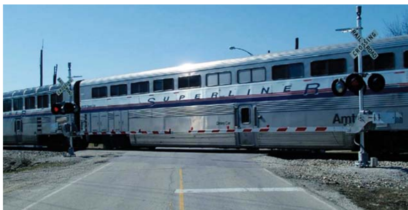
Four-quadrant gate installation on an intercity passenger rail line, an example of grade crossing design in National Cooperative Rail Research Program Report 6, Guidebook for Intercity Passenger Rail Service and Development .
