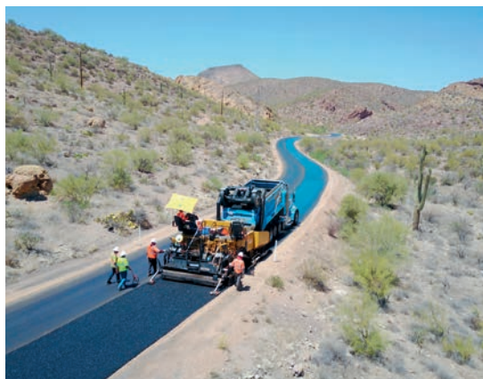
The Arizona Department of Transportation conducts pavement preservation activities along the Apache Trail. Pavement preservation treatments are the subject of NCHRP Research Report 858. (Photo: Arizona DOT)
