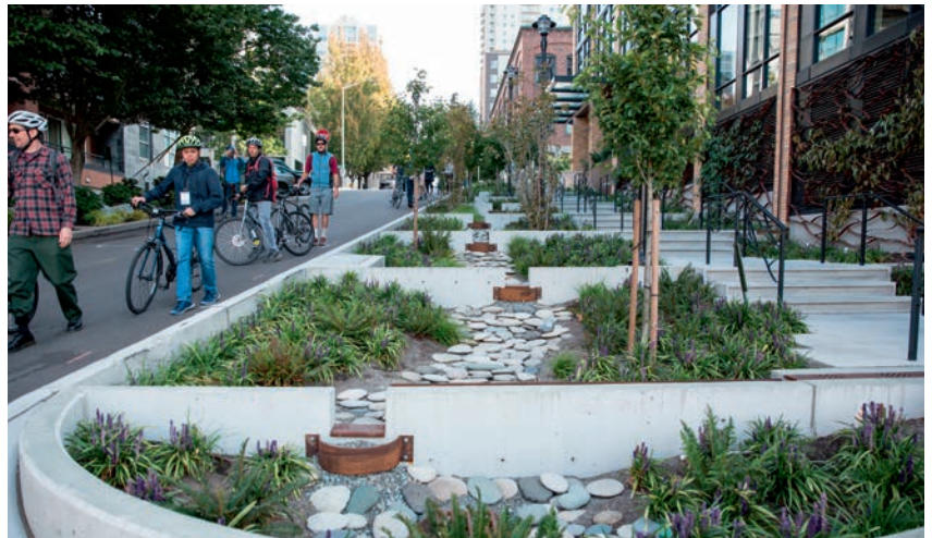
Bioswales remove pollutants and debris from runoff water. A webinar presented by the Stormwater Committee examined a U.S. Environmental Protection Agency web portal for stormwater infrastructure financing options. (Photo: NACTO)
