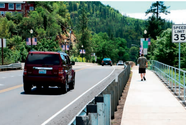
New communications efforts include using social media to highlight research and innovation by state departments of transportation; for example, the impact of bike lane and sidewalk projects in Shady Cove, Oregon. (Photo: Oregon Department of Transportation)
