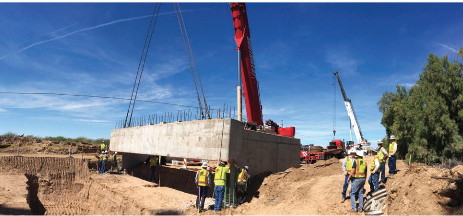
Arizona’s DOT used accelerated bridge construction, one of the innovative bridge construction techniques examined in a TRB consensus study report, in its Sacramento Wash project. (Photo: Arizona DOT)
