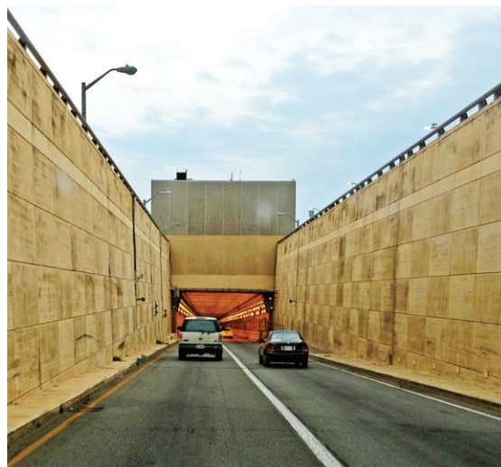
A webinar conducted by TRB along with the Federal Highway Administration and the American Association of State Highway and Transportation Officials examined tunnel management practices, including the Hampton Roads Bridge–Tunnel expansion. (Photo: David Broad, Wikimedia)
