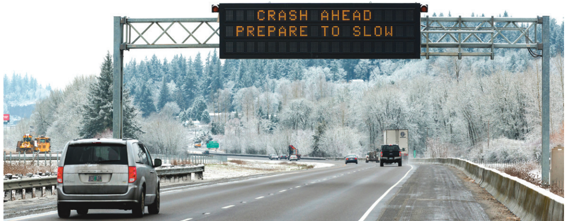
Variable message signs provide information like traffic and weather updates, roadwork warnings, and crash notifications. A BTSCRP project is developing a guide for using these signs, including how and when to post, barriers to implementations, and impacts and effectiveness. (Photo: Oregon DOT)
