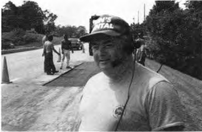
FIGURE 2 Maintenance workers were impressed with the capability of voice recognition system for data collection (photograph taken in Maryland).
