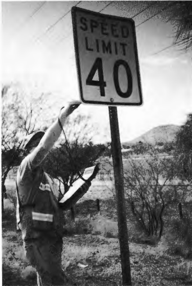
FIGURE 3 Barcoding and pen-based systems are ideal for sign maintenance and inventory management (photograph taken in Arizona).
