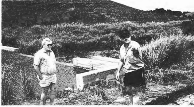
FIGURE 13 Vetiver stabilizing concrete-earth interface and protecting sides of downstream drainage way, Natal, South Africa (photograph courtesy J. C. Greenfield).
