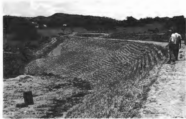
FIGURE 11 Newly planted vetiver on downstream slope of earth dam in Zimbabwe. Vetiver rows have actually been planted too close together and are therefore more costly than necessary. Lines should have been planted about 1 m apart (photograph courtesy J. C. Greenfield).
