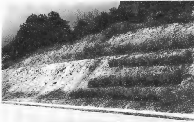
FIGURE 5 Malaysia test planting using containerized raised plants on highway cut 8 months after planting vetiver hedges. Note unprotected area continues to erode; where protected, other grass species are now able to become established. Alternative to vetiver is to continue applying costly and often ineffective hydroseeding techniques (photograph courtesy P. K. Yoon).
