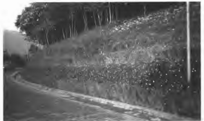
FIGURE 8 Two rows of vetiver hedges interplanted with leguminous cover effectively protect road cut in Thailand. Note sediment-free drain (photograph by R. G. Grimshaw).
