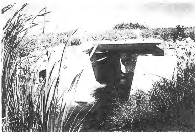
FIGURE 1 V-notch weir.
