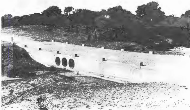
FIGURE 2 Concrete slab with three openings.
