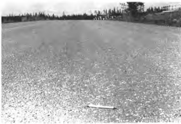
FIGURE 7 Surface performing well after 14 months of treatment.
