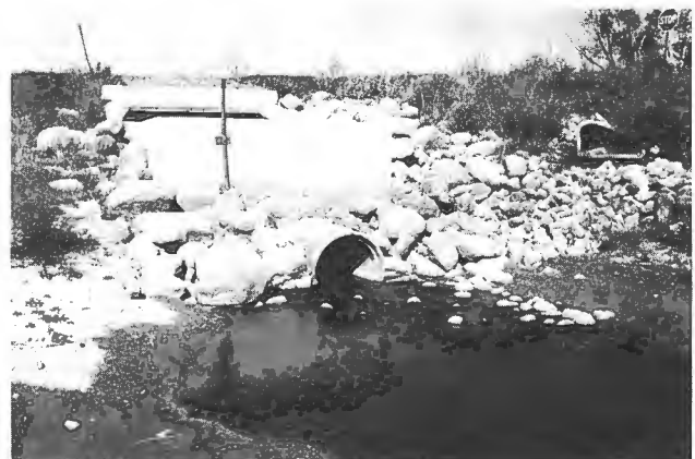
FIGURE 2 Cottonwood River box inlet structure.
