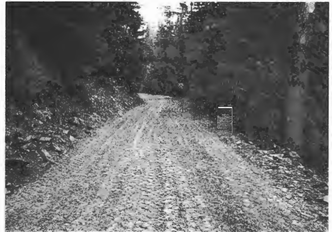
FIGURE 9 Leigh Lake Road: typical section after processing with Roto Trimmer.
