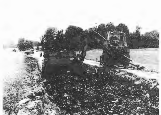
FIGURE 3 Leveling tire chips with backhoe.
