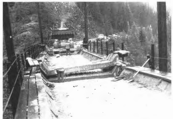
FIGURE 6 Removal of first ballast box from Dick Creek trestle.
