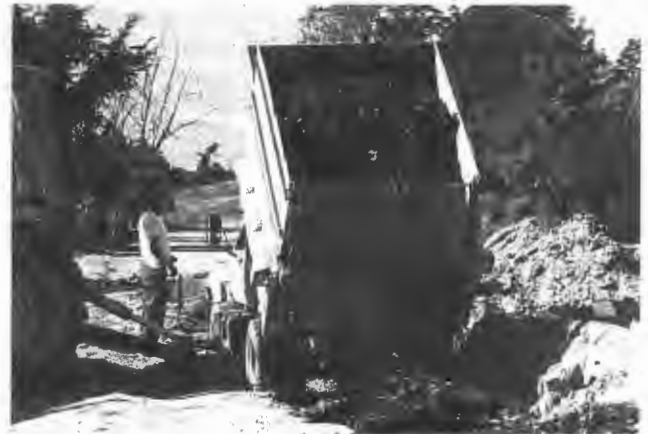
FIGURE 7 Backfilling excavation with 16-yd 3 load of tire chips.
