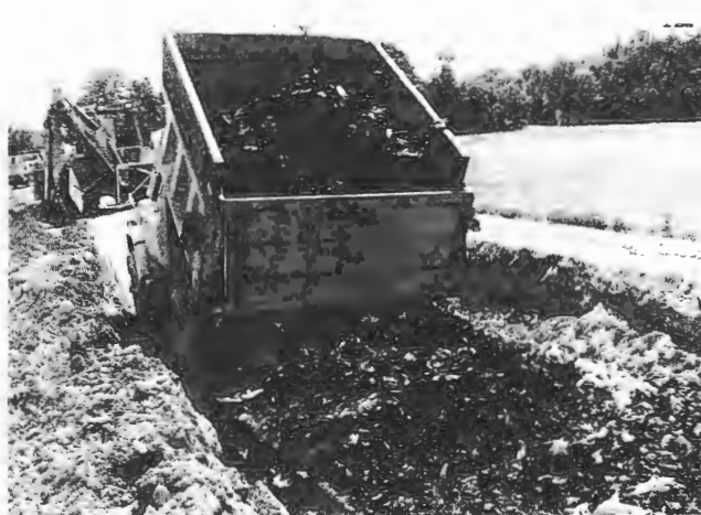
FIGURE 2 Dumping tire chips, August 1, 1990.
