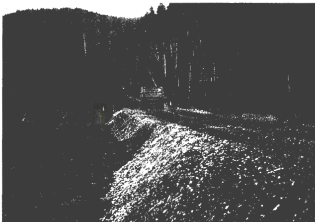
FIGURE 1 Unsurfaced woodwaste road.
