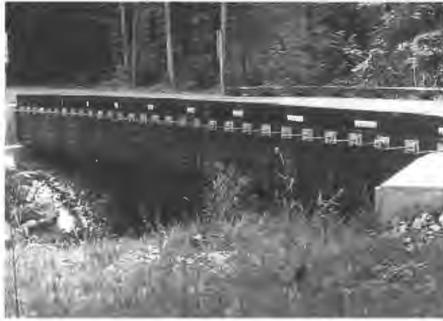
FIGURE 5 Camp Arrowhead bridge.
