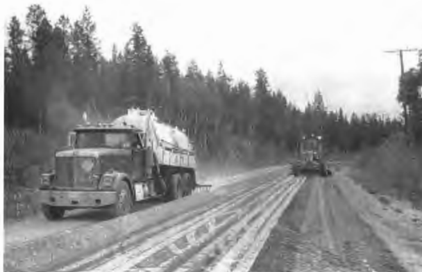
FIGURE 2 Motor grader spreads aggregate before each spray coat.
