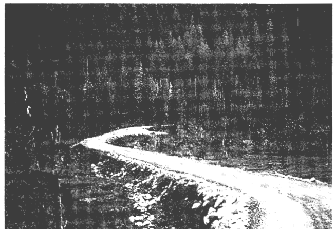
FIGURE 3 Finished woodwaste road.
