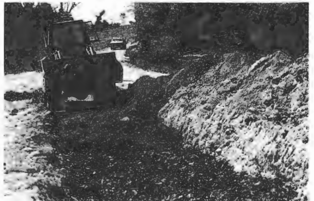
FIGURE 9 Backfilling trench with original gravel.
