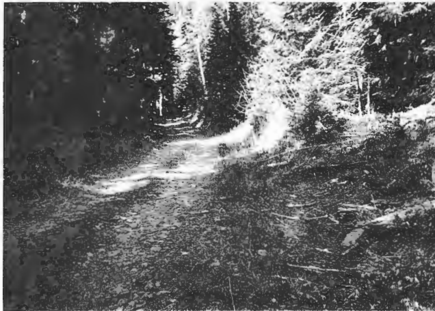
FIGURE 8 Leigh Lake Road: typical section before processing with Roto Trimmer.
