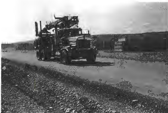
FIGURE 5 Treated road surface.
