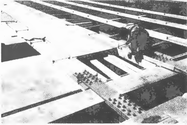
FIGURE 4 Bridge deck formwork.
