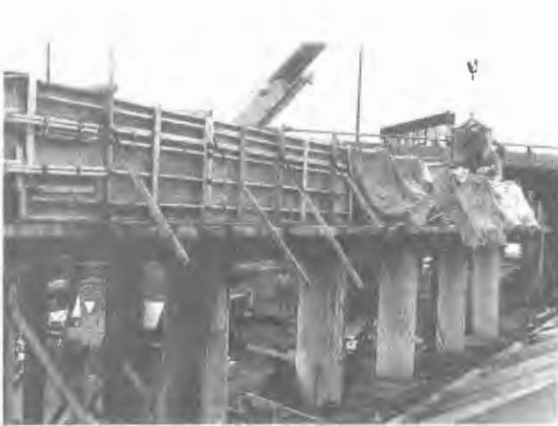
FIGURE 5 Job-built formwork.
