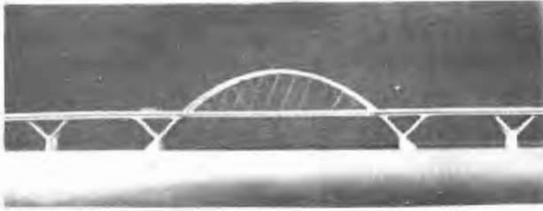
FIGURE 5 Arch rib and delta elevations.
