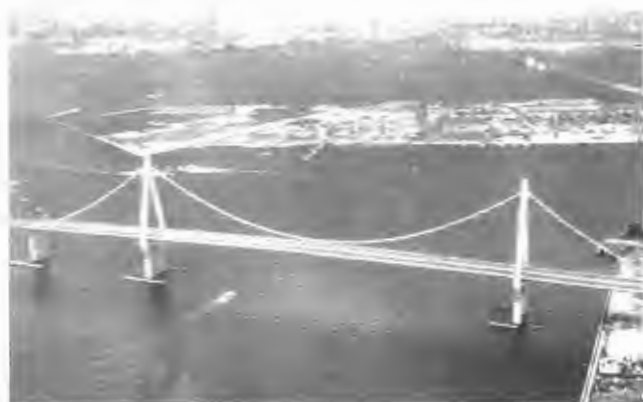
FIGURE 18 Hokko Bridge, Japan.
