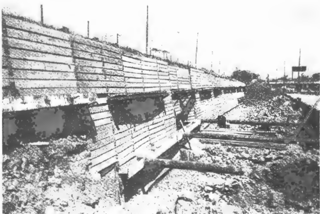
FIGURE 6 Soldier piles retained with soil anchors.
