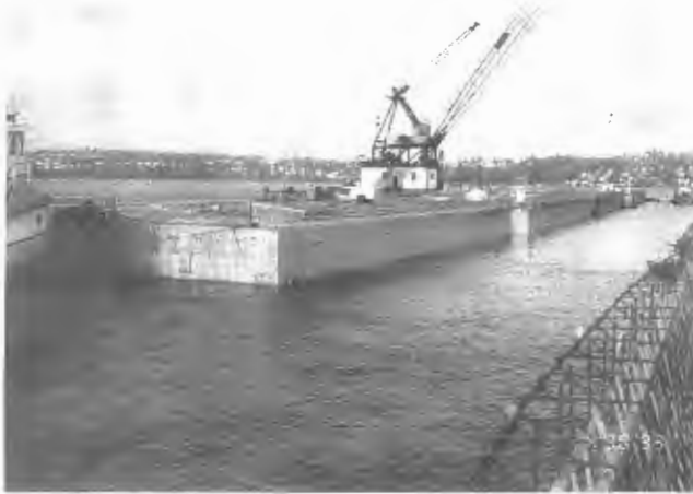
FIGURE 6 Pair of pontoons being maneuvered into position.
