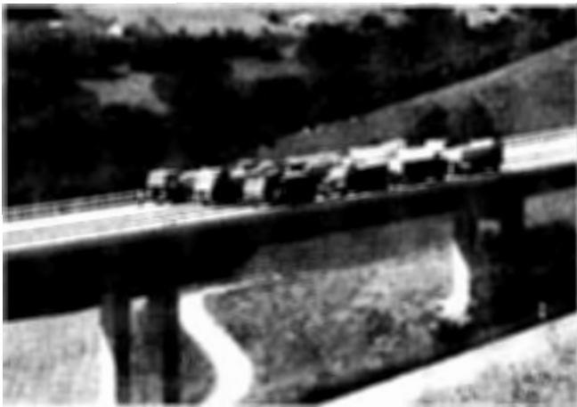
FIGURE 1 Load test of Daidard bridge in French-speaking Switzerland.
