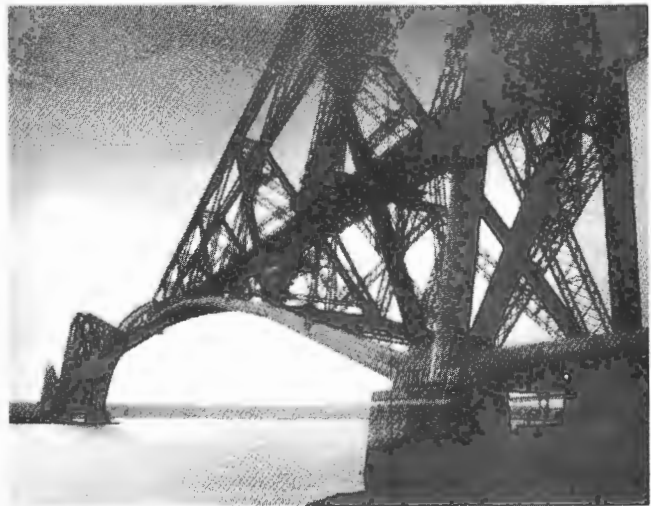
FIGURE 13 Firth of Forth Rail Bridge showing varying angles of the diagonals.
