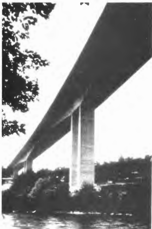
FIGURE 9 Felsenau Bridge, Christian Menn, Bern, Switzerland, 1974.
