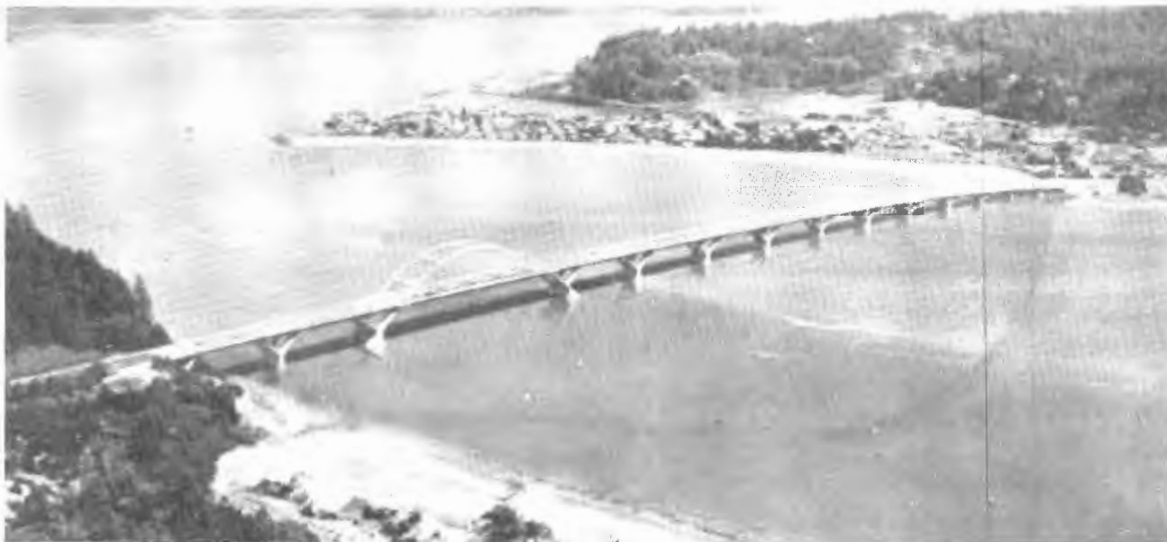
FIGURE 6 New Alsea Bay Bridge.
