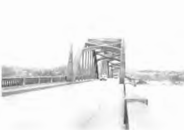
FIGURE 3 First Alsea Bay Bridge showing roadway at through concrete arch spans. Concrete spires provided emphasis to arch span.
