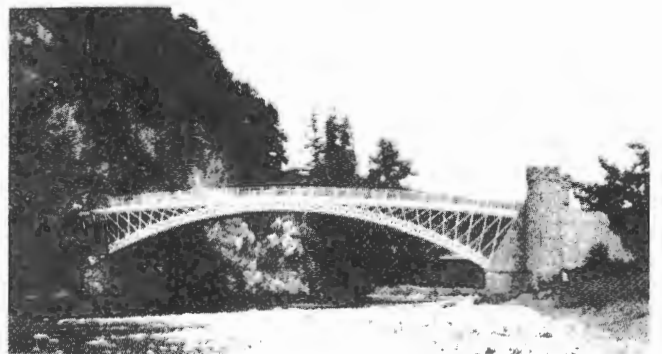
FIGURE 2 Craiglechie Bridge over Spey River, Thomas Telford, Elgin, Scotland, 1814.
