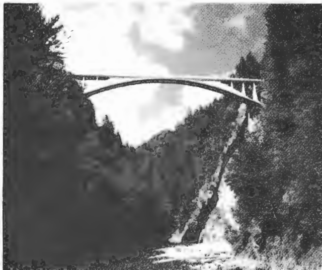
FIGURE 8 Salginatobel Bridge, Robert Maillart, Switzerland, 1930.
