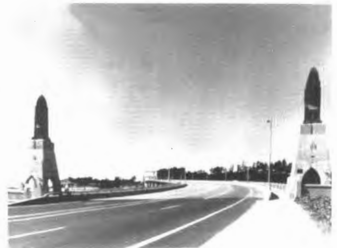
FIGURE 8 Bridgehead at south abutment.
