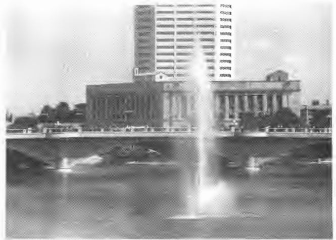
FIGURE 16 Overall view of bridge.
