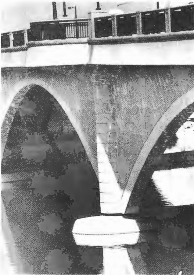
FIGURE 11 Pier pilaster, trumpet, and balcony.
