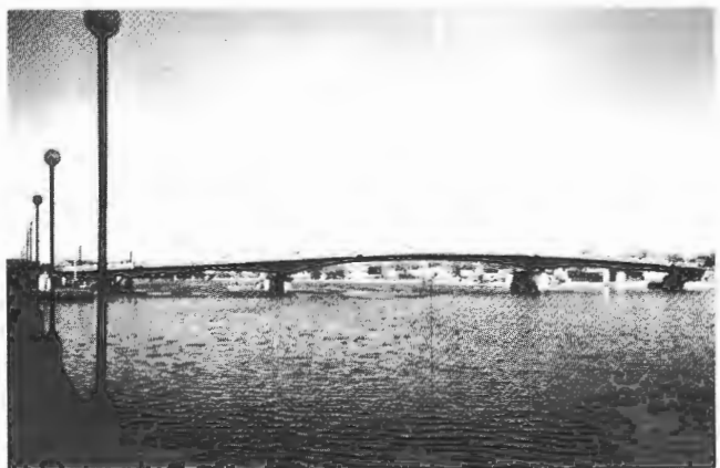
FIGURE 20 Dundas Street over Trent River, Trenton, Ontario.
