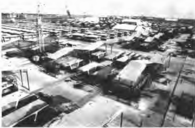
FIGURE 2 Aerial view of casting yard.
