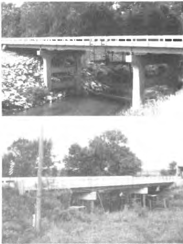
FIGURE 3 Photographs of strengthened bridges: top , Bridge 1; bottom , Bridge 2.
