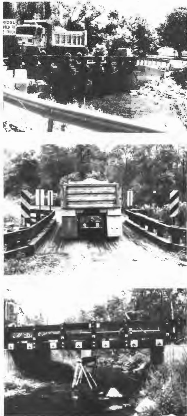
FIGURE 1 Field test bridges: top , Trout Road; middle , Little Salmon; bottom , Lampeter.
