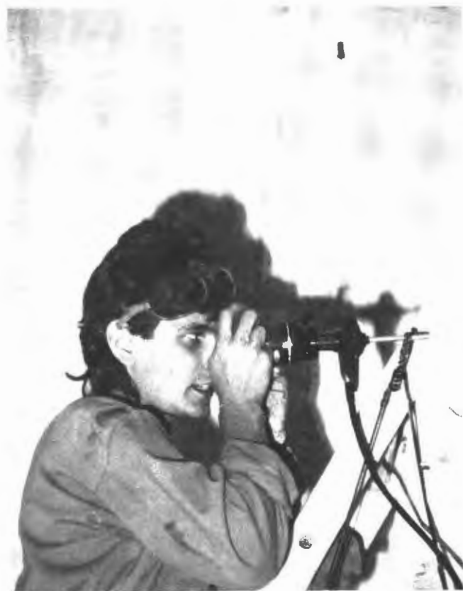
FIGURE 1 Control with an endoscope of a prestressing cable embedded into a beam. Photographic images of cables can also be obtained by this technique.
