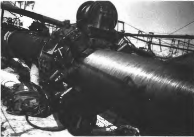
FIGURE 2 Wire wrapping main cable areas.
