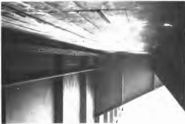
FIGURE 2 View of girder-cantilever bracket.
