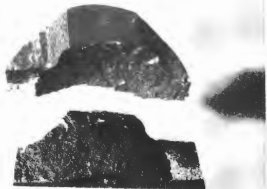
FIGURE 10 Exposed crack surface of Core 25 showing path of crack into flange plate.
