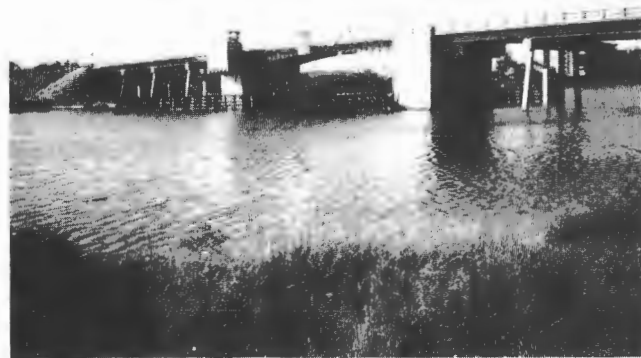
FIGURE 4 Bascule bridge over Intracoastal Waterway, Indian Rocks, District 7, FDOT.
