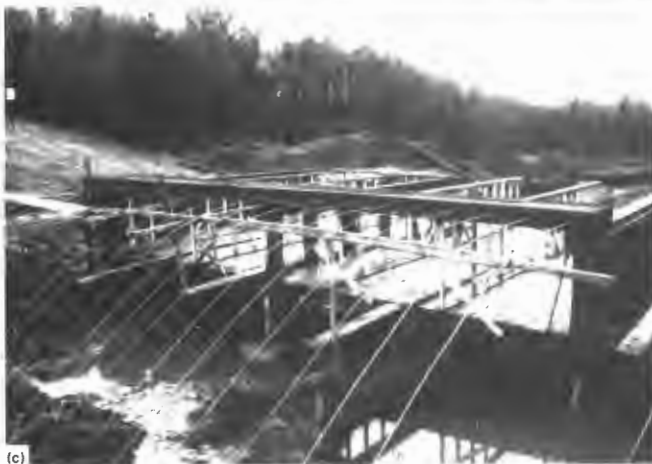
FIGURE 2 Construction sequence for Cooper Creek bridge: (a) placement of laminations along south bridge edge; (b) insertion of stressing bars; (c) support of bar overhang by wood frame; (d) sequential addition of laminations; (e, f) completed bridge width ready for bar tensioning.
