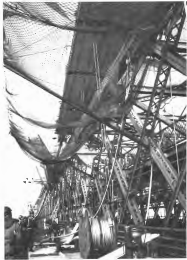
FIGURE 5 Paint chip containment for suspender removal operations: left , shrink wrap being applied to suspender from movable scaffolding; right , plastic-wrapped suspender being lowered to roadway level.
