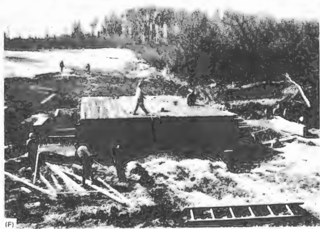
FIGURE 2 Construction sequence for Cooper Creek bridge: (a) placement of laminations along south bridge edge; (b) insertion of stressing bars; (c) support of bar overhang by wood frame; (d) sequential addition of laminations; (e, f) completed bridge width ready for bar tensioning.
