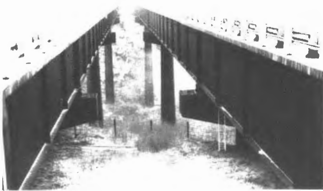
FIGURE 1 View looking west between twin bridge structures.
