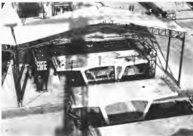
FIGURE 3 Typical D2 casting machine.
