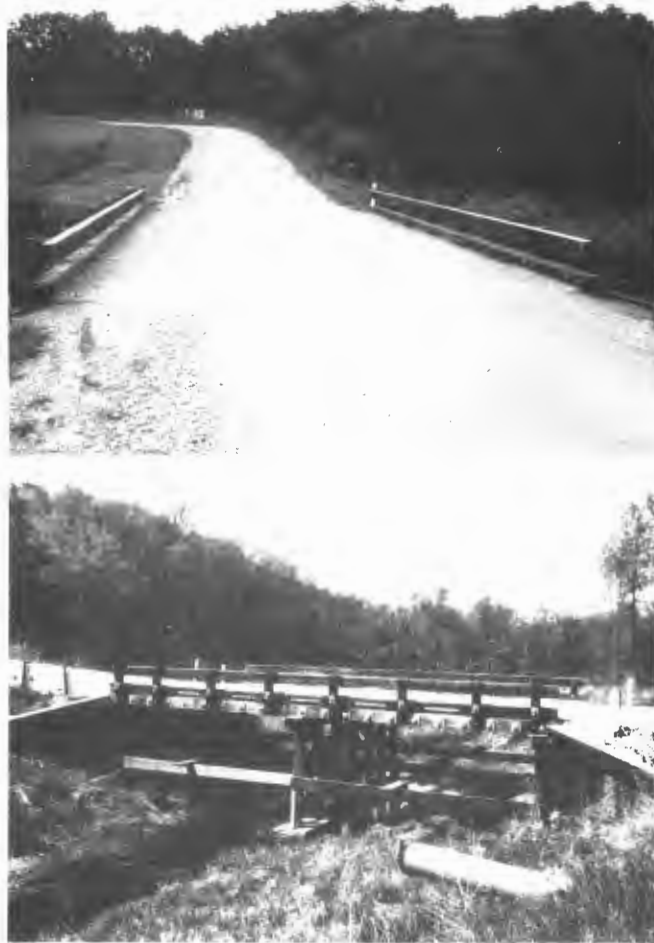
FIGURE 3 Completed Cooper Creek bridge (two views).
