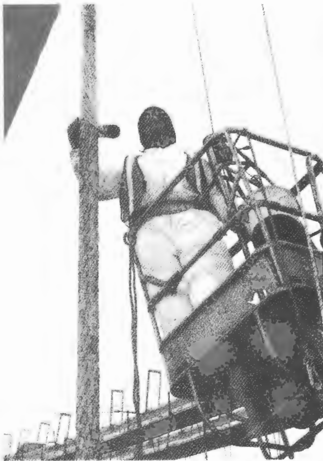
FIGURE 5 Paint chip containment for suspender removal operations: left , shrink wrap being applied to suspender from movable scaffolding; right , plastic-wrapped suspender being lowered to roadway level.
