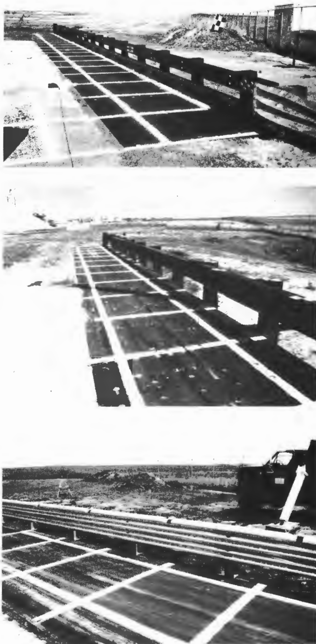
FIGURE 2 Bridge railings successfully crash tested to AASHTO PL-1 (photographs taken before testing).
