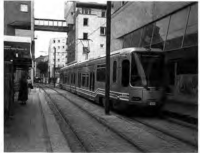
FIGURE 9 All passenger entry doors in a partial low-floor car are the low-platform level, typically about 330 mm (13.5 in.). This example is operating in Paris.
