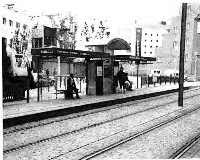
FIGURE 8 Low-level platforms are not as intrusive on a city street as are high-level platforms. This stop is in Paris.
