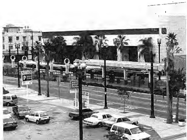
FIGURE 7 High-level platforms provide level entry to high-floor cars. Integrating such platforms into the city scene can be done attractively, as in Long Beach, California.
