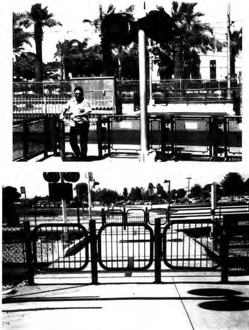
FIGURE 8 Pedestrian swing gate examples: top , Los Angeles LRT system; bottom , San Jose LRT system.
