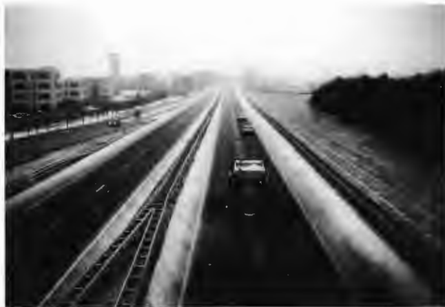
FIGURE 4 Prewetted salt is spread on surface before ice layer forms.
