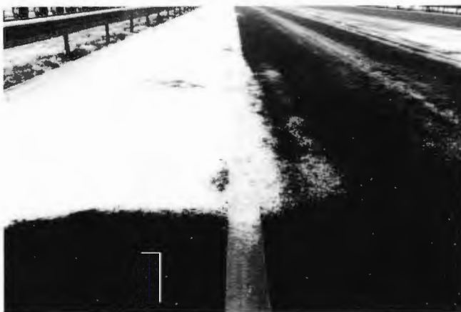
FIGURE 8 Hard shoulder of porous asphalt next to dense asphalt concrete road surface. Shoulder is fully covered with snow because without traffic action, salt remains in voids rather than transferring to surface.
