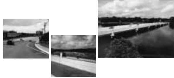
FIGURE 3 Navesink River Bridge, Route 35.
