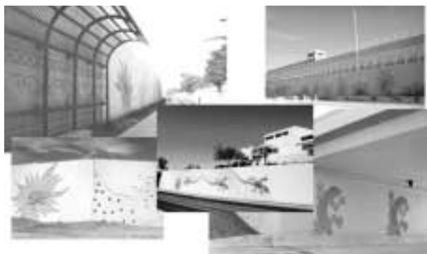
FIGURE 2 Pima Freeway, Scottsdale, Arizona.
