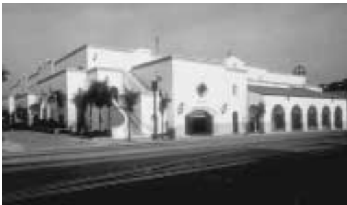
FIGURE 5 Parking garage, Santa Barbara, California.
