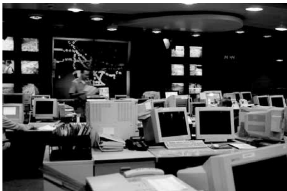
FIGURE 5 Caltrans District 7 Traffic Management Center.
