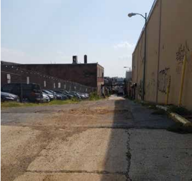
Impervious surfaces, such as this sloped alleyway in Washington, D.C., reduce opportunities for infiltration, thereby increasing the speed of runoff and the likelihood of flooding while reducing water quality. (ULI Washington)
