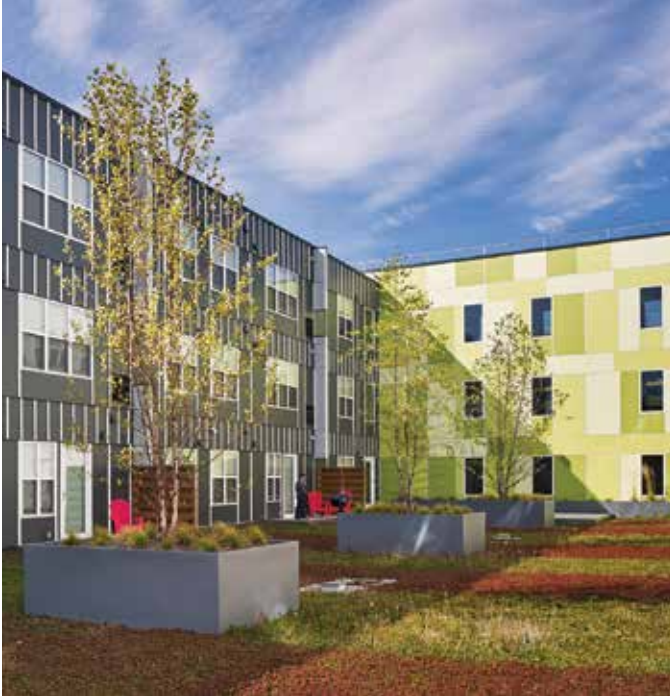
Paseo Verde, a 120-unit mixed-income development in North Philadelphia, has a green roof over the first level that minimizes runoff and doubles as garden courtyards, an attractive amenity for residents. (Halkin Mason Photography)
