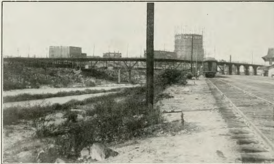
FIG. 47. FIRST STREET VIADUCT, ACROSS LOS ANGELES RIVER This is a steel structure with a wooden floor, built prior to 1890, now in a very bad state of repair, and it has been condemned by the City Engineering Department. The approaches carry the street over the Santa Fe and Salt Lake tracks.
