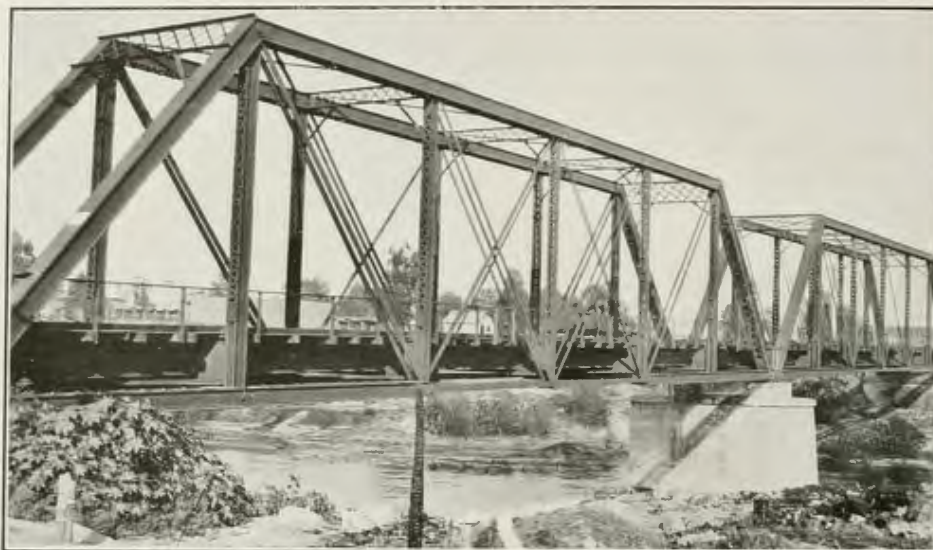
FIG. 61. SANTA FE BRIDGE ACROSS LOS ANGELES RIVER SOUTH OF BUTTE STREET
