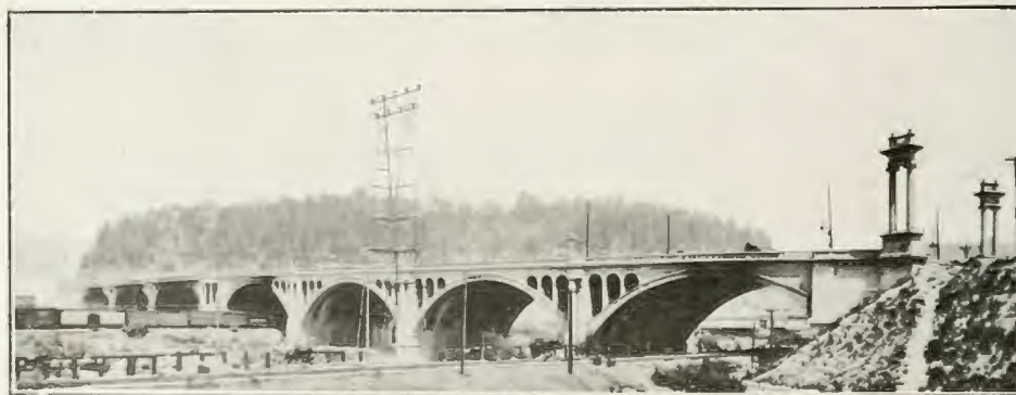
FIG. 31. NORTH BROADWAY BRIDGE
