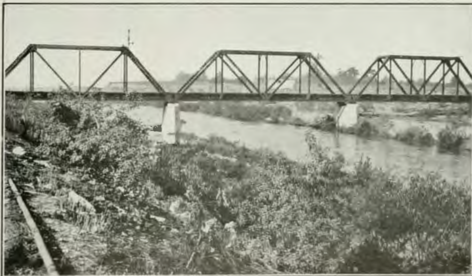
FIG. 60. SALT LAKE BRIDGE ACROSS LOS ANGELES RIVER AT BUTTE STREET
