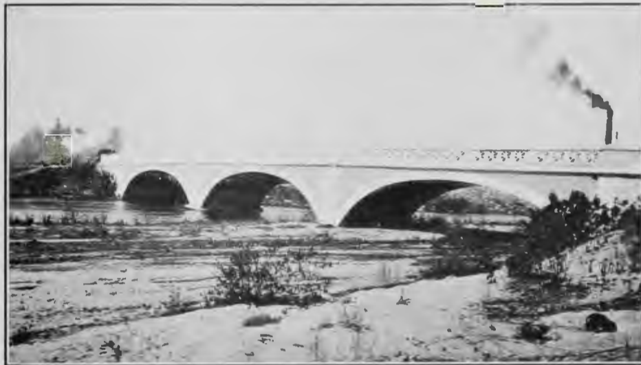
FIG. 62. TWENTY-SIXTH STREET BRIDGE OF THE LOS ANGELES RIVER
