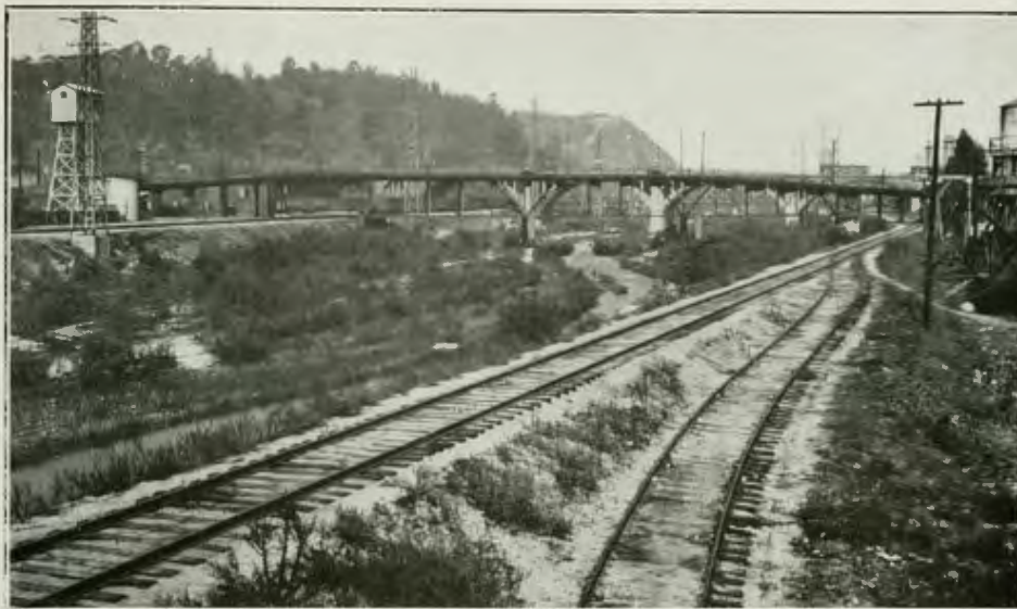
FIG. 32. NORTH SPRING STREET BRIDGE CROSSING THE TRACKS OF THE SANTA FE, THE LOS ANGELES RIVER AND THE TRACKS OF THE SALT LAKE
