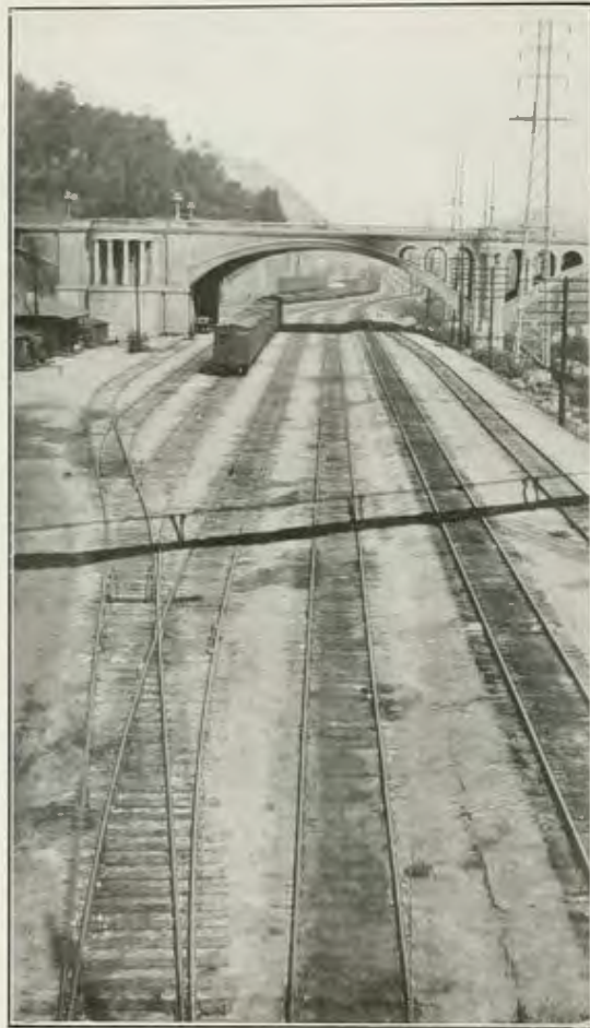
FIG. 35. LARGE PIER—NORTH BROADWAY BRIDGE
