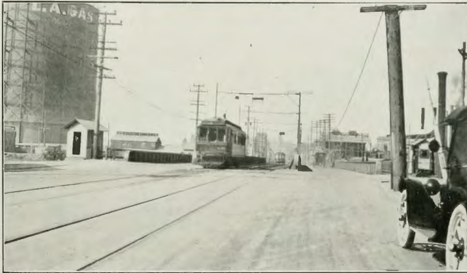
FIG. 43. VIEW LOOKING ALONG ALISO STREET BRIDGE ACROSS THE LOS ANGELES RIVER
