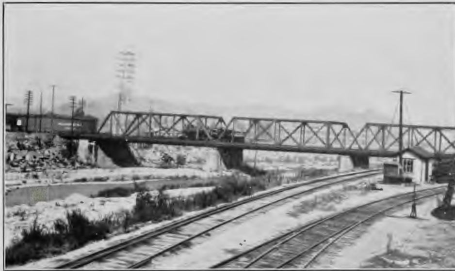
FIG. 38. SOUTHERN PACIFIC BRIDGE ACROSS THE LOS ANGELES RIVER AT ALHAMBRA AVENUE
