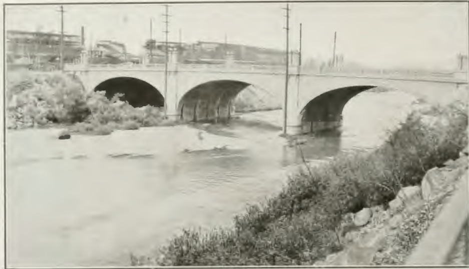
FIG. 54. SEVENTH STREET BRIDGE ACROSS LOS ANGELES RIVER
