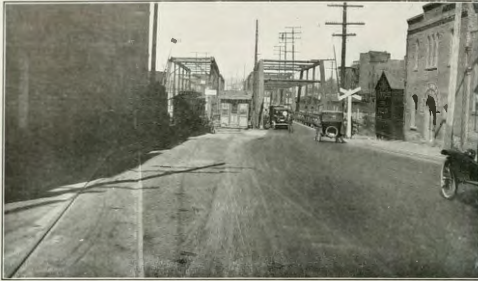
FIG. 40. ALONG MACY STREET BRIDGES
