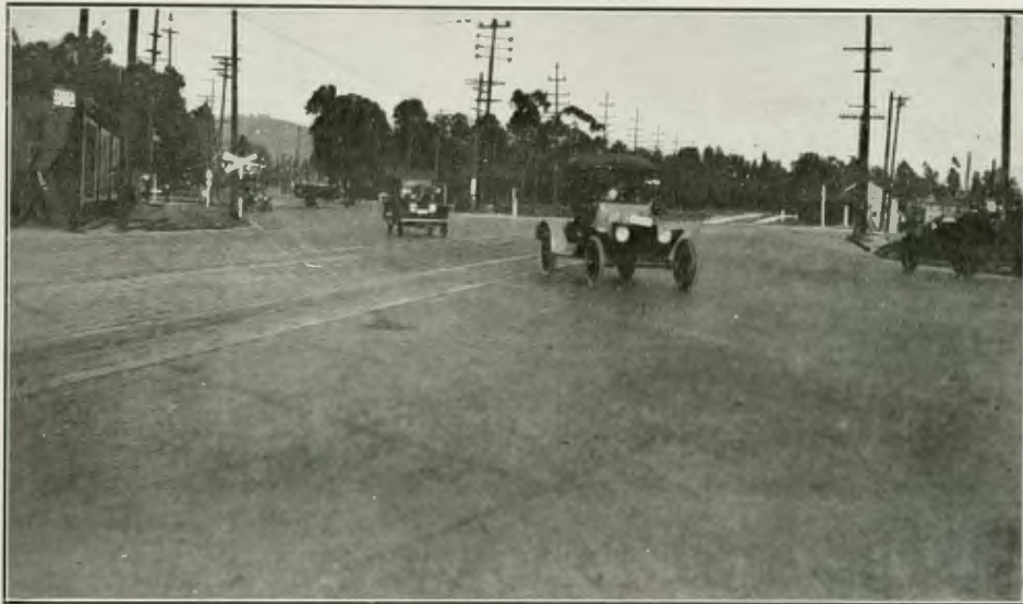
FIG. 71. INTERSECTION OF MISSION ROAD AT ALHAMBRA ROAD
