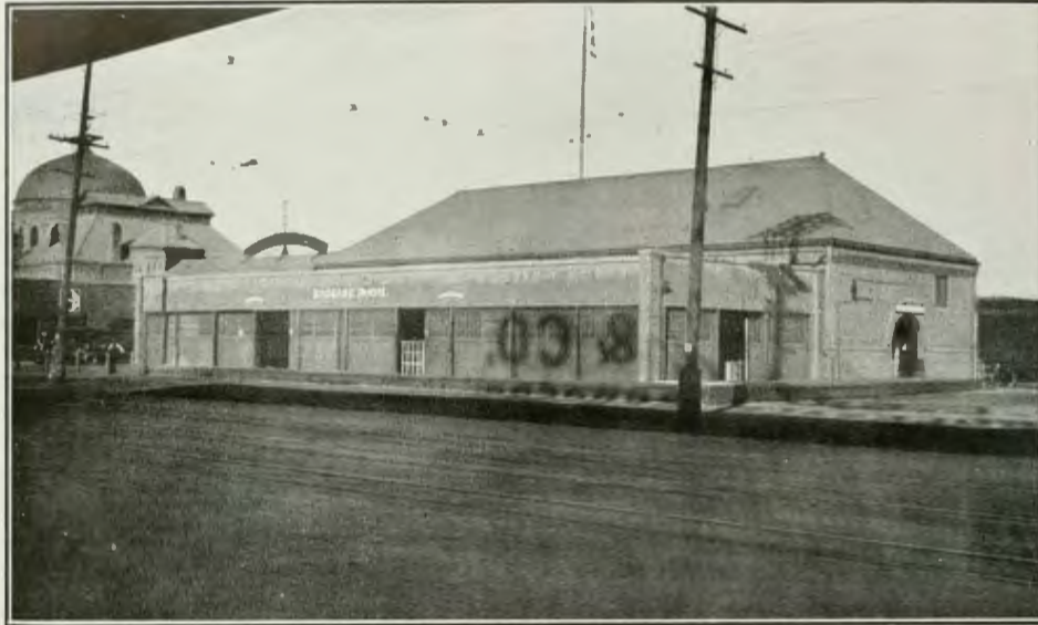
FIG. 94. BAGGAGE BUILDING AT SANTA FE DEPOT
