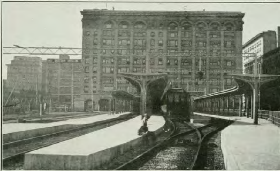
FIG. 87. PACIFIC ELECTRIC BUILDING—REAR VIEW
