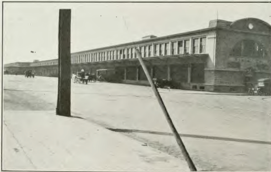
FIG. 150. SANTA FE INBOUND FREIGHT SHED
