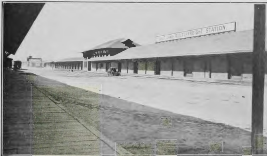
FIG. 154. SALT LAKE FREIGHT STATION
