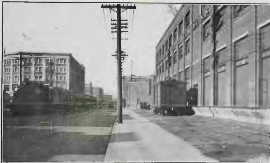
FIG. 170. SPUR TRACK PLACED BEHIND SIDEWALK
