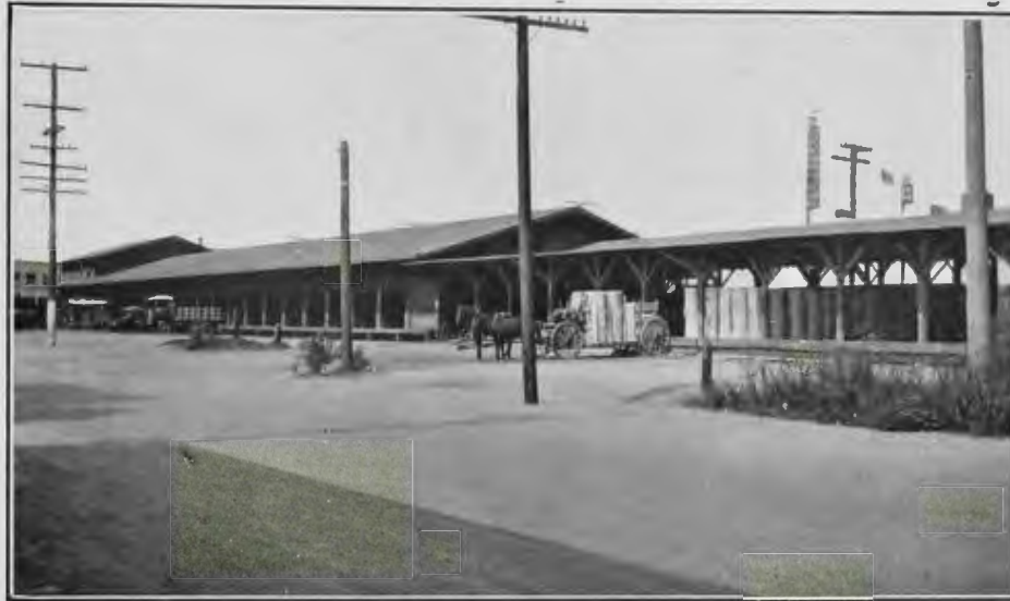
FIG. 156. PACIFIC ELECTRIC FREIGHT STATION
