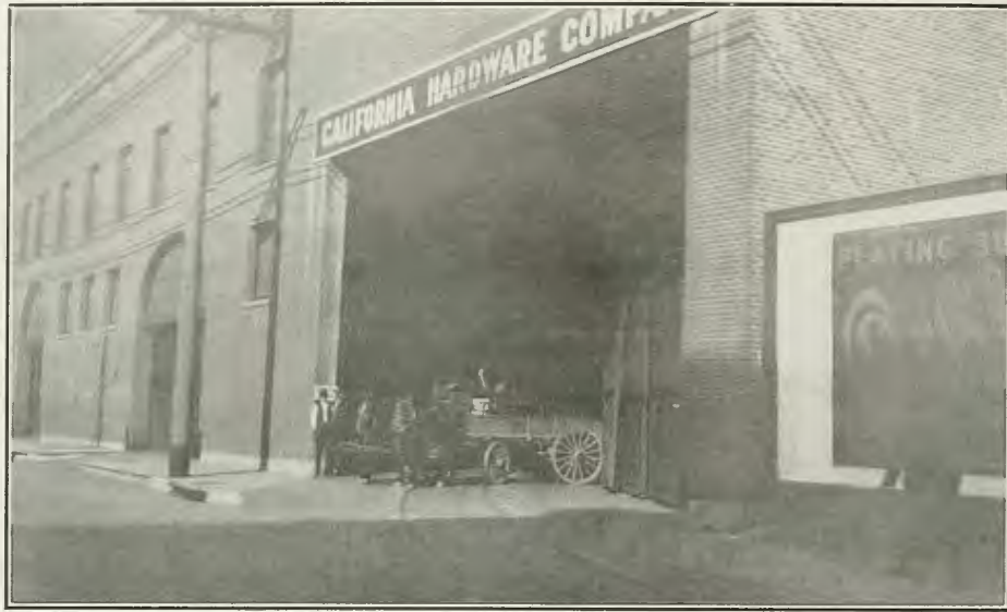
FIG. 171. WAREHOUSE WITH SPUR TRACK INSIDE
