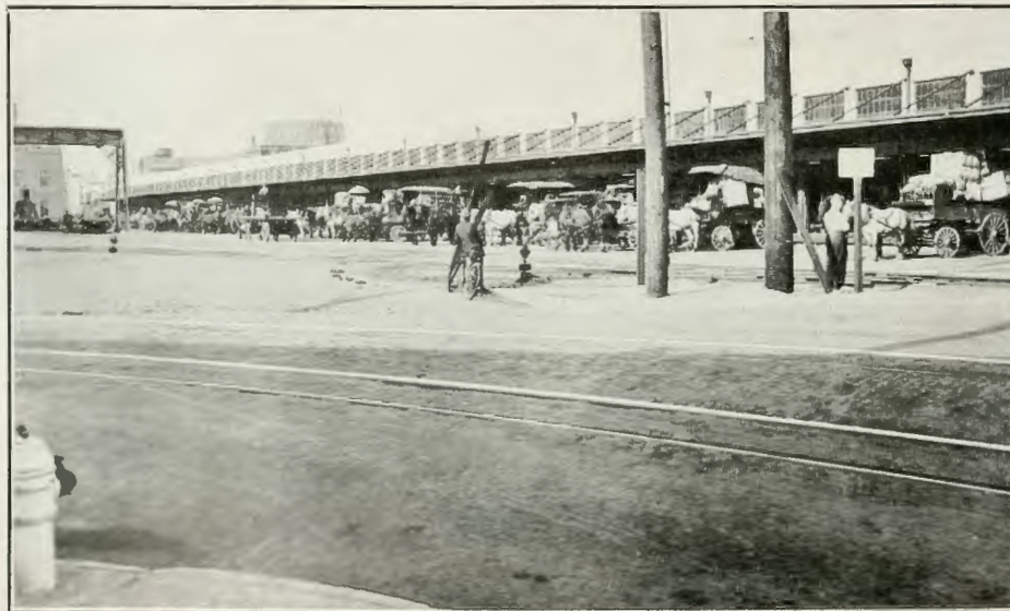
FIG. 153. SANTA FE OUTBOUND FREIGHT SHED
