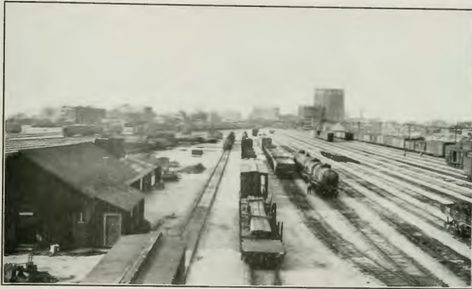
FIG. 141. SANTA FE YARDS NORTH OF FOURTH STREET BRIDGE
