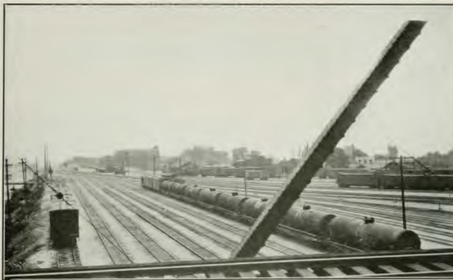
FIG. 142. SOUTHERN END OF SANTA FE FREIGHT YARD
