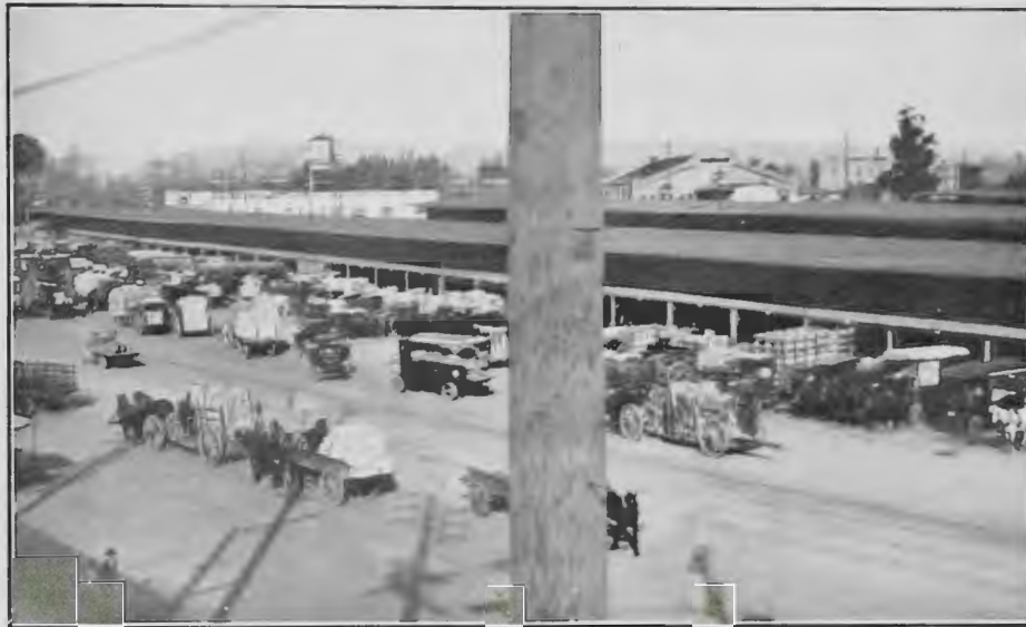
FIG. 148. SOUTHERN PACIFIC OUTBOUND FREIGHT SHED
