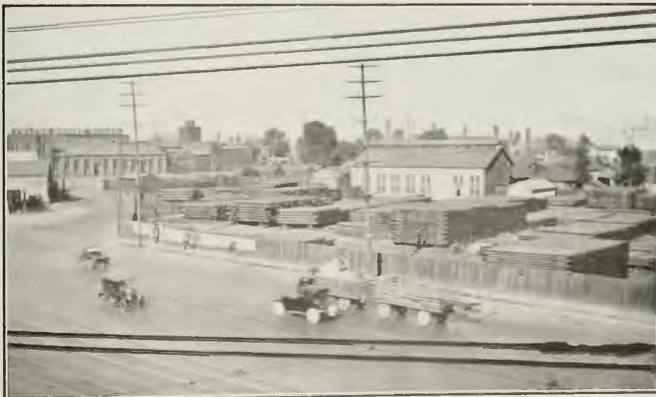
FIG. 197. LOOKING EAST ACROSS ALHAMBRA AVENUE AT ALAMEDA STREET This view shows the pipe yard of the Oil Well Supply Company with the plant of the Fulton Engine Works at the extreme left.
