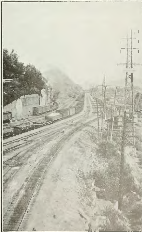
FIG. 140. SOUTHERN PACIFIC MIDWAY YARD. LYING ALONG THE WEST BANK OF THE LOS ANGELES RIVER AND NORTH OF BROADWAY.
