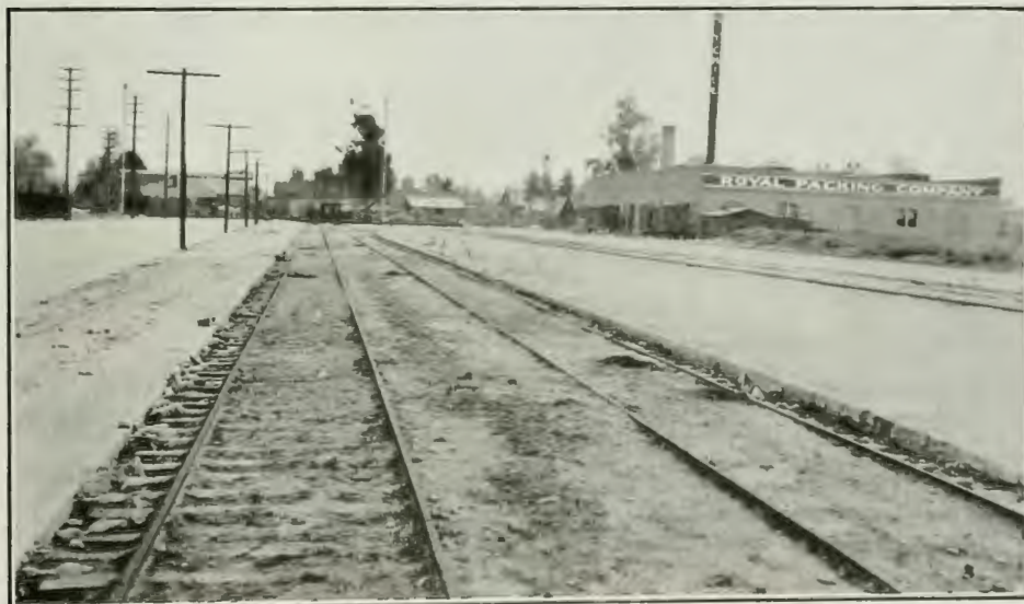
FIG. 162. SANTA FE TEAM YARD AT BAY AND LAWRENCE STREETS
