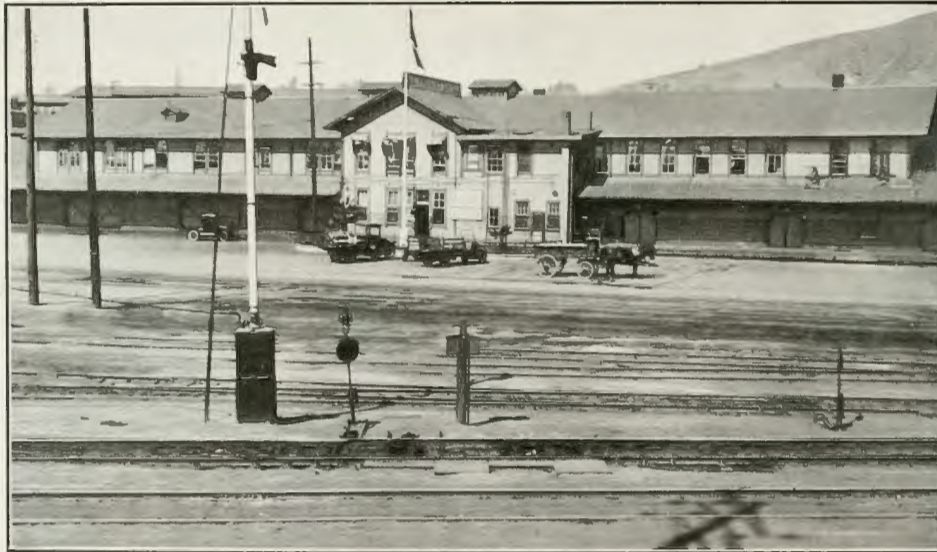
FIG. 147. SOUTHERN PACIFIC FREIGHT DEPOT
