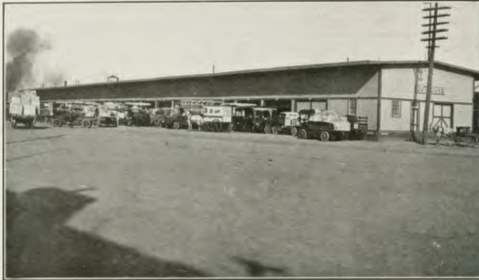
FIG. 149. ANOTHER VIEW OF SOUTHERN PACIFIC OUTBOUND FREIGHT SHEDS
