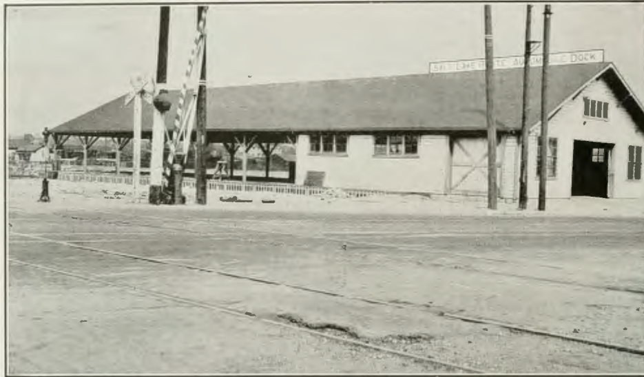
FIG. 155. SALT LAKE AUTOMOBILE FREIGHT STATION
