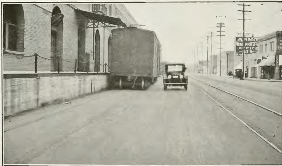
FIG. 172. SPUR TRACK ON ALAMEDA STREET NEAR FIRST STREET
