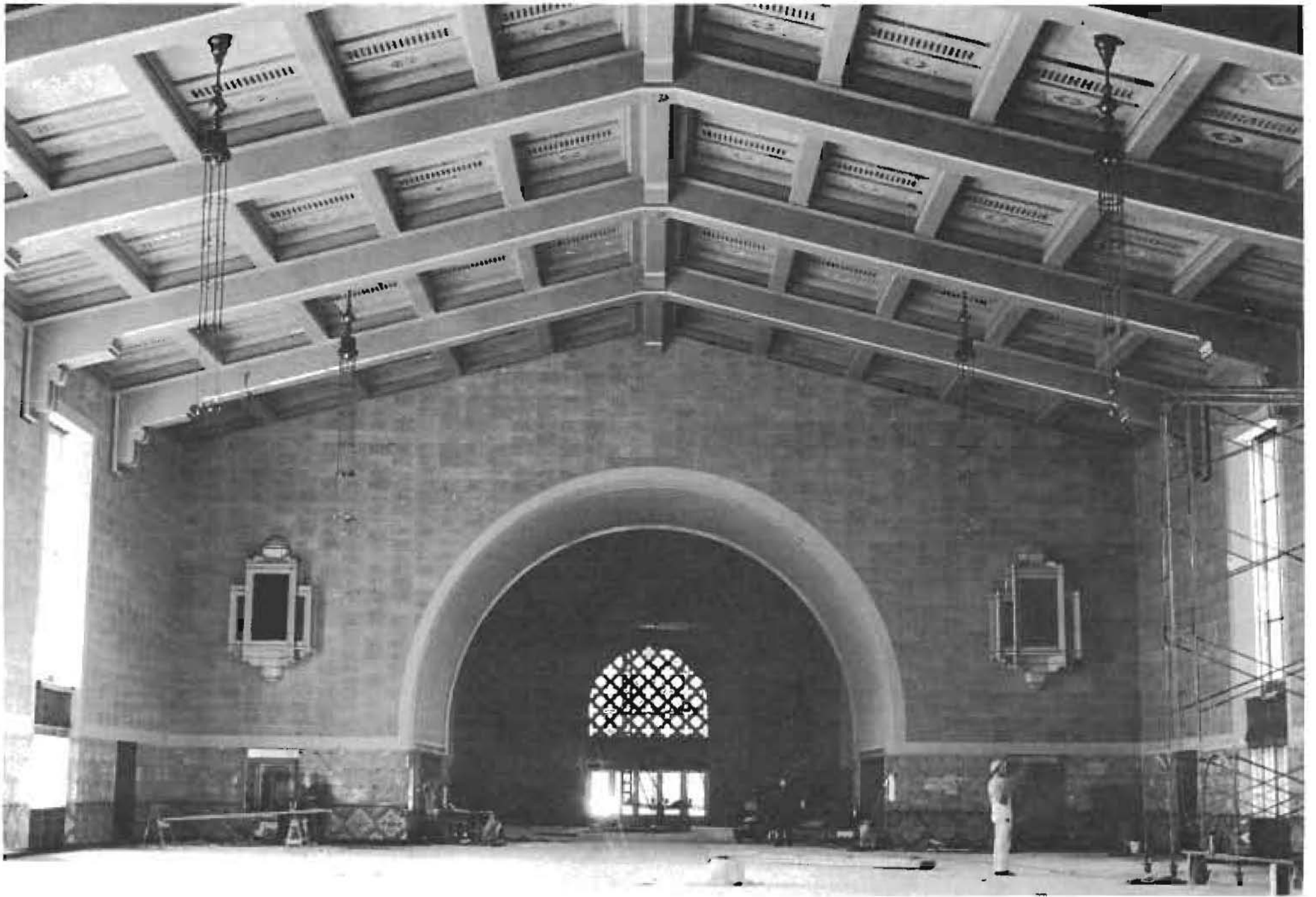
THE MAIN Waiting Room nears completion. Santa Fe Railway
