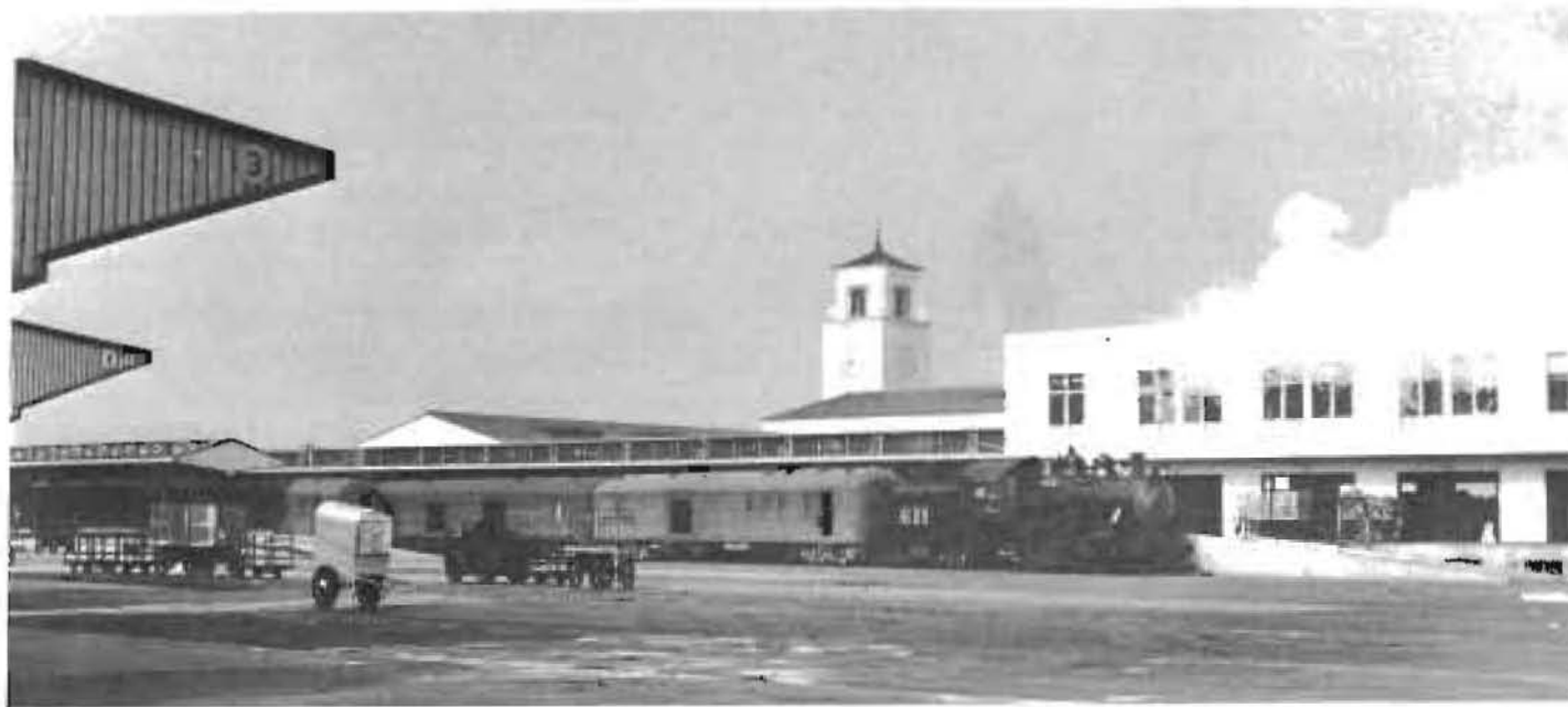
JUST BEHIND THE locomotive is the Utility Building, a two-and three-story structure which extends along the entire length of the platforms, acting as a bridge between them and the terminal building. In the '40s and '50s, this building handled all baggage, mail and express. Baggage carts moved up to train level from the street on a curving ramp (off the picture at right). Donald Duke
