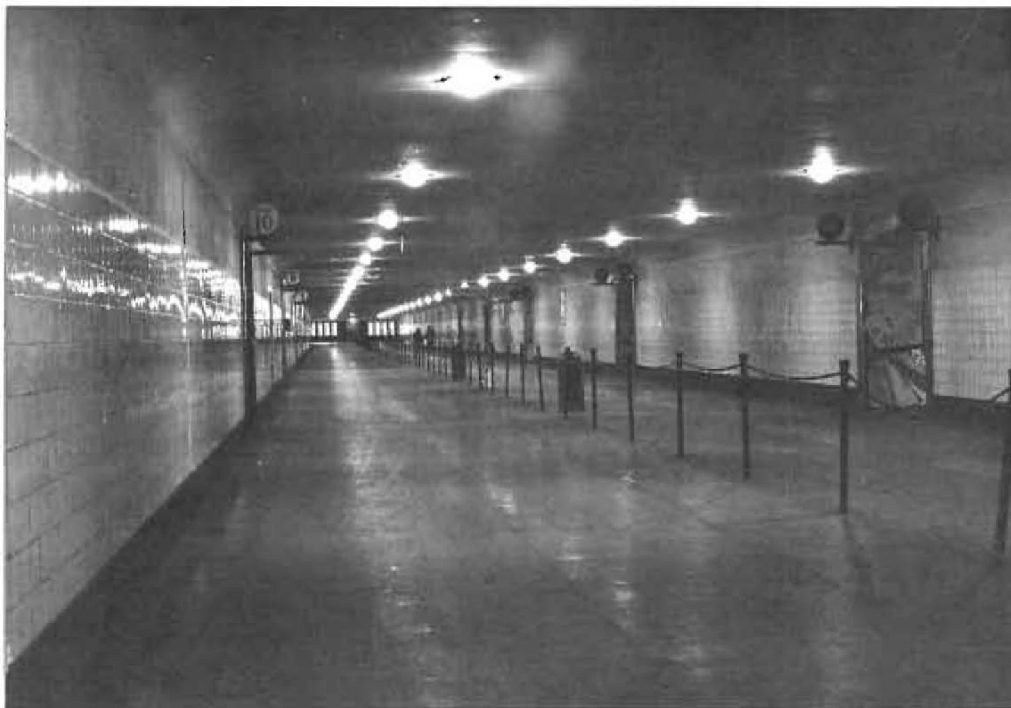
The passenger subway leading to the train platforms
