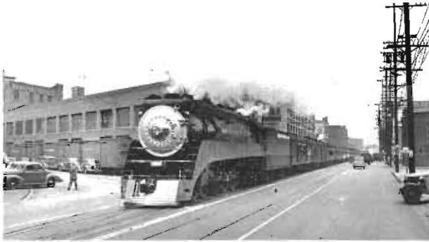
(Above) BEFORE UNION STATION went into service, trains passed along Alameda St. on their way to Southern Pacific's Central Station. The traffic congestion that this caused was one reason why the city and the railroad commission called for grade separation and a new station at the Plaza. Southern Pacific's suggested answer to this problem was to reroute the trains across the Los Angeles River, and connect them by elevated tracks to the station. Seen here on Alameda at Second St. is Southern Pacific's Lark , arriving from San Francisco, about 1938. Stan Kistler
