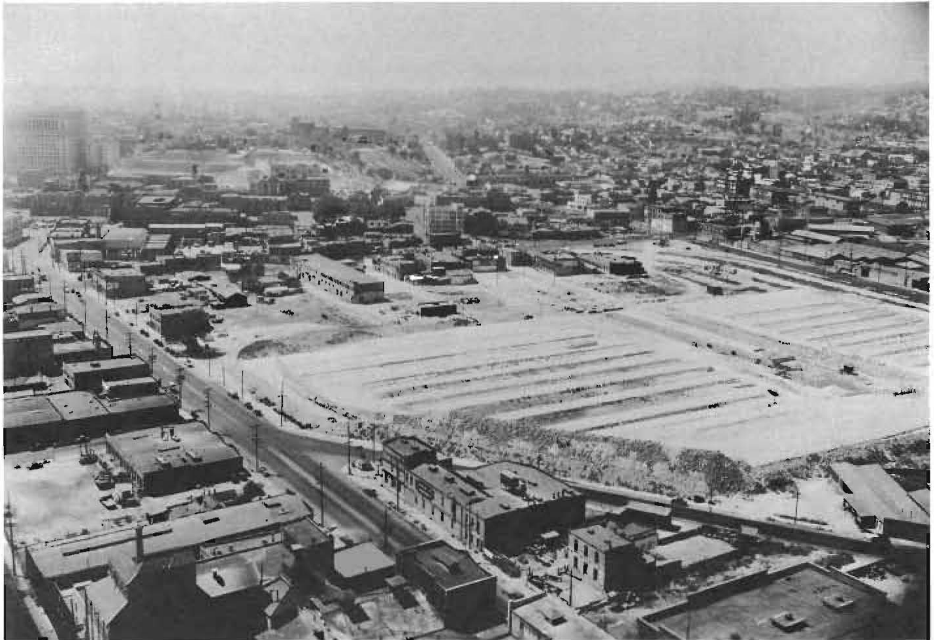
COMPARE this photo with the one on page 57. The first phase of construction involved moving a massive 400,000 cubic yards of earth to raise tracks 12 feet above Macy Street (right) and 16 feet above Aliso Street (left). When this picture was taken in 1935, work had already begun on the 500-foot-long subway that would connect passengers with the tracks. Progress on the rest of the site was delayed as controversy raged over the location of the Post Office Terminal Annex. California Historical Society/Title Insurance (Los Angeles)
