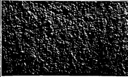
Architectural concrete walls are used throughout the Los Angeles Union Passenger Terminal Buildings planned and designed by Architects H. L. Gilman of the Santa Fe, J. H. Christie of the Southern Pacific, and R. I. Wirth of the Union Pacific, John Parkinson and Donald B. Parkinson, consulting architects. (Inset) Characteristic wall texture obtained with Celotex form lining.
