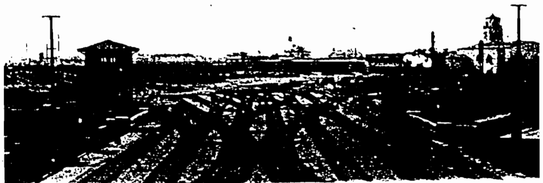
Looking Toward the Terminal Over a Part of the Highly Flexible Track Arrangement Provided—Note the Terminal Interlocking Tower at the Left
