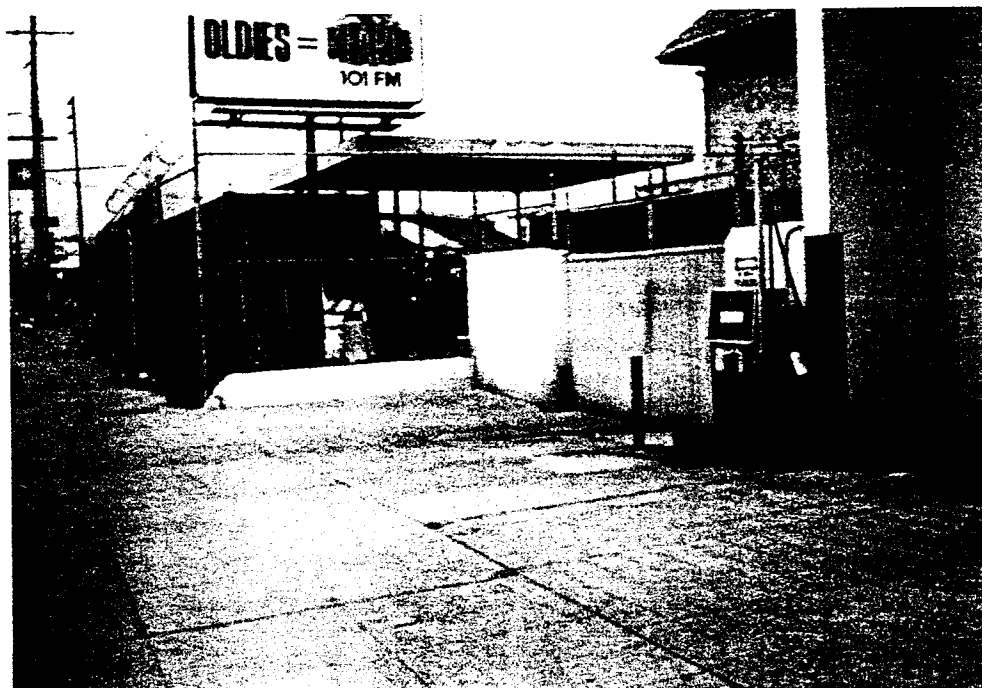
Photograph 12: View to the north of the fuel dispenser located in front of the City of Los Angeles Fire Station No. 4. To the north is the unidentified equipment yard located at the corner of Main and Vignes Streets.
