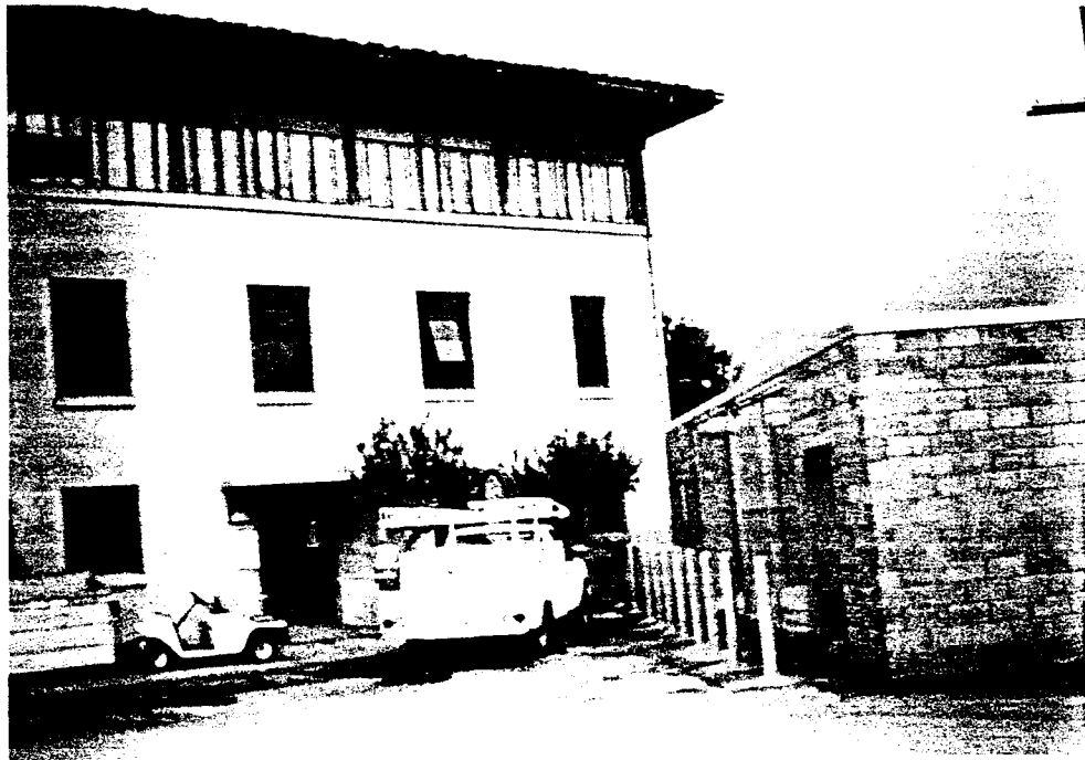
Photograph 7: View to the north of the AMTRAK switching tower and the new power enclosure currently under construction by the Metropolitan Transit Authority (MTA).
