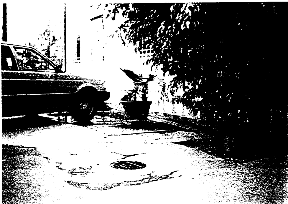
Photograph 5: View to east of the clarifier located near the AMTRAK office at the eastern boundary of the site. Groundwater monitoring well MW-10 is visible in the foreground.
