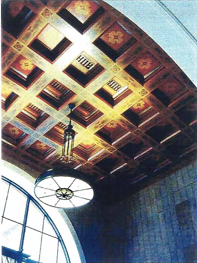
SOUTH VESTIBULE CEILING AND ADJACENT ACOUSTICAL TILE WALL SURFACE
