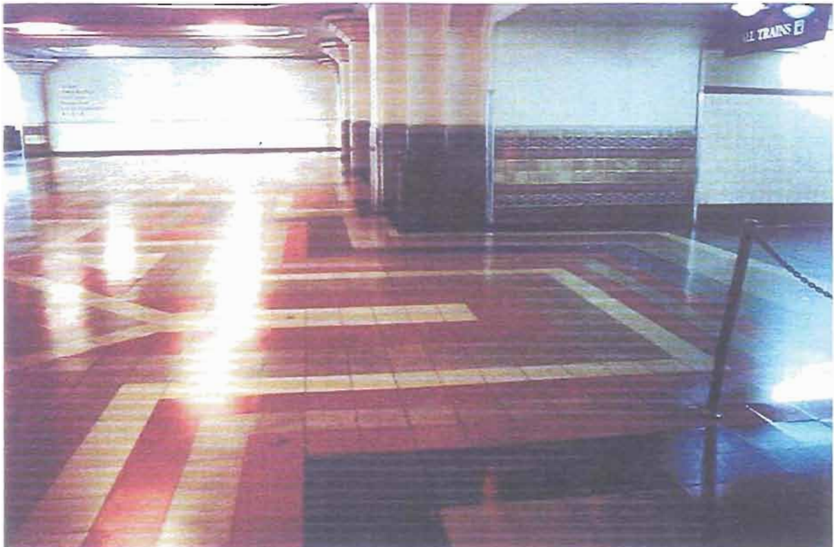
TUNNEL WEST ENTRANCE (RIGHT) AT PASSENGER LOBBY
