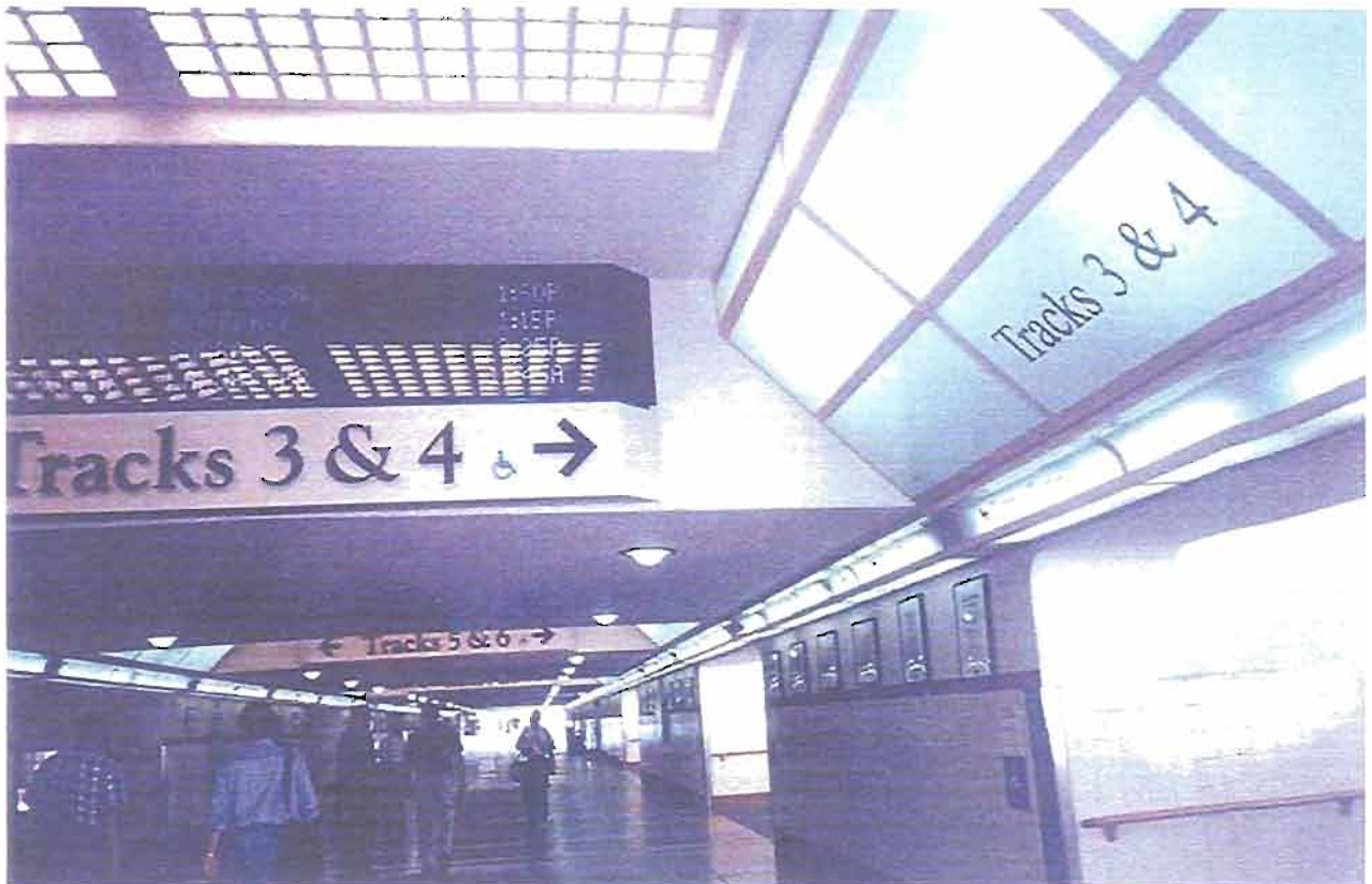
TRACK ENTRANCES AT EAST END OF TUNNEL (VARIED CEILING HEIGHT IS NOT A HISTORIC CONDITION)
