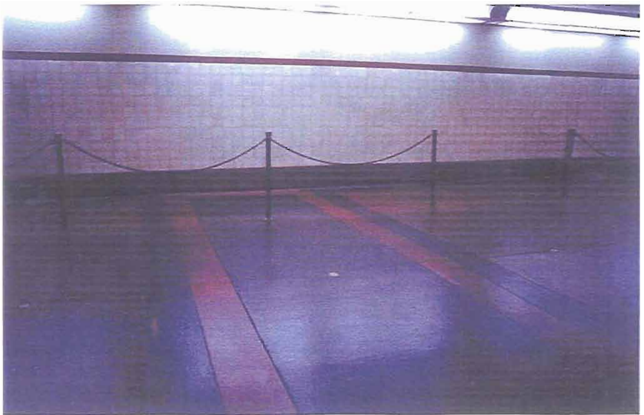
TUNNEL: CONCRETE FLOOR AND NON-HISTORIC WALL TILE
