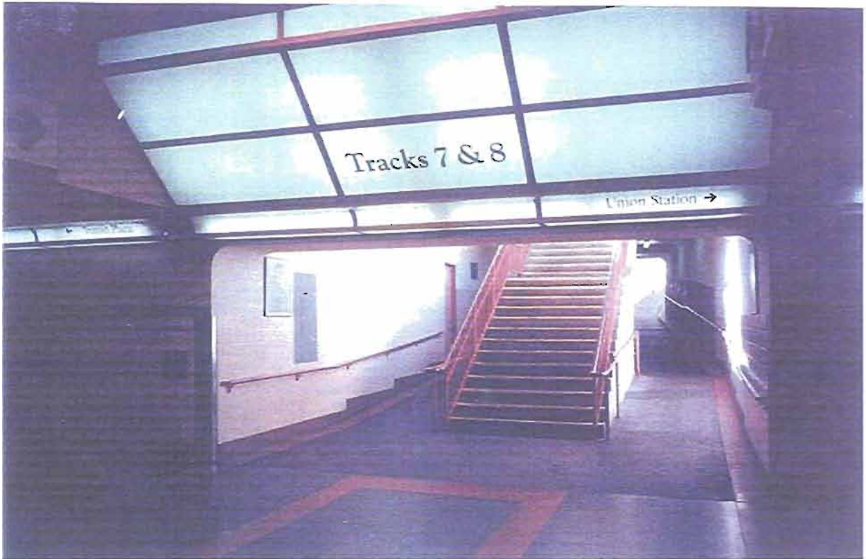
TYPICAL SOUTH SIDE TRACK ENTRANCE WITH STAIRS TO PLATFORM AND RAMP BEHIND; STAIR RAILING IS NOT HISTORIC
