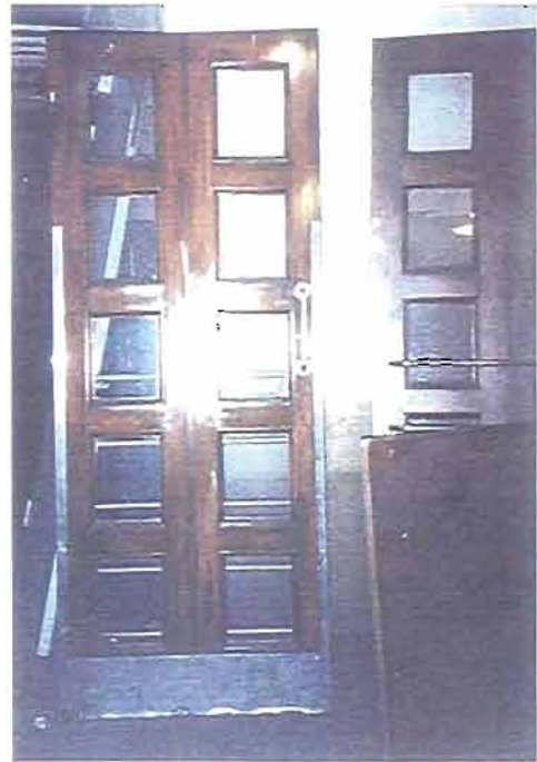
LEFT: NONORIGINAL DOORS ON EAST SIDE OF SOUTH PATIO IN ARCHWAY THAT WAS ORIGINALLY OPEN AND UNGLAZED. RIGHT: DOORS FOUND IN STORAGE, WHICH WILL REPLACE NON-ORIGINAL DOORS TO SOUTH PATIO.
