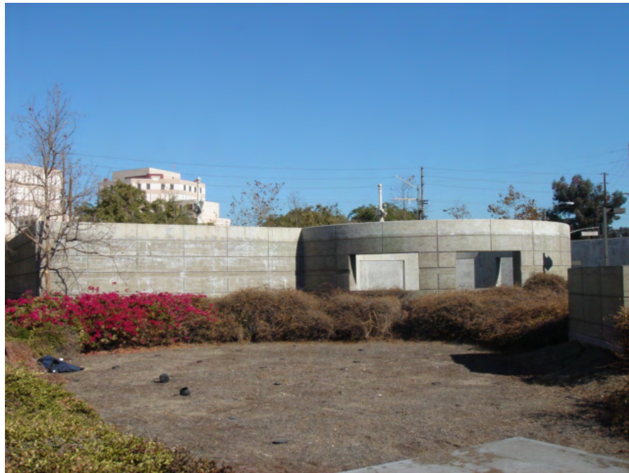
View of Area 3
