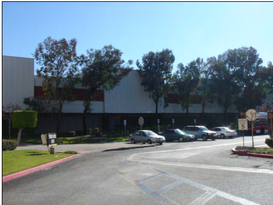
View of Building 1 in Area 2 Facing Southeast
