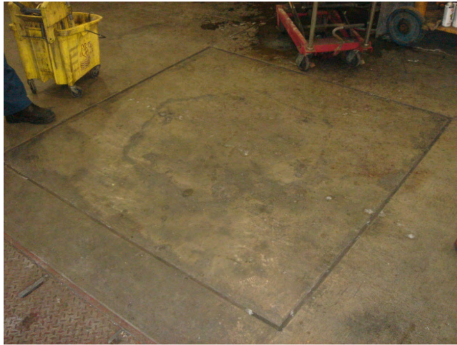
View of slab from removal of previously mounted equipment in Building 1
