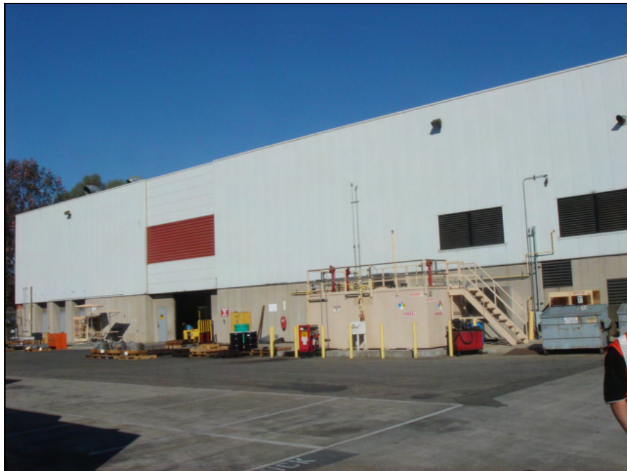
View of Building 1 in Area 2 Facing Northwest
