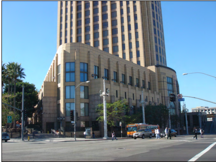
View of Metro Headquarters southwest of Area 1
