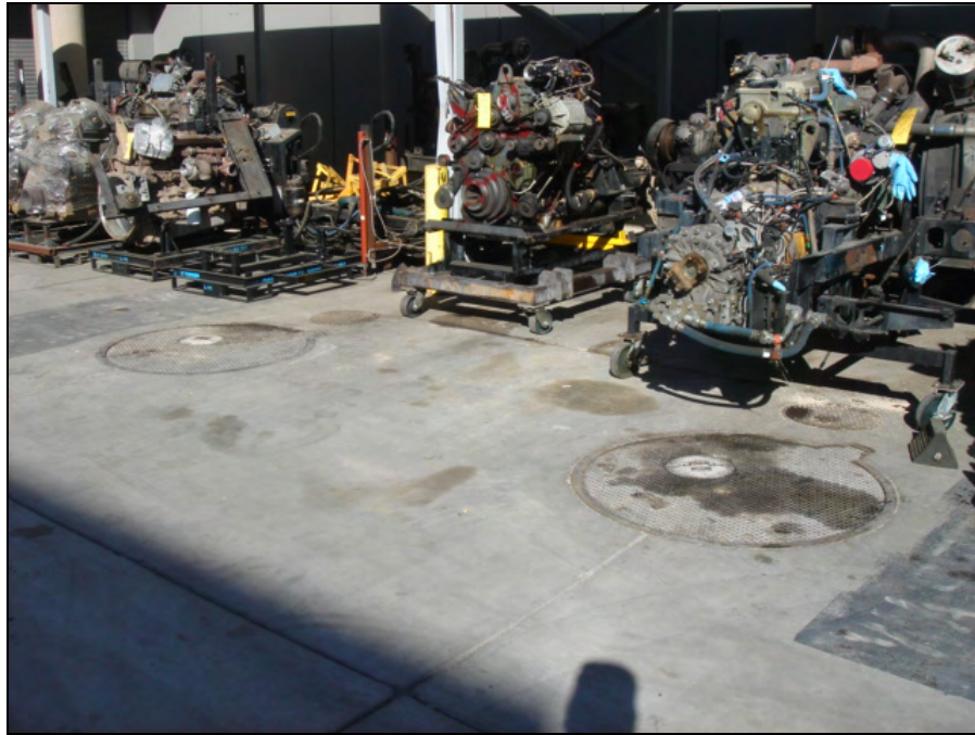
View of top of USTs with engines to be rebuilt north of Building 1
