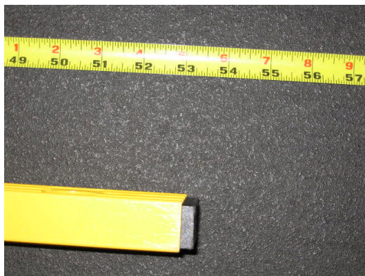
Measurement indicating that the resting landing is less than the required 60".
