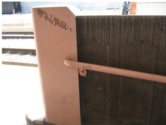
Handrails do not extend beyond the top of the ramp and does not extend at the bottom of the ramp.
