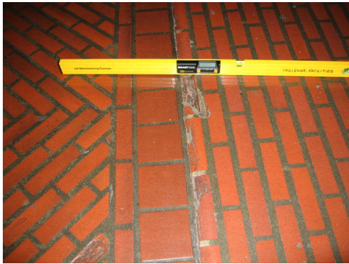
Tripping hazard on the south side walkway Uneven floor in the patio
