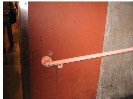
Handrails do not extend beyond the top of the ramp and does not extend at the bottom of the ramp.
