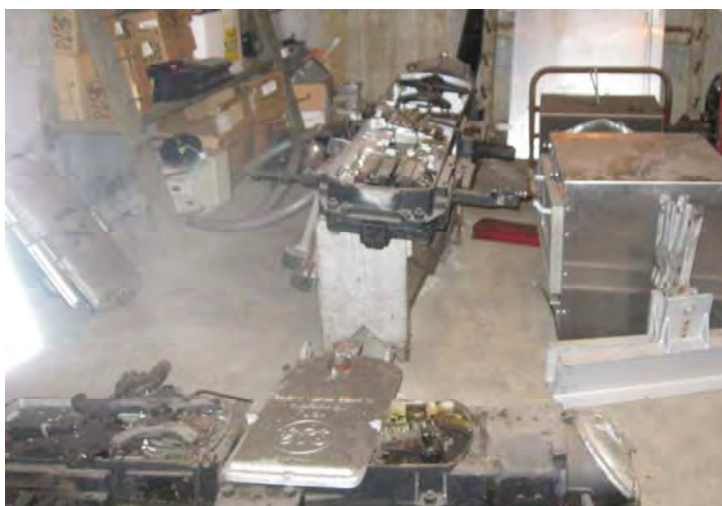
Interior of basement of Amtrak Switch Building.
