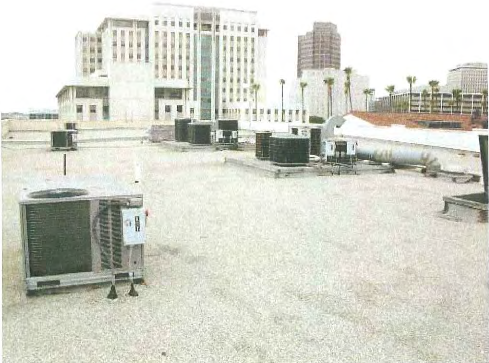
Photo #1 – General overview of roof.
