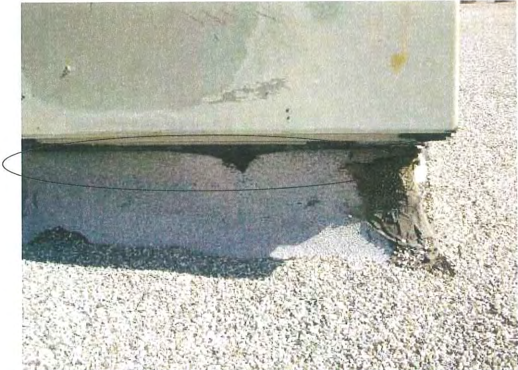
Photo #2 – Top of base flashing exposed.
