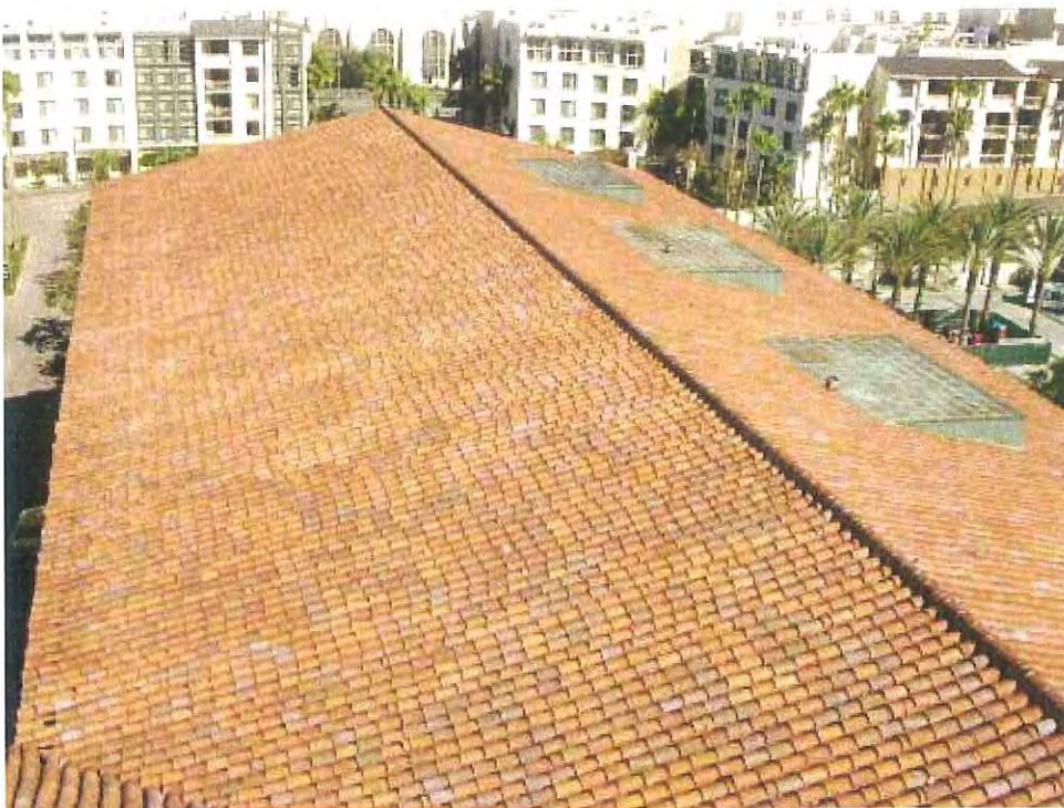
Photo #1 – General overview of North roof area.
