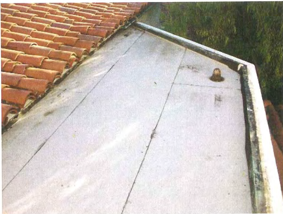
Photo #8 – General overview of Southeast APP modified roof area.
