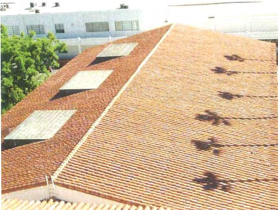
Photo #3 – General overview of East roof area.
