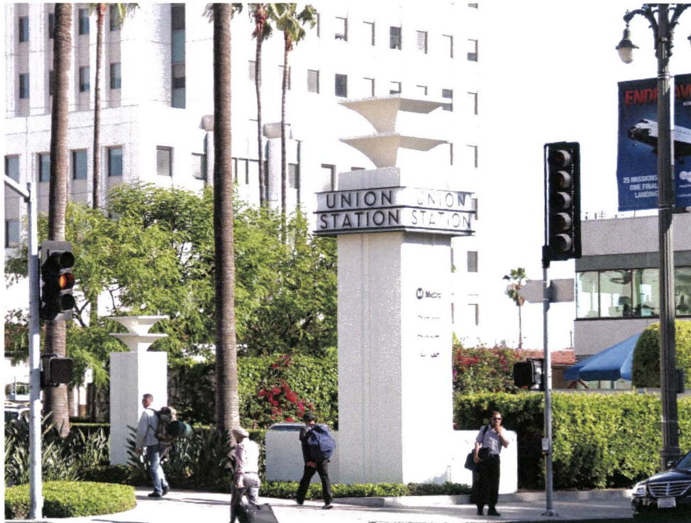
Columnar Wayfinding structures Forecourt
