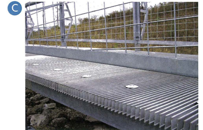
Metal Grate Walkway
