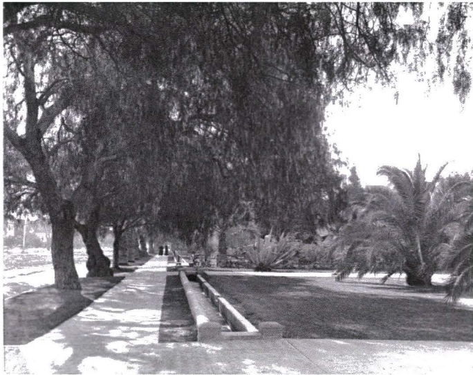
Zanja Madre Aqueduct System on Figueroa Street
