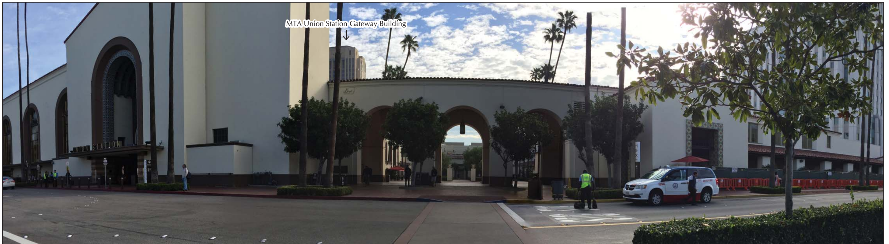
PHOTO 20. Southern Pedestrian Path Towards Southern Union Station Courtyard in February 2017 – Facing East
