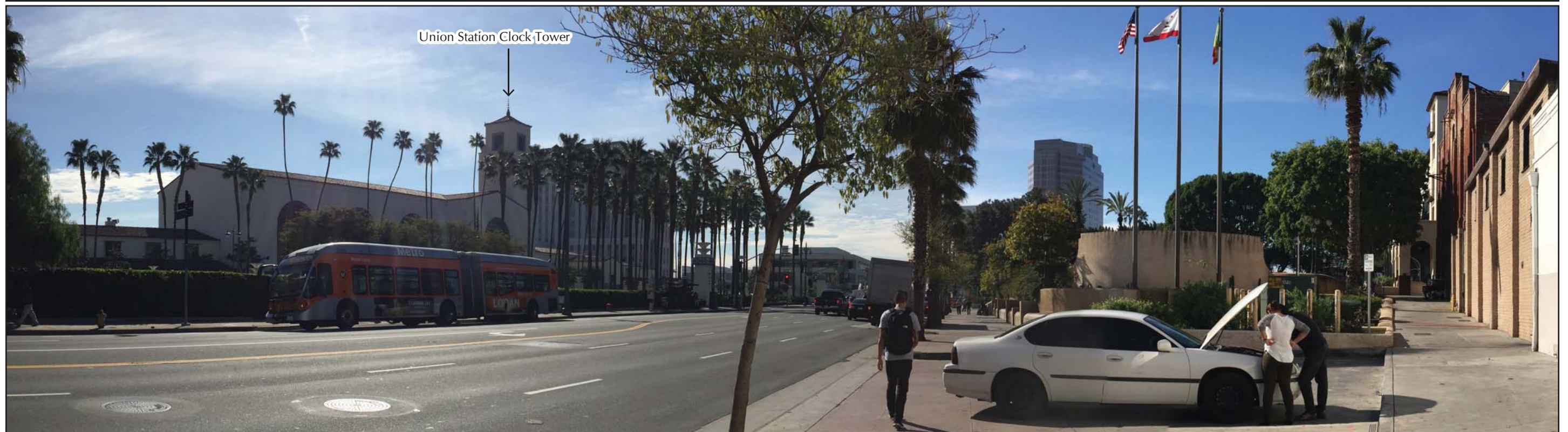
PHOTO 31. Union Station Terminal From Alameda Street in February 2017 – Facing Southeast
