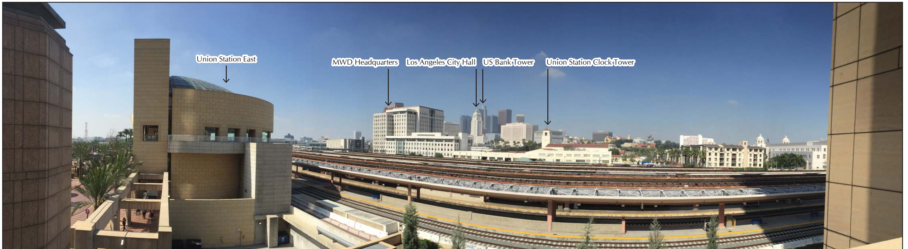
PHOTO 10. MTA Union Station Gateway Building at Union Station East in April 2016 – 3rd Floor Balcony – Facing Southwest
