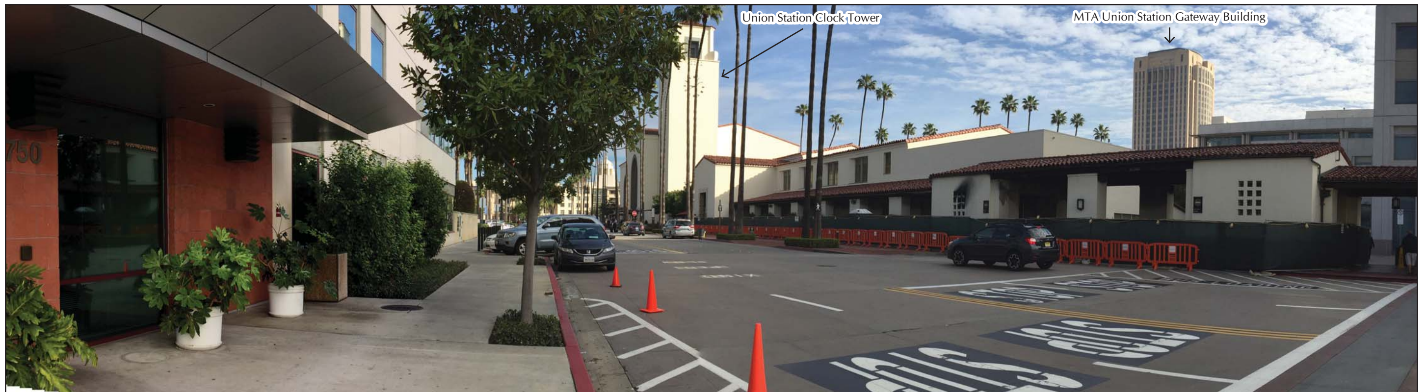
PHOTO 17. Sidewalk Adjacent to First 5 LA Building Entrance in February 2017 – Facing Northeast
