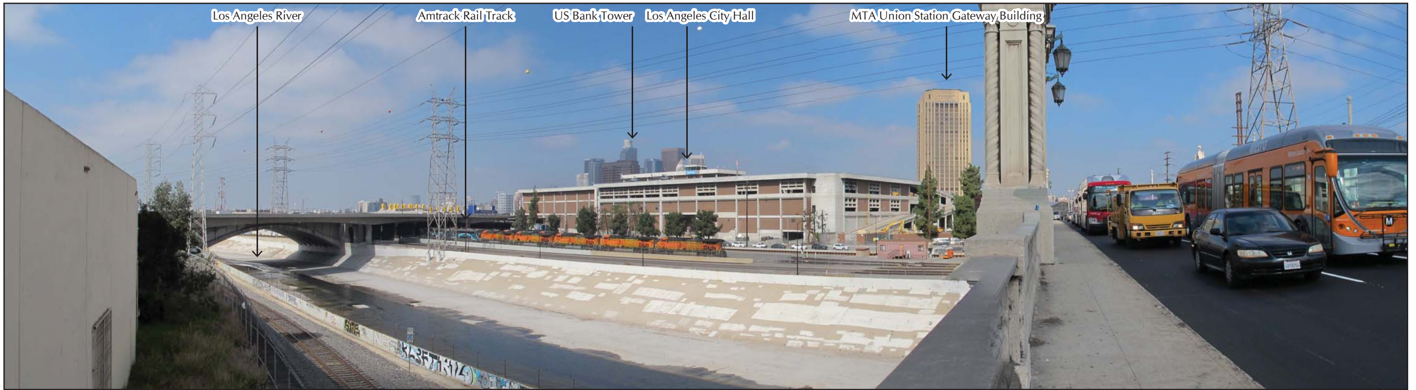
PHOTO 9. Historic Macy Street Viaduct on East Cesar E Chavez Avenue in April 2016 - Facing West
