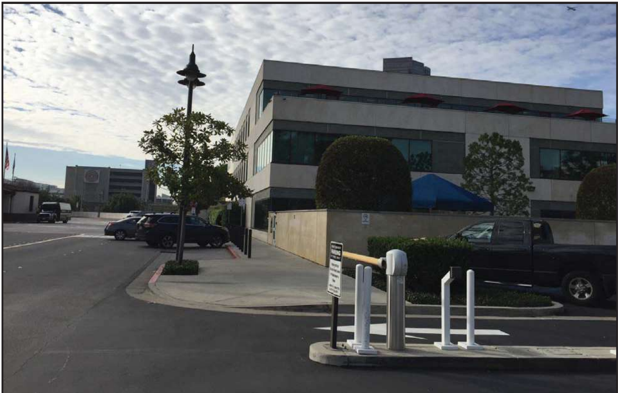
PHOTO 18. First 5 LA Parking Lot and Building in February 2017 – Facing South
