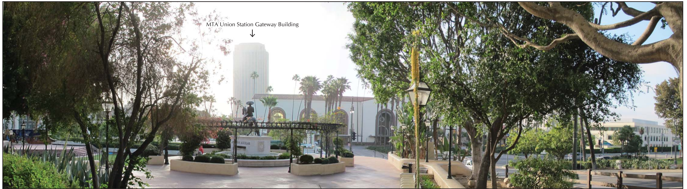
PHOTO 33. Los Angeles Plaza Park - View from Plaza Substation in April 2016 - Facing East
