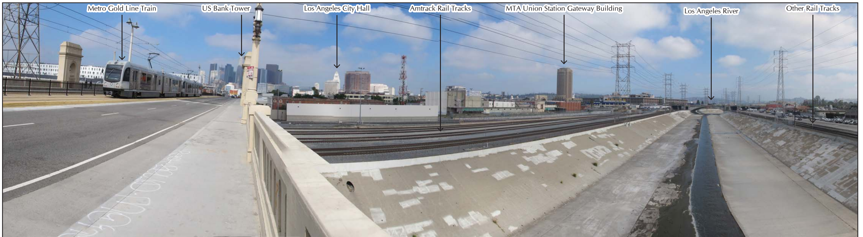
PHOTO 8. E 1st Street Bridge Over Los Angeles River in April 2016 - Facing North
