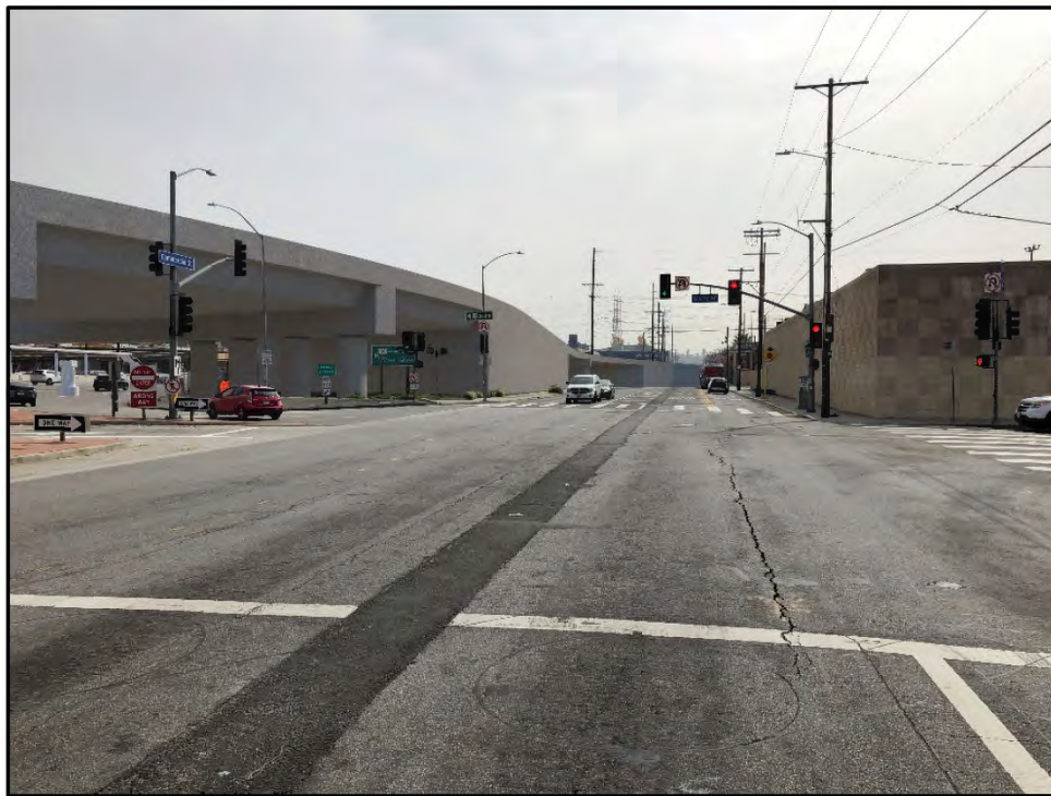
Figure 10-14. Key View #5c – Commercial Street (View Looking East from US-101 On-/Off-Ramps toward Embankment) Post-Final EIR Project Conditions
