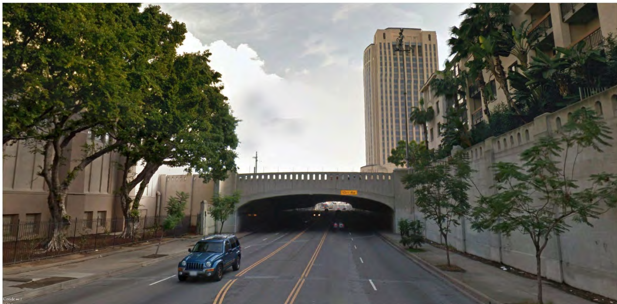
Figure 3.4-7. Key View #3b – Cesar Chavez Avenue (View Looking East from Road toward Bridge)
