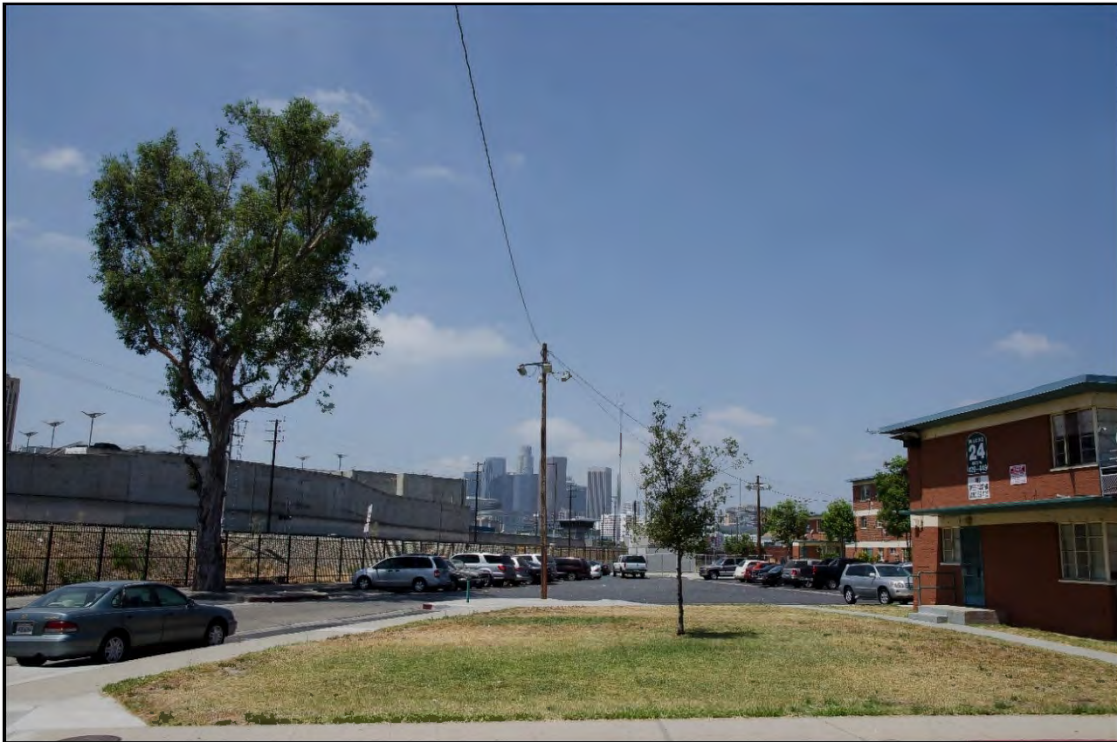
Figure 5-9. Key View #1a – Existing Condition (Retaining Wall)
