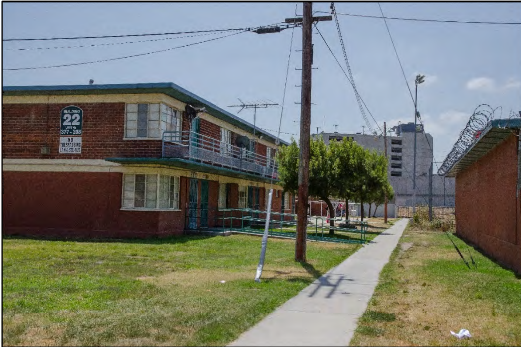
Figure 3.4-20. Key View #1b – Existing Conditions
