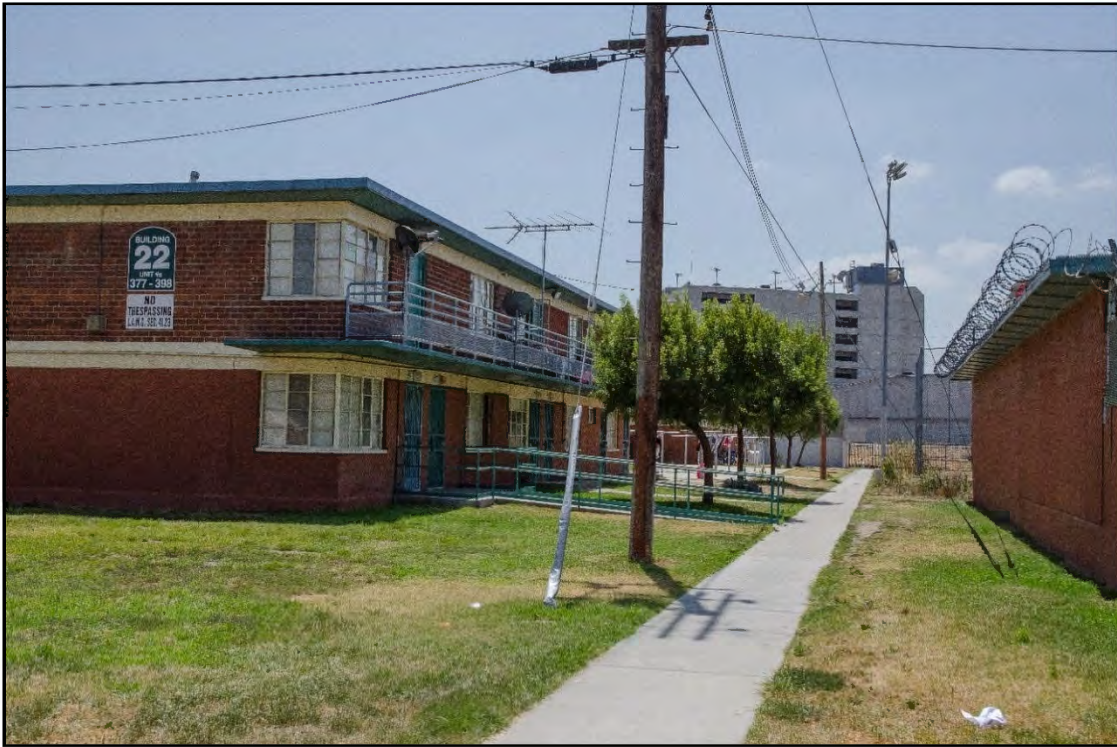
Figure 5-11. Key View #1b – Existing Condition (Retaining Wall)
