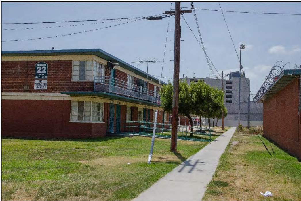
Figure 3.4-19. Key View #1b – Post-Project Conditions (Retaining Wall)
