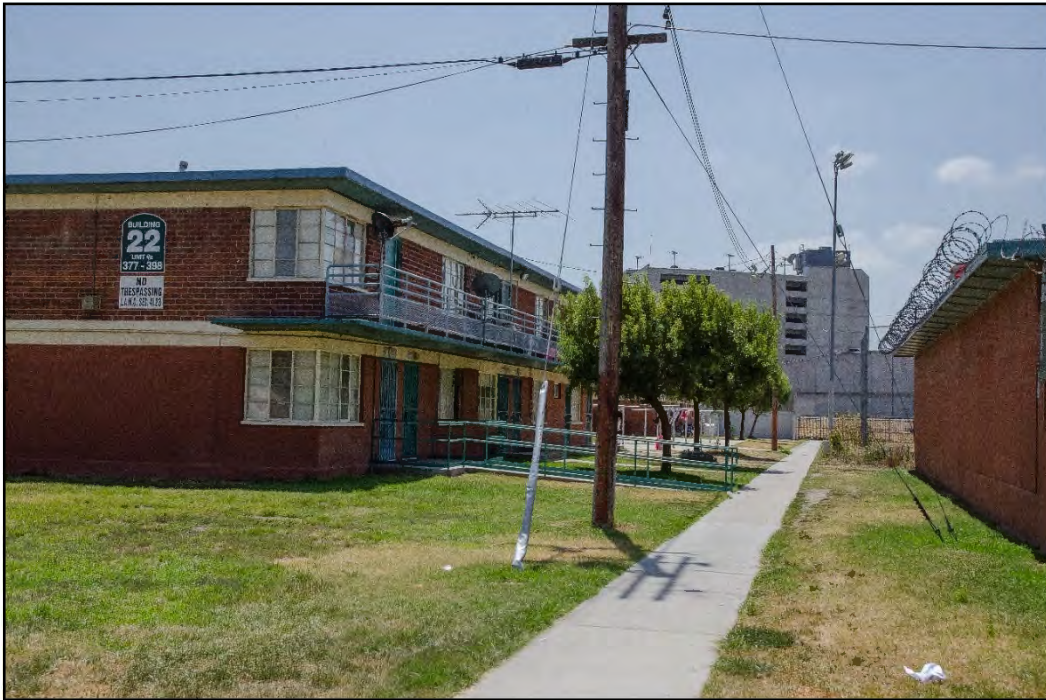
Figure 3.4-18. Key View #1b – Existing Conditions
