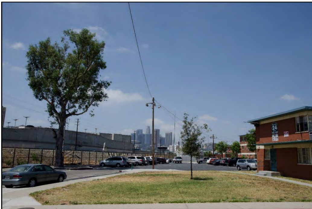
Figure 3.4-2. Key View #1a – William Mead Homes (View Looking Southwest from Corner of Bolero Lane/Bloom Street toward Railroad Right-of-Way)
