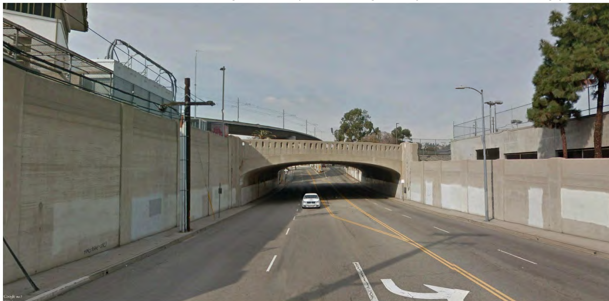
Figure 3.4-4. Key View #2a – Vignes Street (View Looking North from Road toward Bridge)
