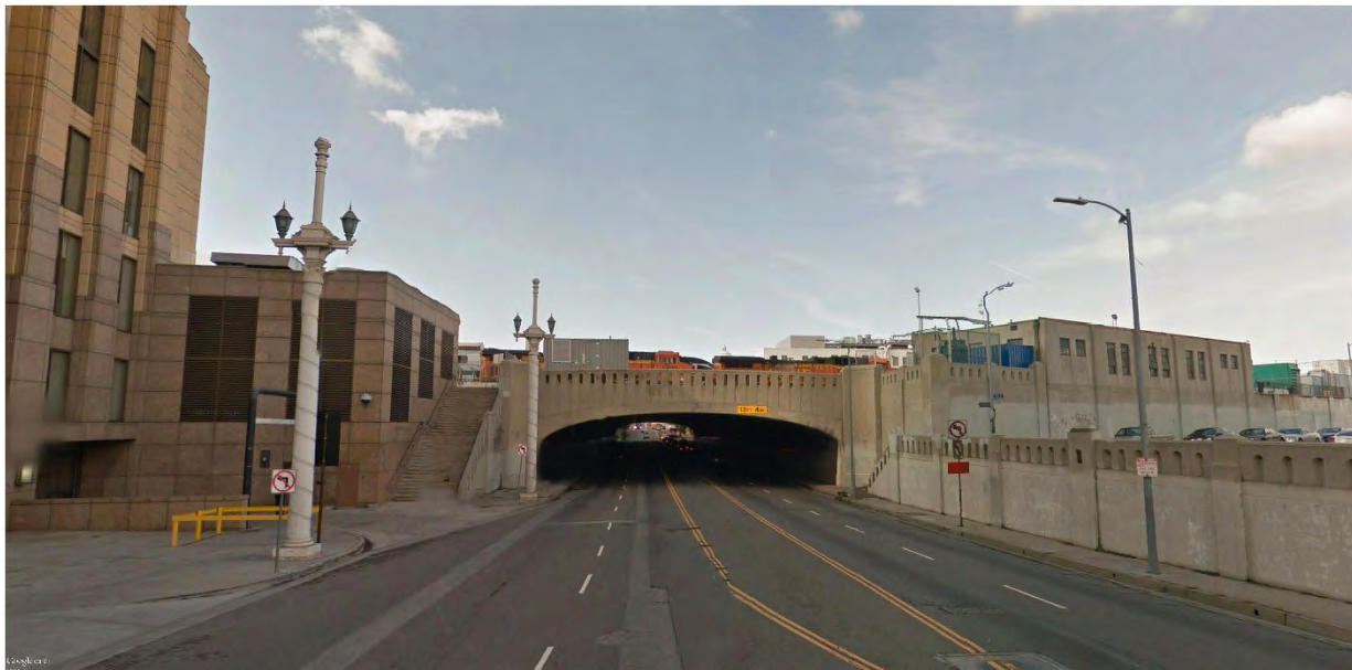
Figure 3.4-26. Key View #3a – Cesar Chavez Avenue (View Looking West toward Bridge) Existing Conditions
