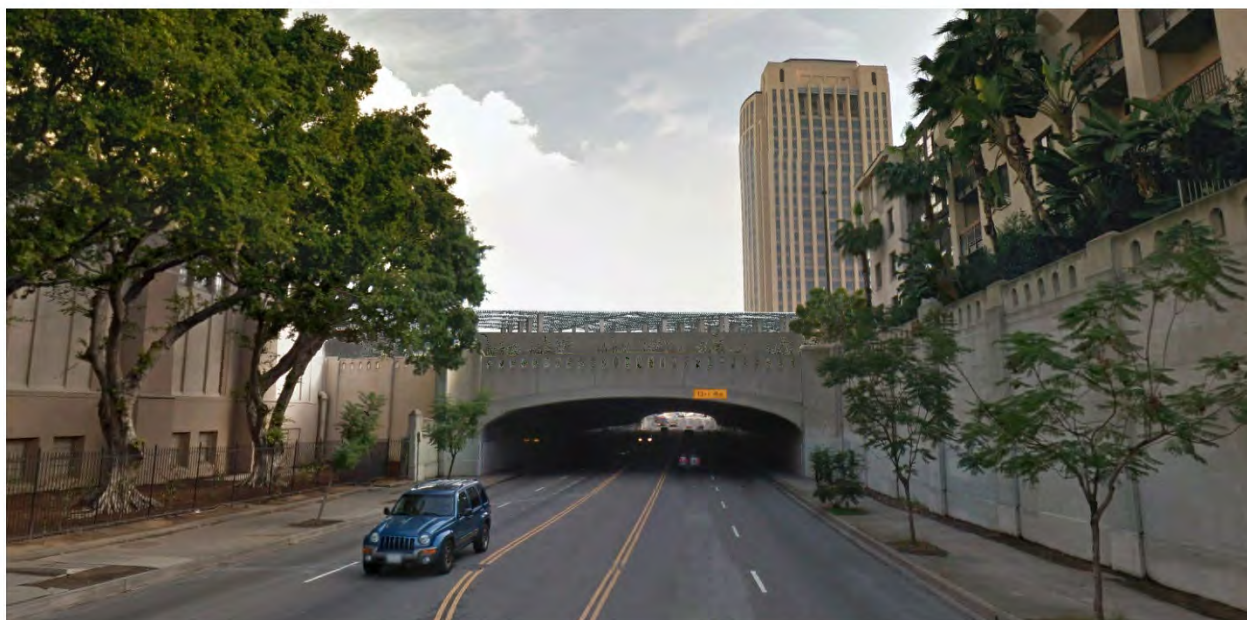
Figure 3.4-29. Key View #3b – Cesar Chavez Avenue (View Looking East toward Bridge) Post-Project Conditions
