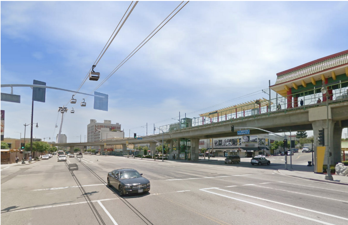
Figure 6-15: Simulation Views of the Alameda Tower under the proposed Project (top) and Design Option B (bottom) – Looking South on Spring Street/Alameda Street from just North of College Street
