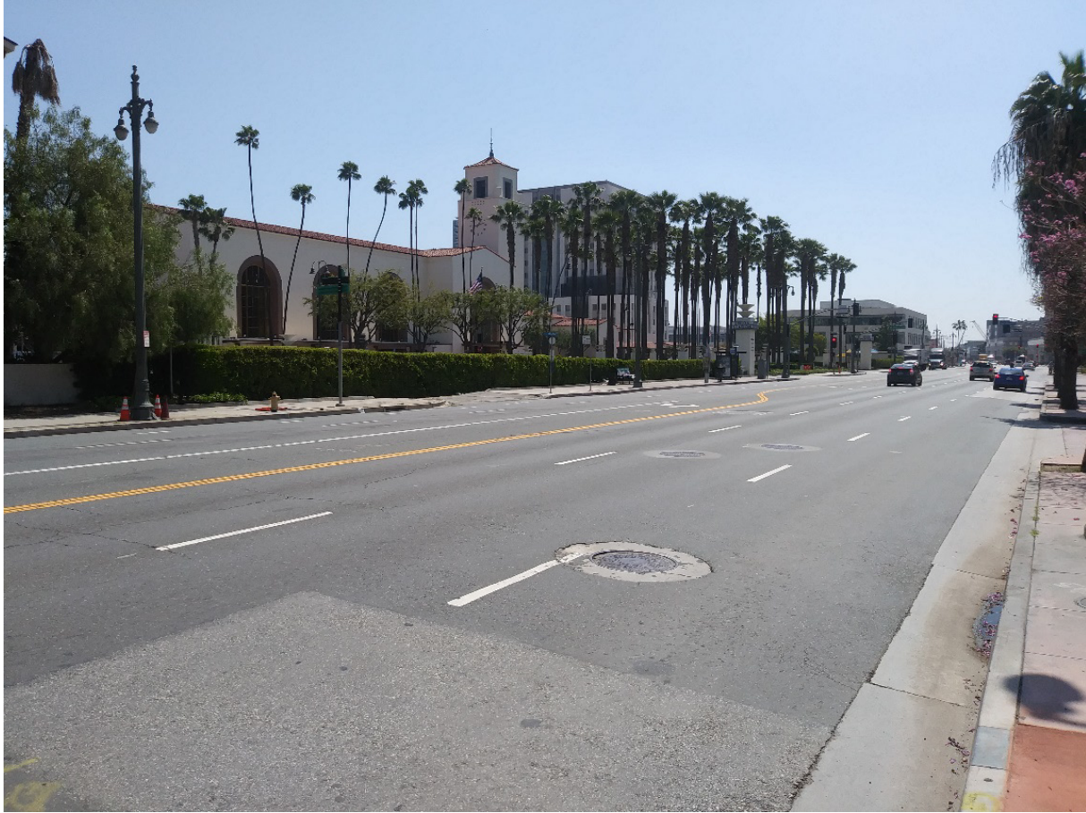
Figure 3.1-3: Existing View of LAUS Looking South along Alameda Street
