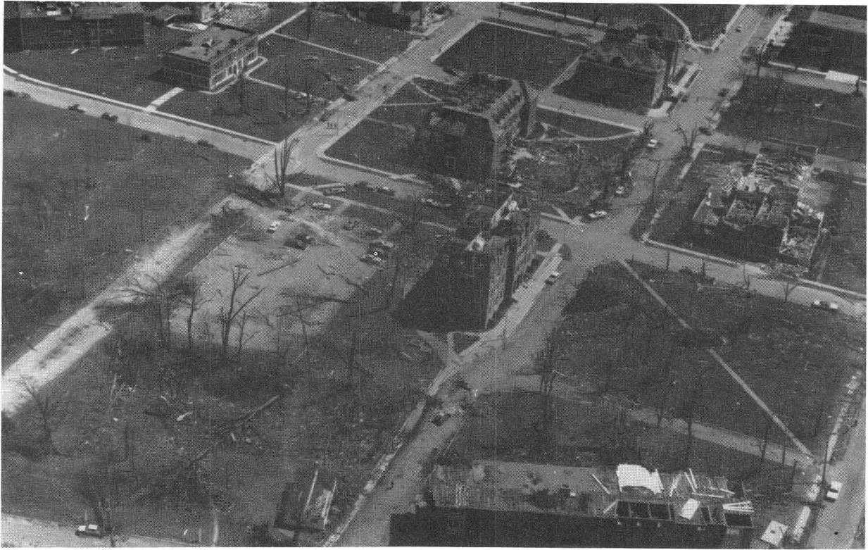
Damage from tornadoes of April 3, 1974, in Xenia, Ohio
