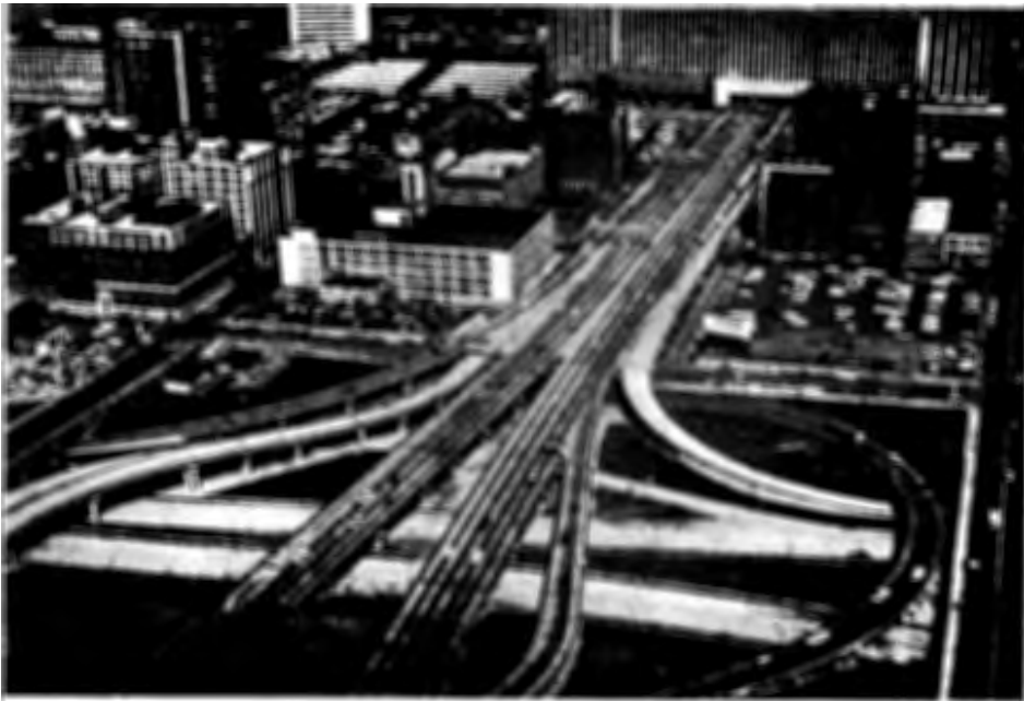
The United States Post Office over the Eisenhower Expressway on the west edge of downtown Chicago is another of America's best-known airspace developments. The view is of the east wall which faces downtown. April 1962 photograph courtesy of State of Illinois, Public Works & Building Department, Division of Highways, District 10.
