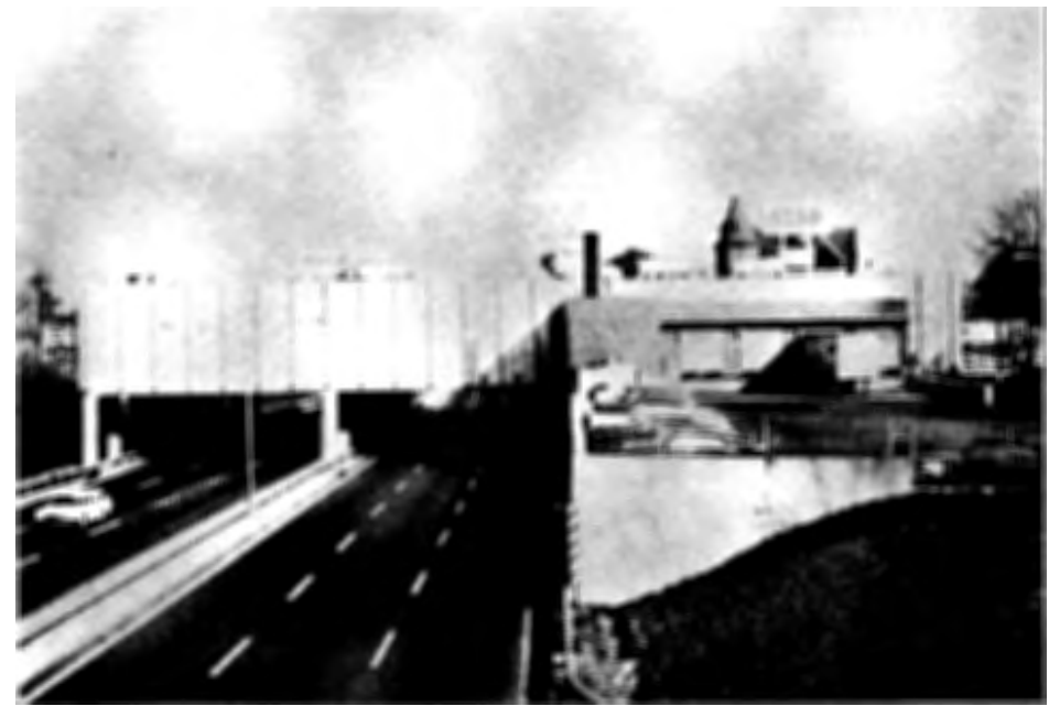
The Star Market is a freestanding neighborhood store. The nearest freeway off-ramp is more than one mile in either direction. Note the hazardous edge of highway abutment.
