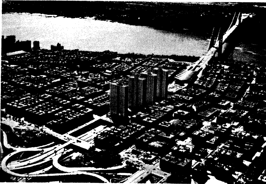
The four Bridge Apartments (960 units) and three-level Uptown Bus Station in New York City over the approaches to the George Washington Bridge spanning the Hudson River are one of the nation's best known freeway airspaca projects. July 1963 photograph courtesy of The Port of New York Authority.
