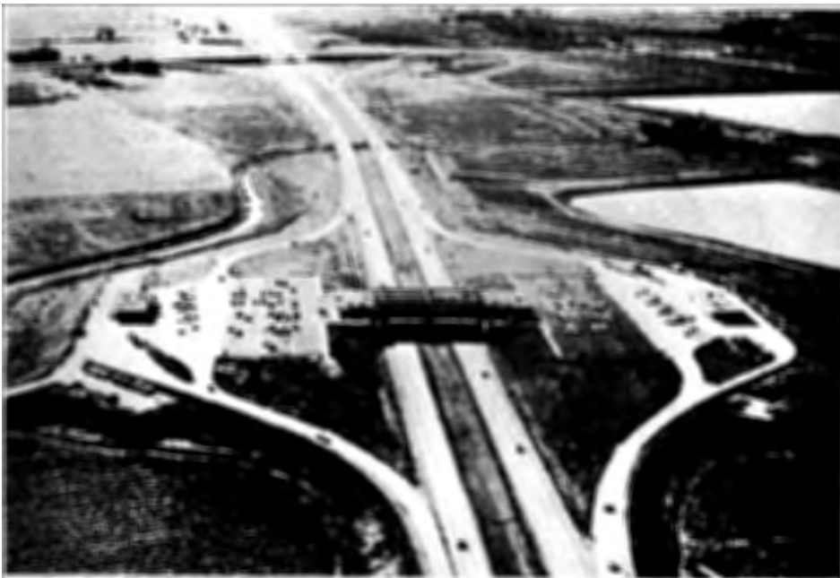
The Des Plaines Oasis, located over Interstate 90 one mile northwest of Chicago's O'Hare International Airport, is one of five identical facilities. The Fred Harvey Restaurants on the horizontal bridges are flanked by Standard Oil Stations which serve passenger cars and trucks.
