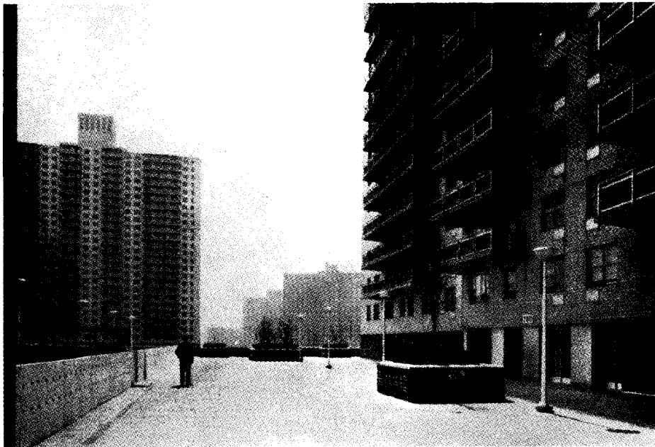
Concourse Village high-rise apartments after completion. The open deck serves as a play and recreation area and makes it possible for efficient snow removal during the winter. The 1965 photograph courtesy of Amalgamated Meat Cutters and Butcher Workmen of North America.
