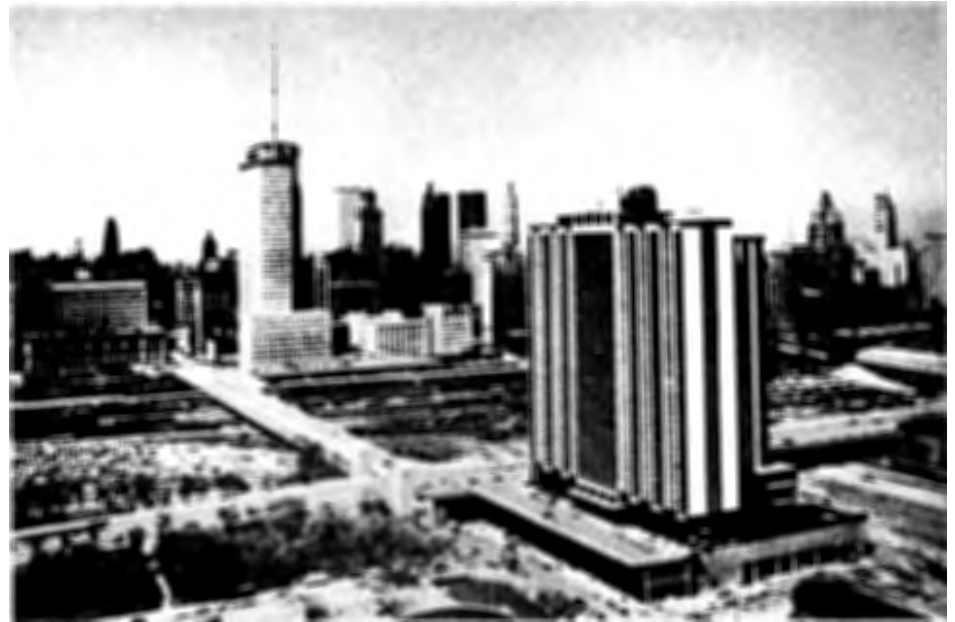
Outer Drive East —These luxury apartments (940 units) are on the shore of Lake Michigan at the east edge of downtown Chicago, Illinois. The Prudential Tower beyond the Illinois Central Railroad yard also fronts on Randolph Street. August 1966 photograph courtesy of Prudential Insurance Company of America.
