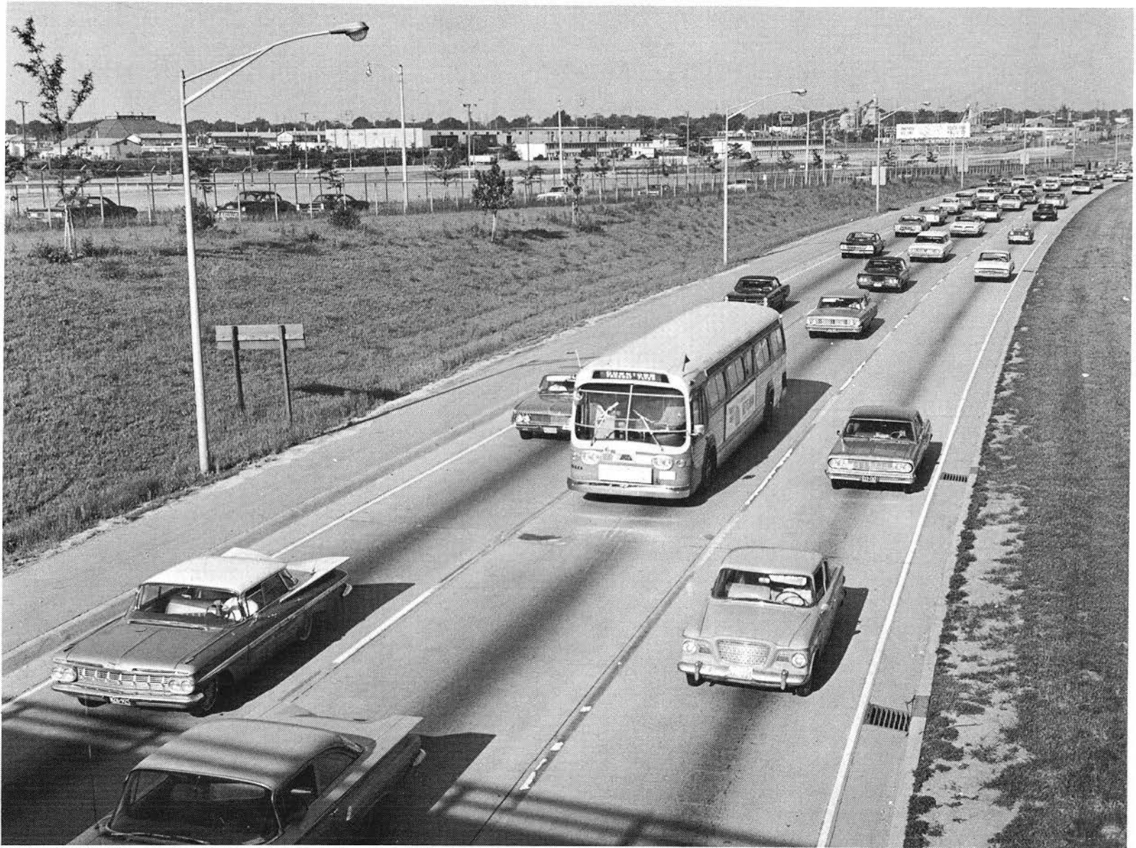
FREEWAY FLYER ON EAST-WEST FREEWAY
