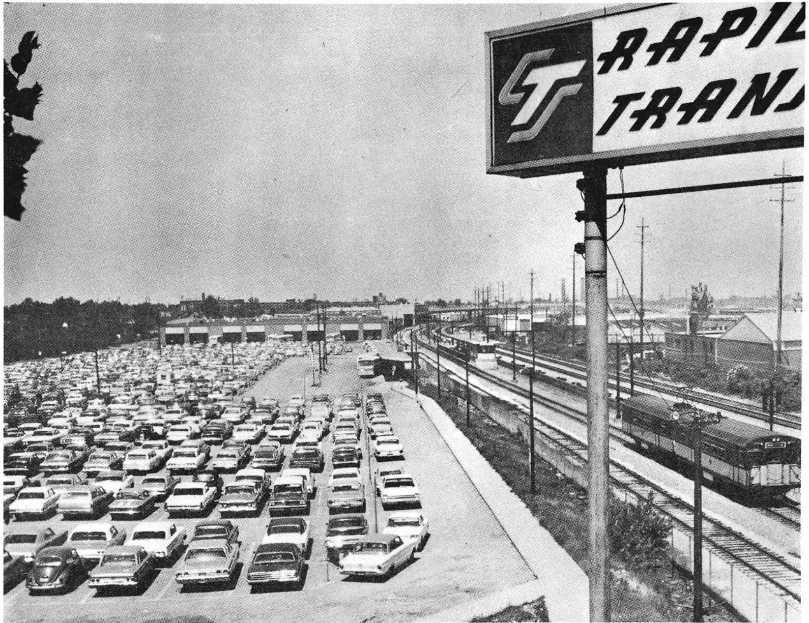
TRISKETT RAPID TRANSIT STATION FACILITIES FOR PARKING 1, 200 AUTOS AND SEPARATE LANES FOR 20 KISS 'N RIDE CUSTOMERS
