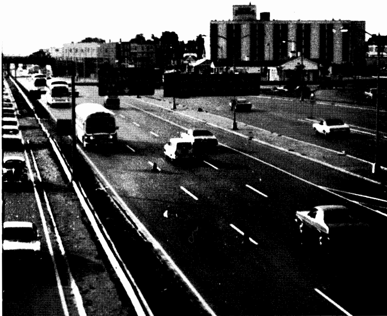
Figure 3 - 10 BOSTON SOUTHEAST EXPRESSWAY PERMANENT LANE SIGNS
