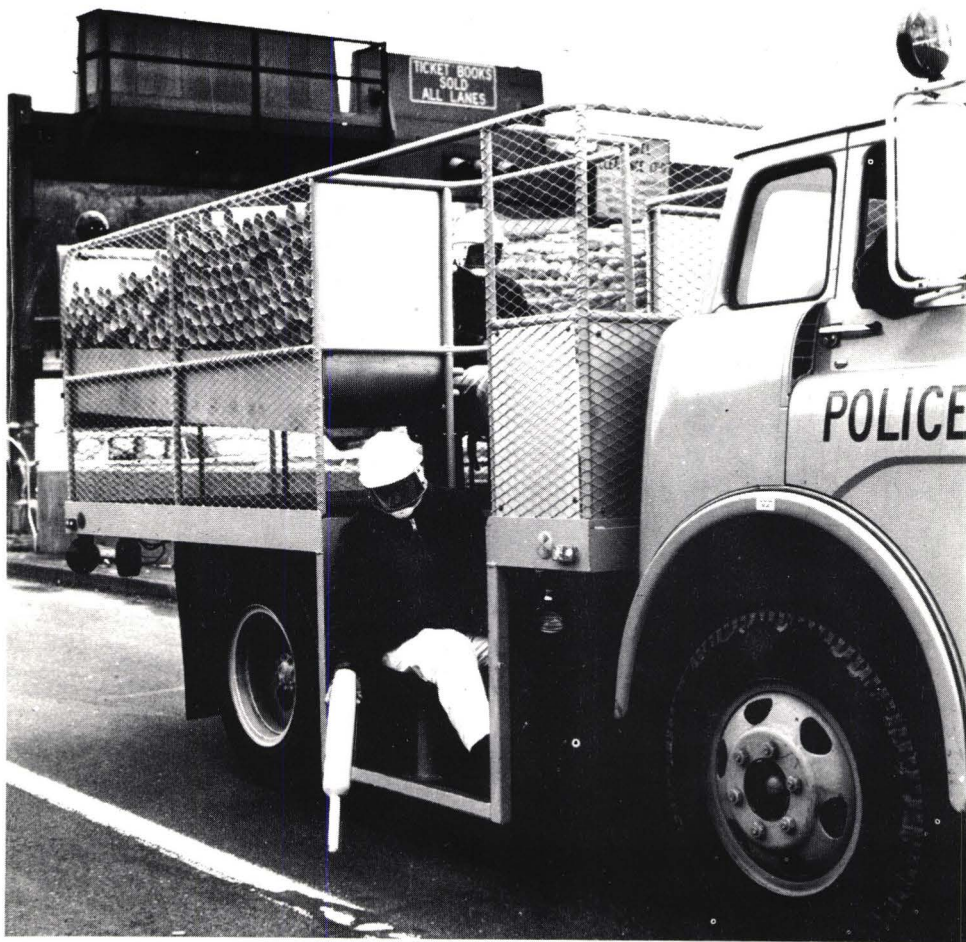
Placement of traffic posts each morning prior to contra-flow operation.
