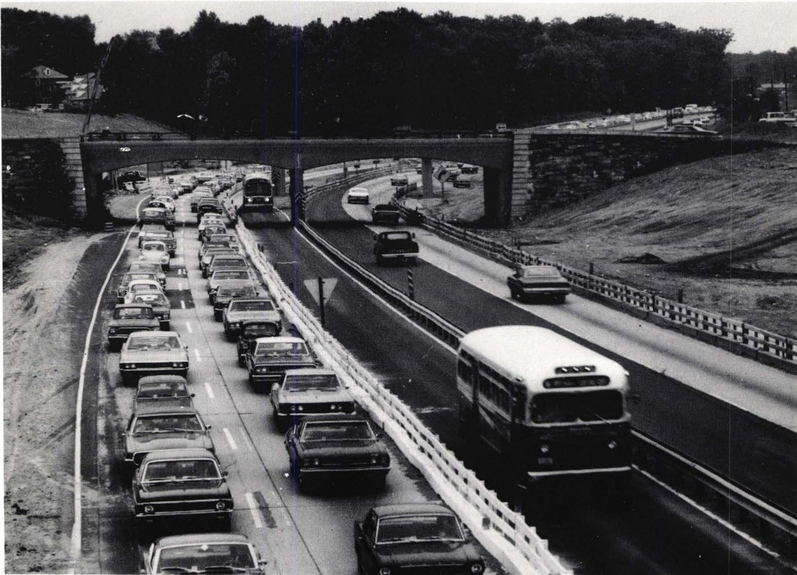
Temporary busway during Shirley Highway reconstruction.
