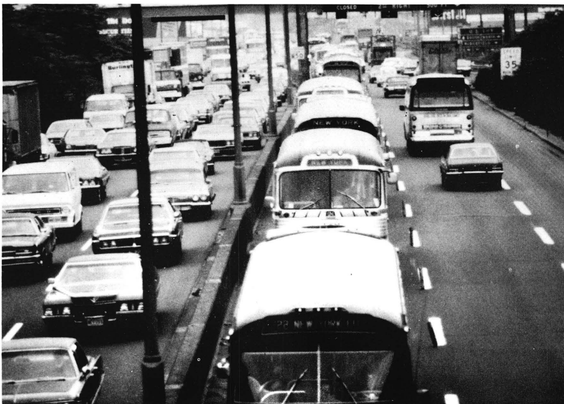
Contra-flow bus lane on I-495 approaching the Lincoln Tunnel.
