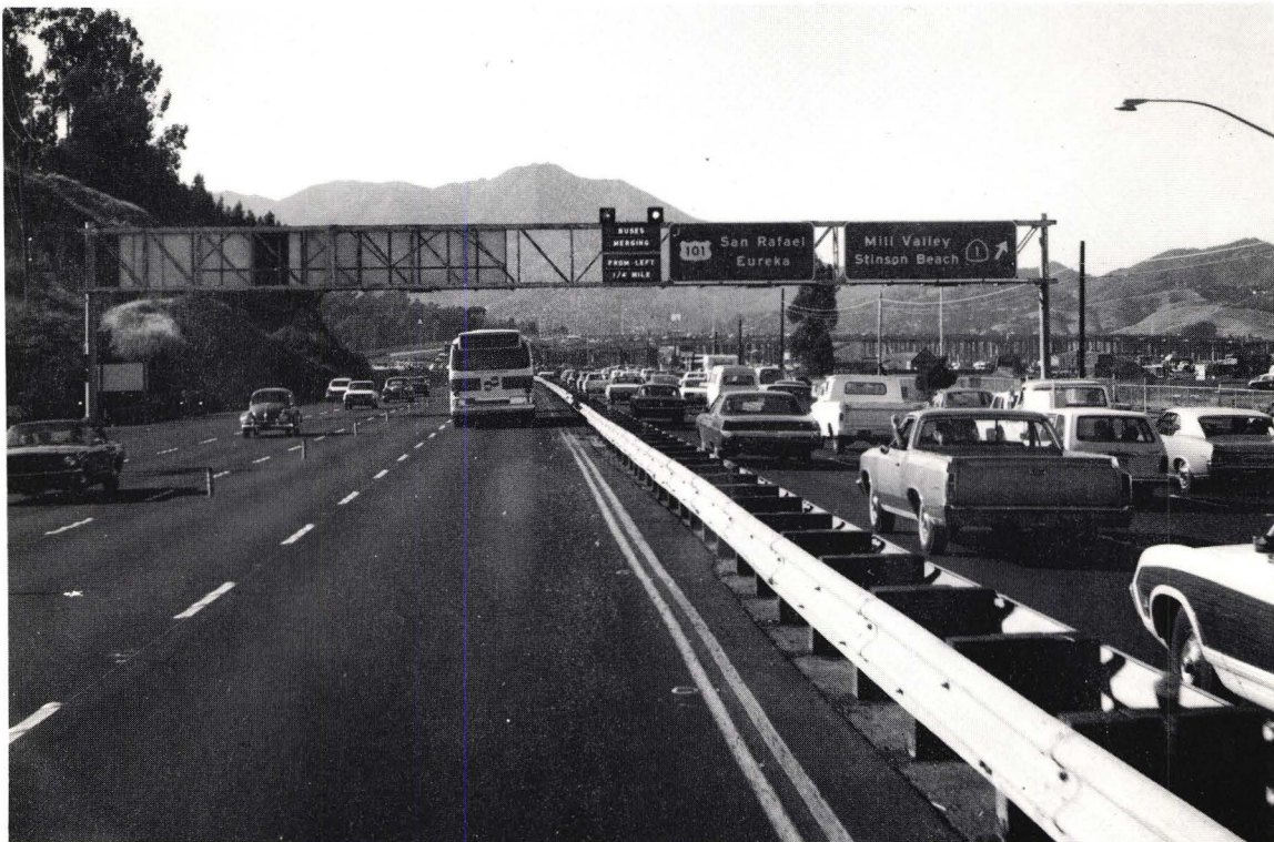
U.S. Route 101 contra-flow lane near Richardson Bay.
