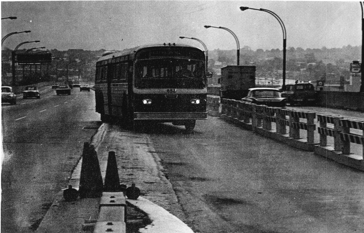
Buses enter the contra-flow lane via a median crossover.
