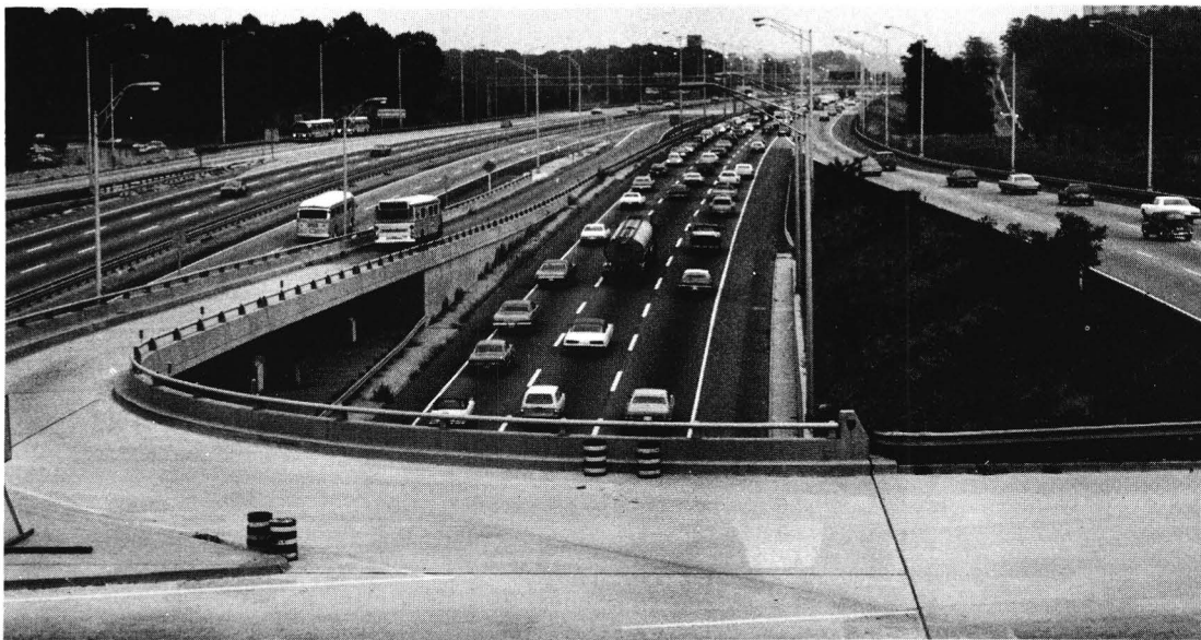
Exclusive bus ramp to Shirley Highway bus and carpool lanes.
