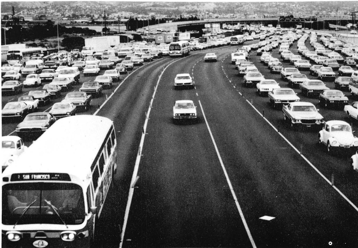
Exclusive bus and carpool lanes through the toll plaza of the San Francisco-Oakland Bay Bridge.
