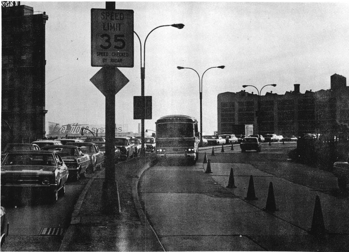
Contra-flow bus lane on the Long Island Expressway in New York City.
