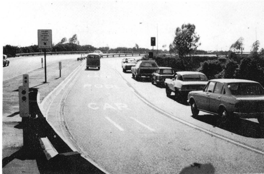
Operation of the carpool bypass lane.
