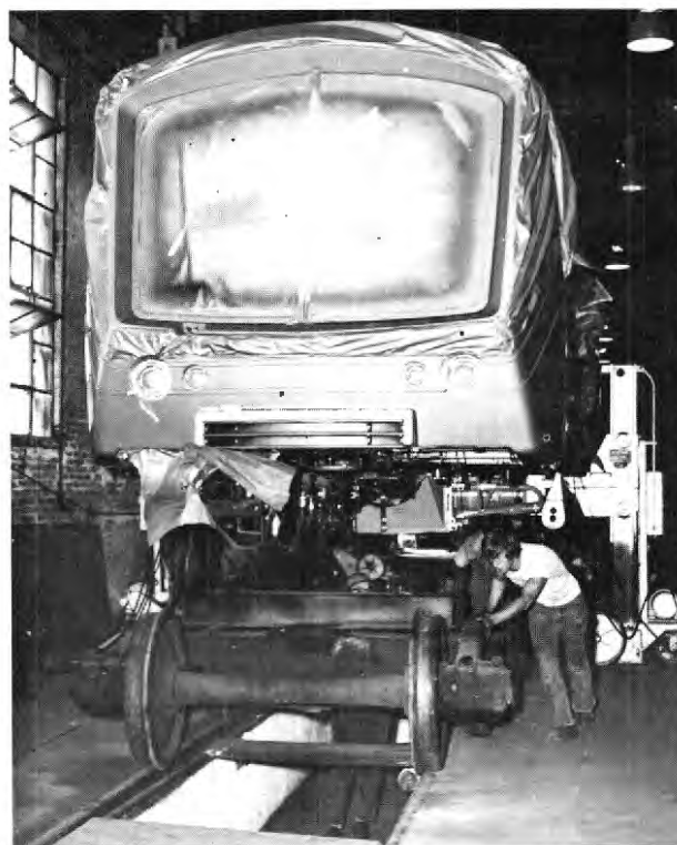
Figure 2-3. SOAC Construction, July 1972
