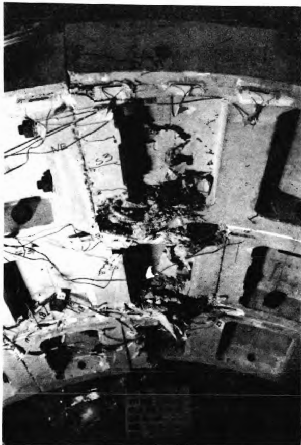
(a) View of failure from inside
