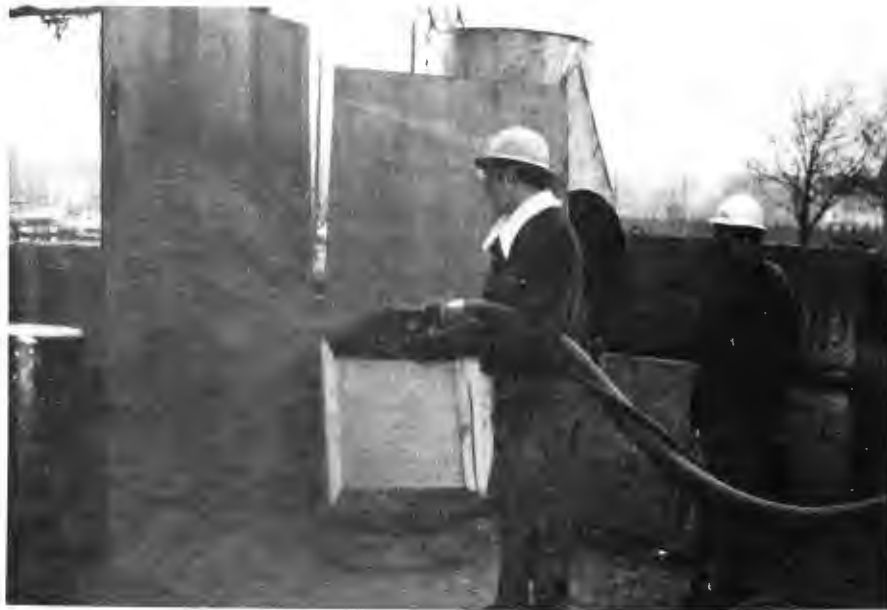
FIGURE 4.10 WARM-UP SHOOTING AGAINST PLYWOOD WALL
