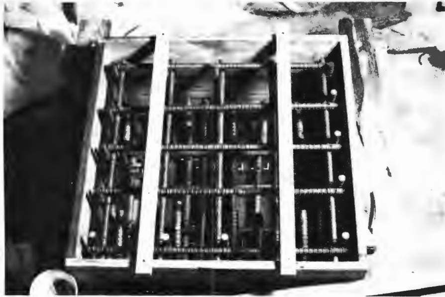
FIGURE 2.8 FORM AND REINFORCEMENT FOR THE MOVABLE BLOCKS
