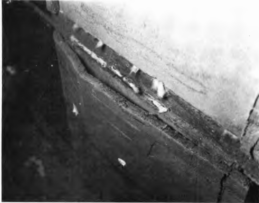
FIGURE 3.10 TOP VIEW OF MORTAR CRACKING PATTERN IN TEST NO. 17
