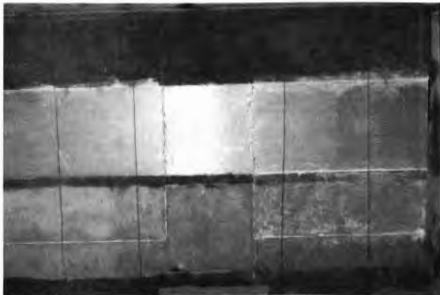
FIGURE 4.2 CLOSE-UP SHOWING VERTICAL SCREED WIRES AND TAPED SURFACE
