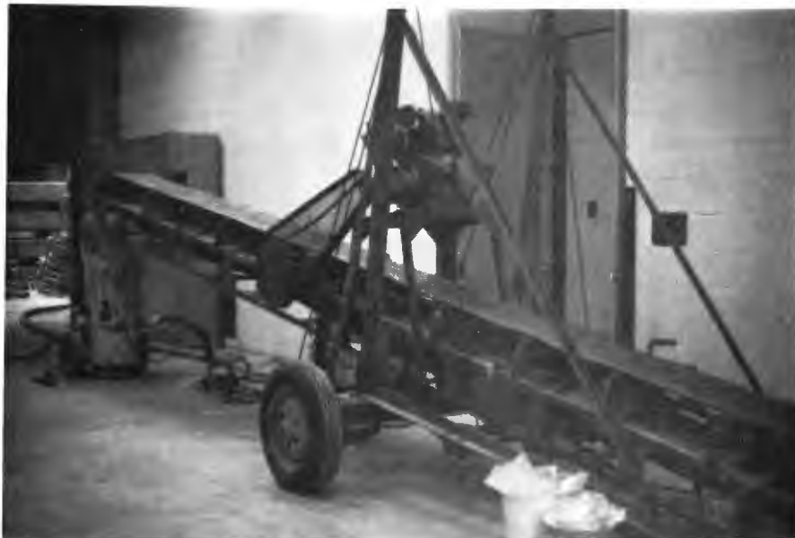
FIGURE 4.8 CLOSE-UP VIEW OF BELT CONVEYOR AND POWERED GUN
