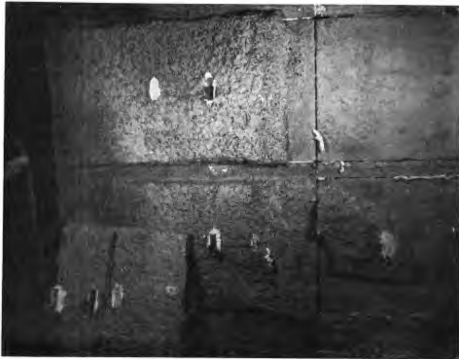
FIGURE 4.19 FRONTAL VIEW OF FAILED SURFACES IN TEST NOS. 1 AND 2
