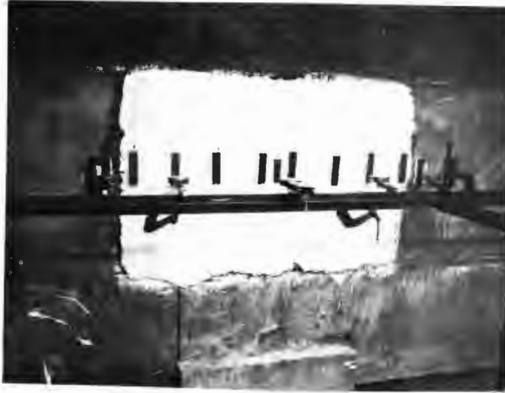
FIGURE 3.6 FRONTAL VIEW OF FAILED MORTAR LAYER WITH NO CRACKS AT THE MOVABLE-FIXED BLOCK CONTACT
