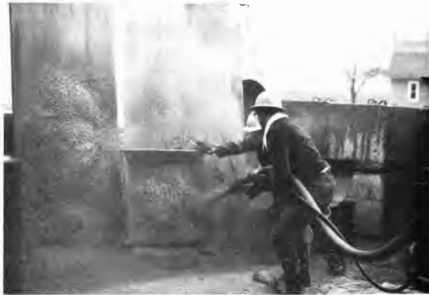
FIGURE 4.11 STRENGTH-SPECIMENS PANEL BEING FILLED UP
