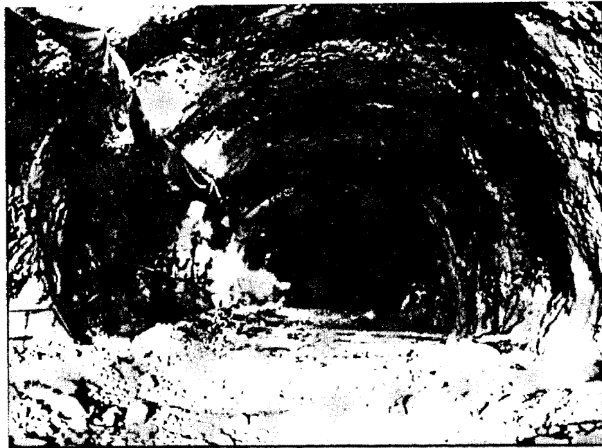
Example of tunnel excavated by full-section method
