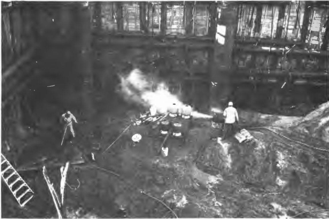
Figure 10. Small grouting job in cut-and-cover construction.
