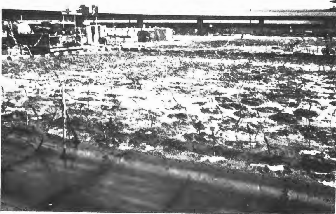
Figure 16. Grouting tubes in place for grout injection.
