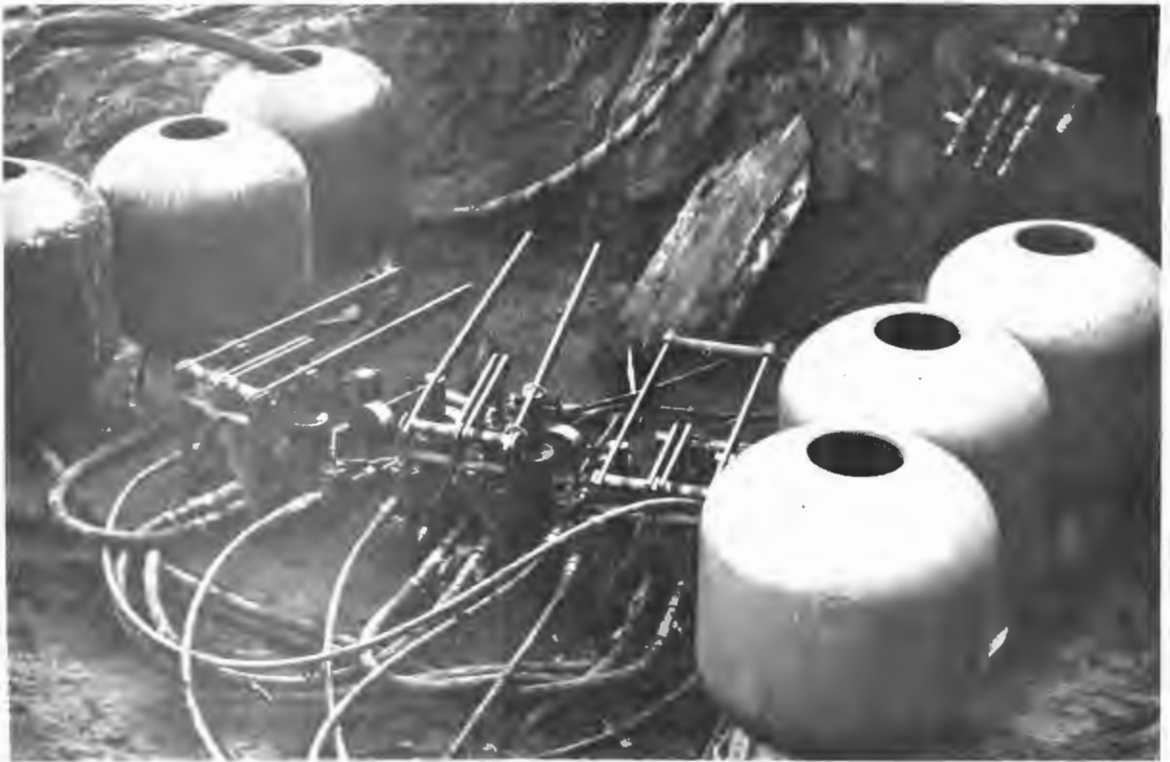
Figure 9. Dual piston type grouting pumps and mixing tanks.
