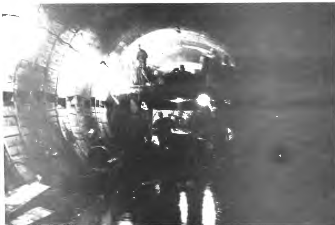
Figure C-10. Typical excavation under gouted area.
