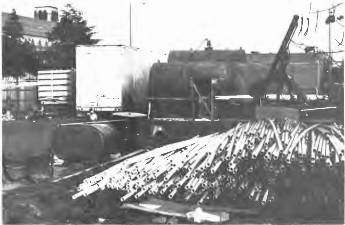
Figure 12. Large grouting job site and equipment.
