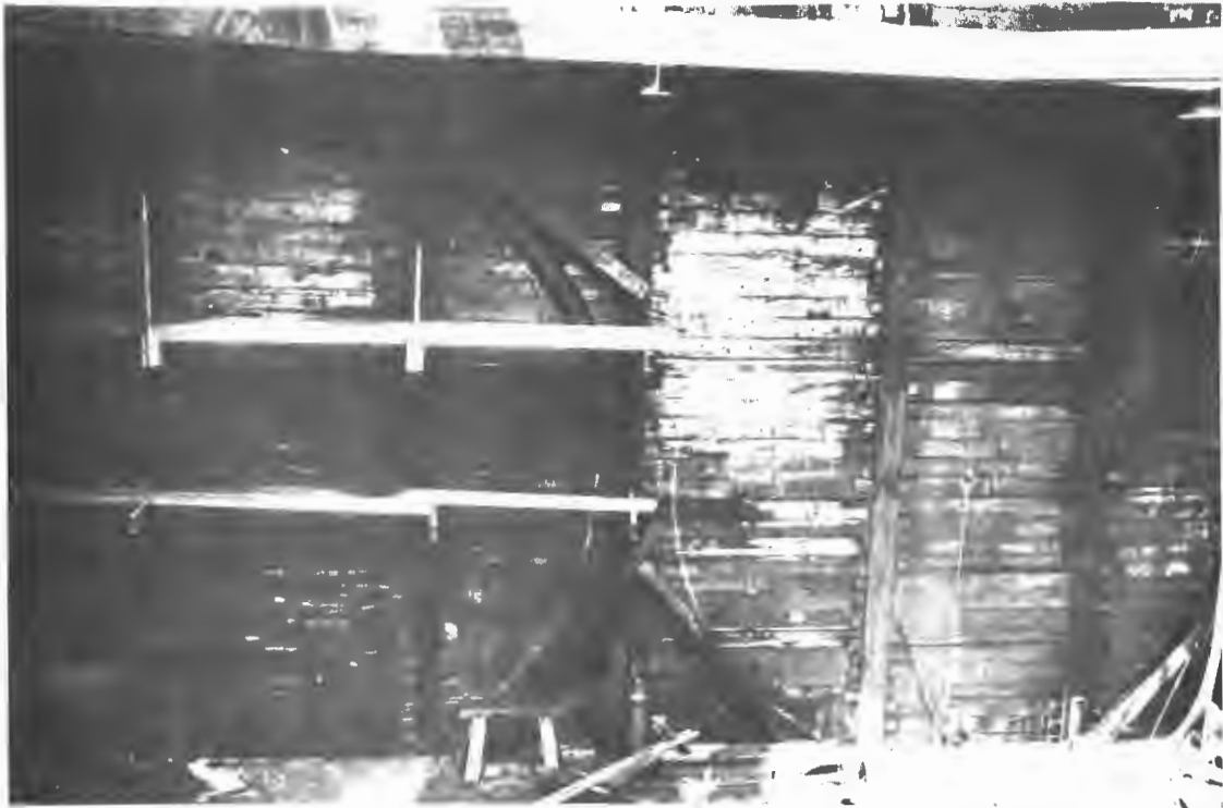
Figure C-20. Tunnel portal opening.
