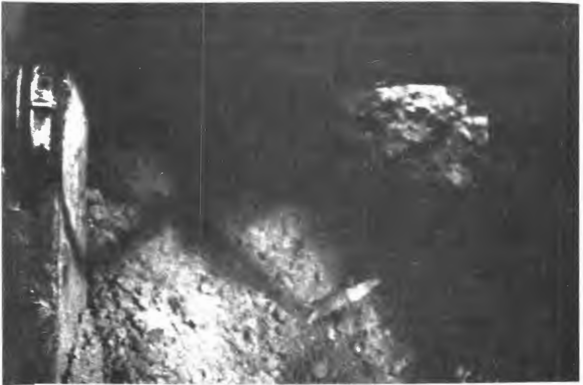
Figure C-21. Grouted soil at tunnel face.
