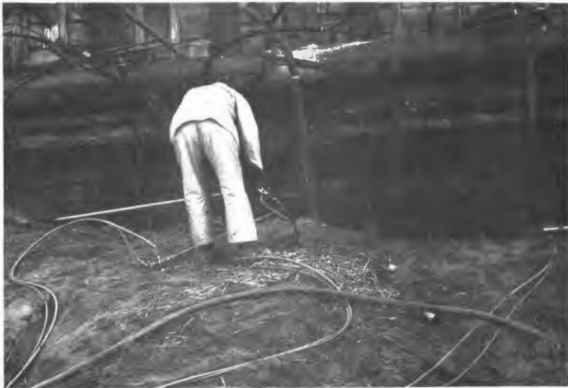
Figure 11. Grouting to consolidate sand behind wood lagging.
