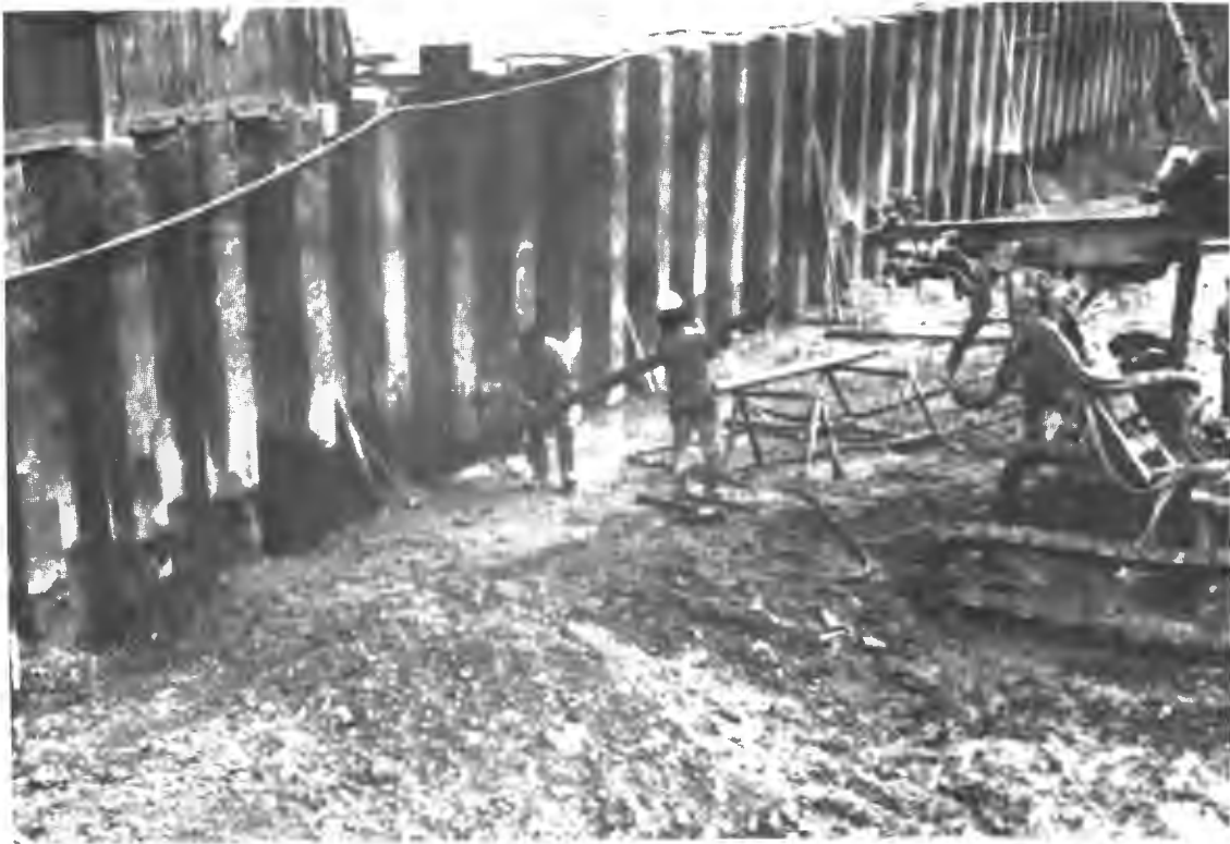
Figure 29. Placing tieback in sheet steel wall.
