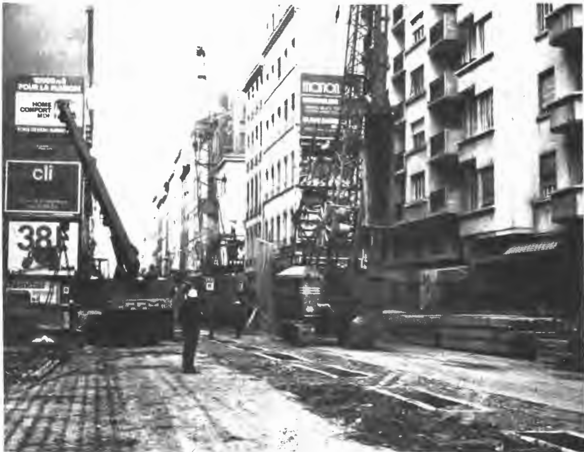
Figure 74. Clamshell bucket crane used for slurry trench construction
