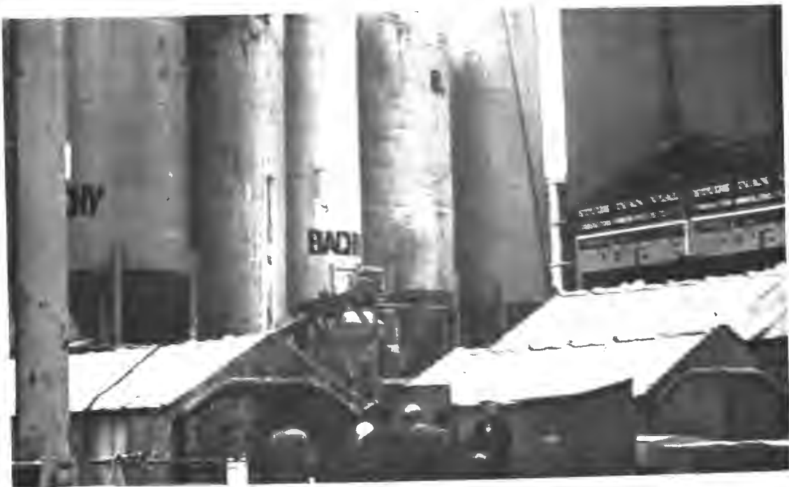
Figure 45. Batch plant for large grouting operation.
