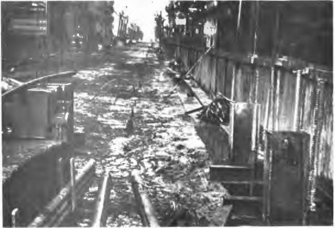
Figure 8. Slurry trench, diaphragm wall and grouting on French job.
