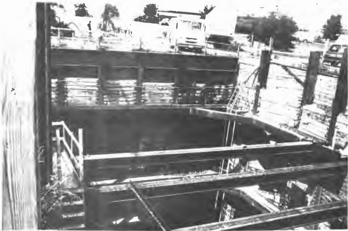
Figure C-19. Grouting toward portal opening
