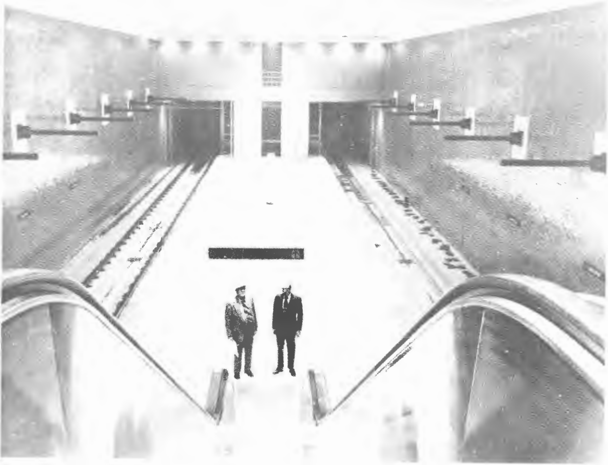
Figure 11. Van Ness Station Under Construction
