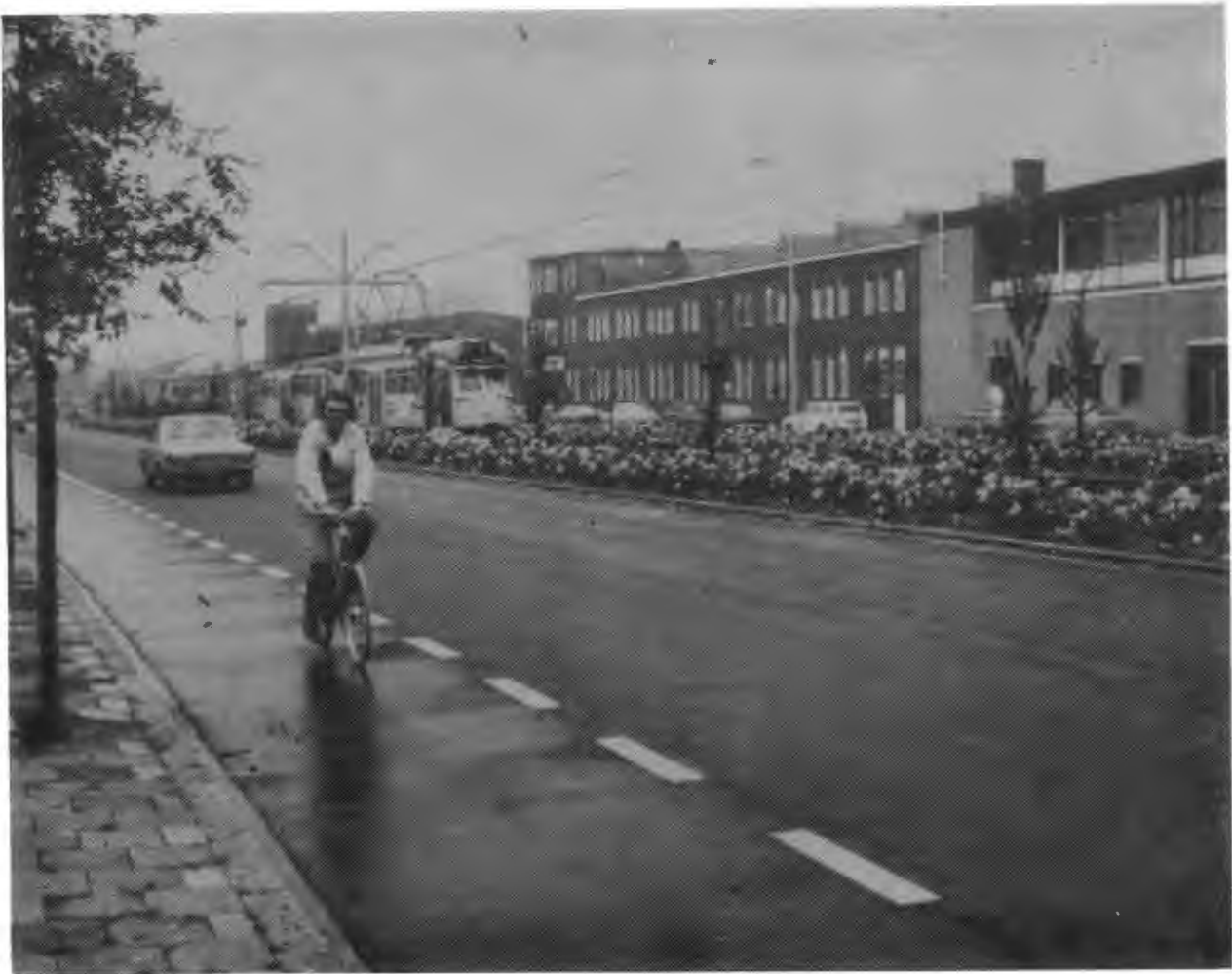
Figure 76. Catenary Power Distribution at The Hague
