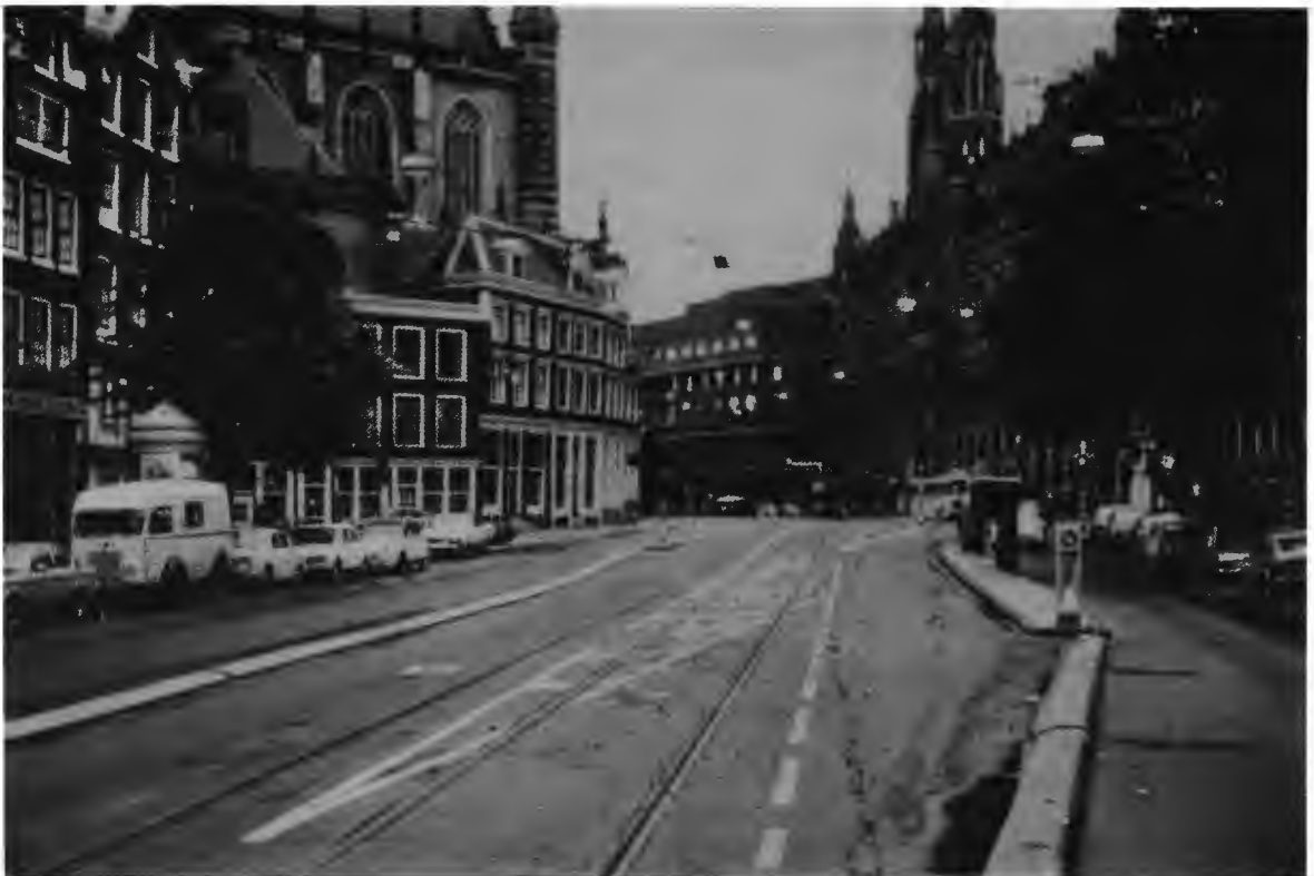
Figure 4. Off Line Bus Stop on Amsterdam Transit Lane
