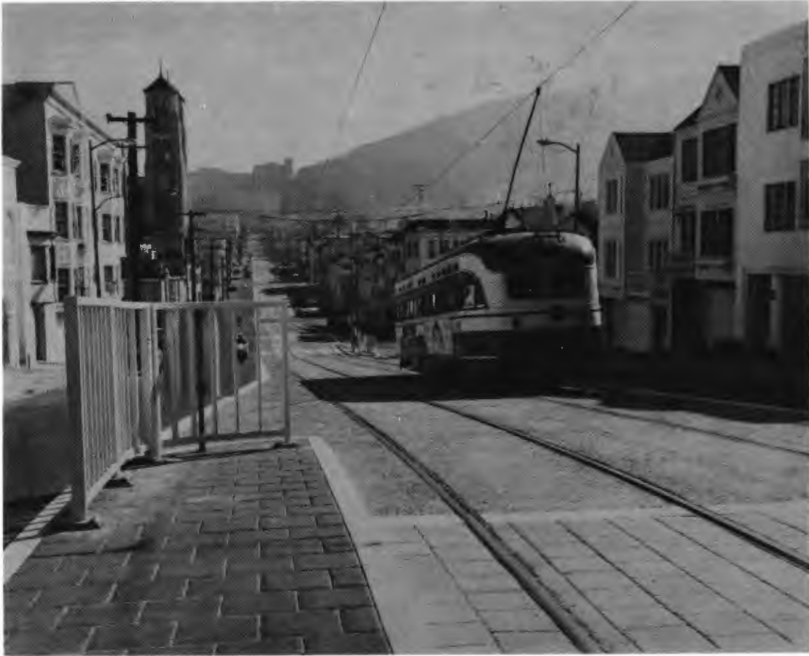
Figure 26. New Median Trackage – Judah Street
