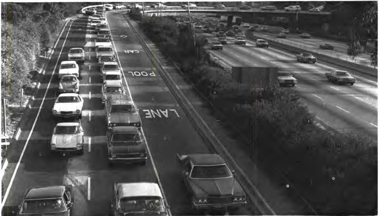
Figure 4. Los Feliz Boulevard at Golden State Freeway (I-5). This is the only bypass ramp that utilizes two metered lanes in addition to the bypass lane.
