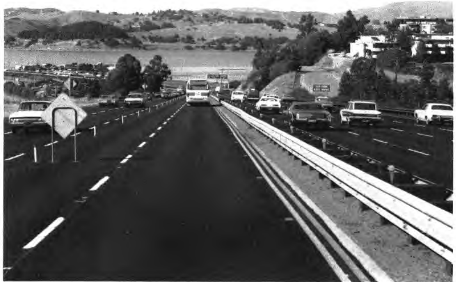
Northbound p.m. contra-flow lane on Waldo Grade. Note the closed buffer lane on the left.
