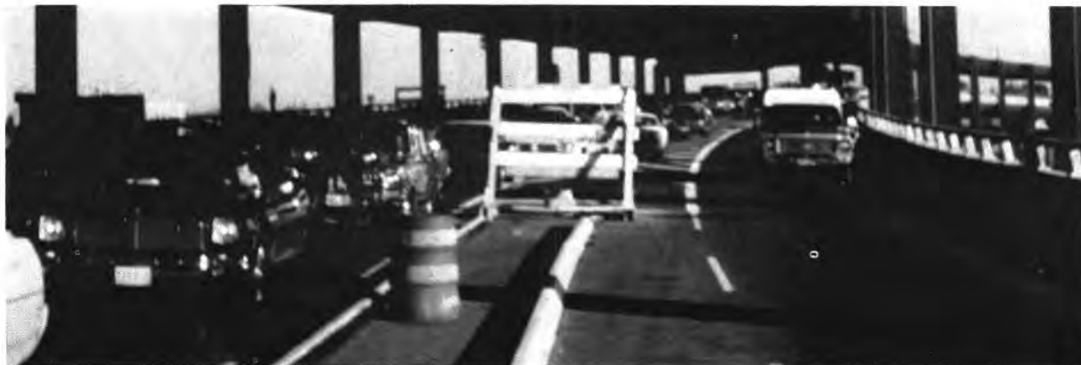
Carpool entering priority lane. Bituminous curb in adjacent lane separates buses and carpools from the regular traffic lanes.
