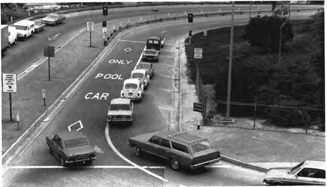
Figure 2. Hawthorne Boulevard at San Diego Freeway (I-405) in Lawndale. This is the only bypass lane now being metered.
