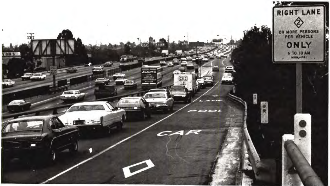
Figure 5. Manning Avenue at Santa Monica Freeway (I-10). This is one of the five right lane bypasses. The compliance rate on this ramp is the highest of all bypasses.
