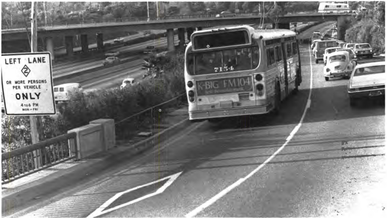
Figure 3. Los Feliz Boulevard at Golden State Freeway (I-5) in Los Angeles. This bypass lane is used by twelve buses as well as 500 to 600 car pools daily between 4:00 and 6:00 p.m.
