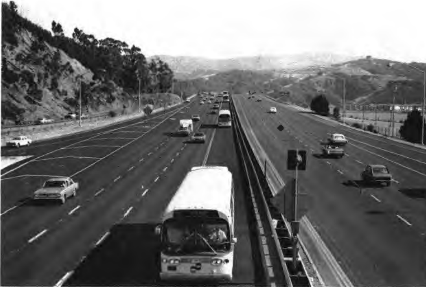
Exclusive p.m. concurrent flow bus lane northbound. Note that southbound left lane has been closed before the contra-flow lane is encountered.
