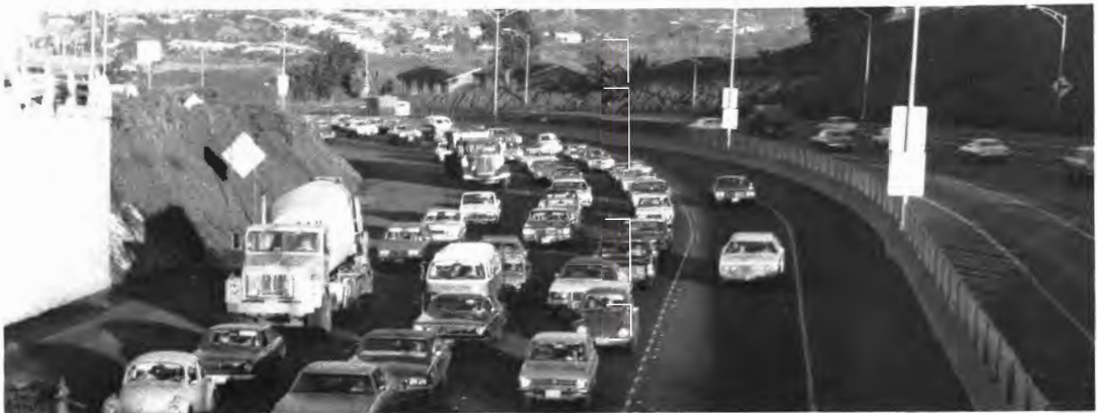
Reserved bus and carpool lane along the Moanalua Freeway
